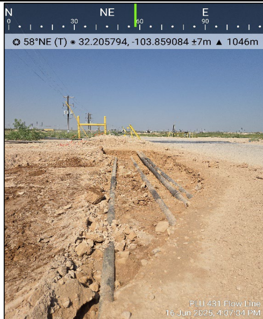
Photograph: 3 Date: 6/16/2025 Description: Excavation activities; near FS01 View: Northeast
