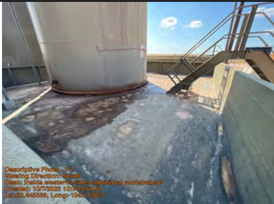
Inside western side additional containment
