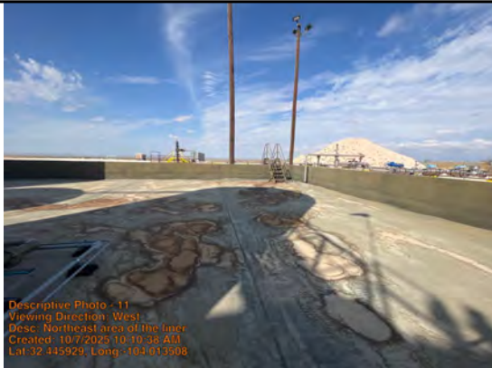
Northeast area of the liner
