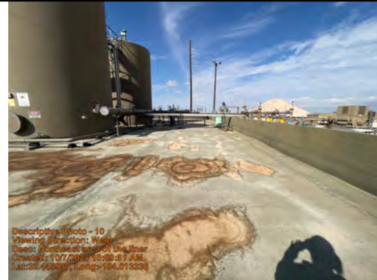
Northeast area of the liner
