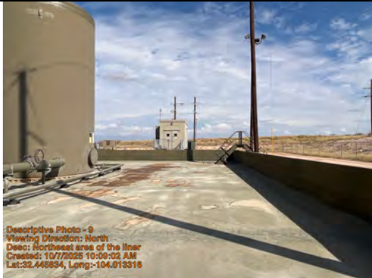
Northeast area of the liner
