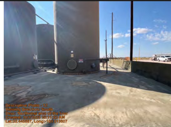
Northwest area of the liner
