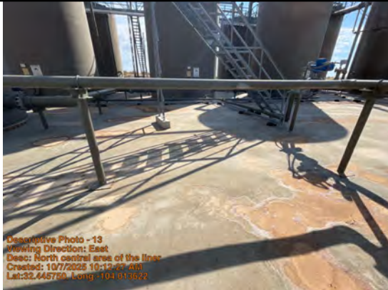
North central area of the liner
