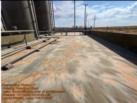
Southwestern area of containment
