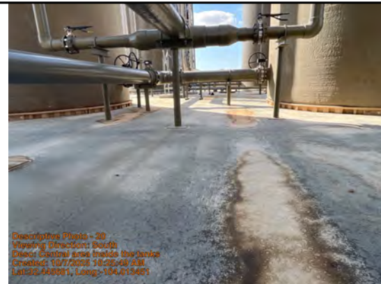
Central area inside the tanks
