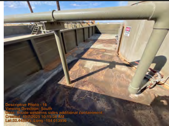
Inside western side additional containment
