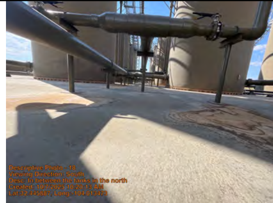
In between the tanks in the north
