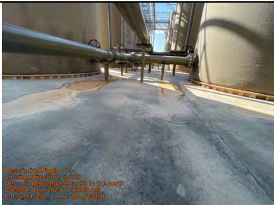
In between the tanks in the north
