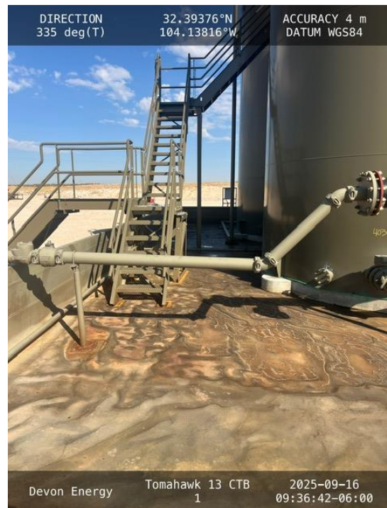
Photo 8 View of containment towards Northwest.
