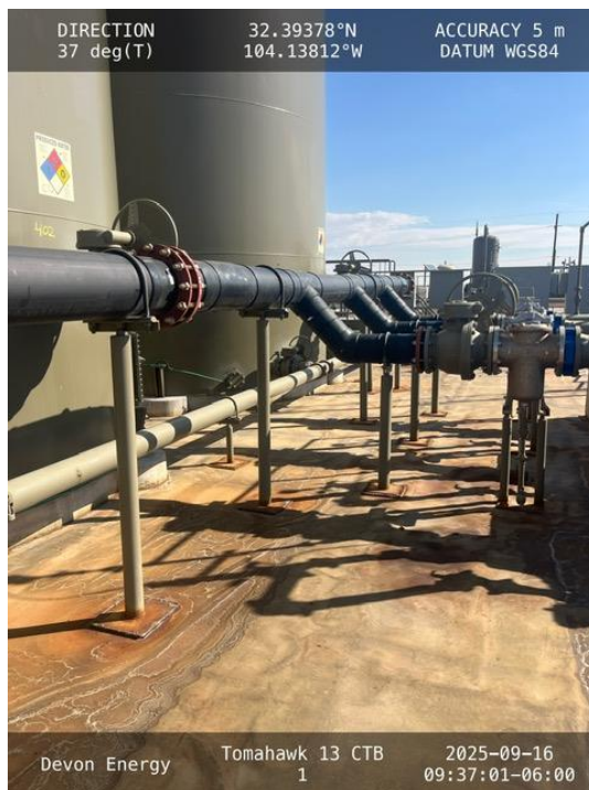
Photo 9 View of containment towards Northeast.
