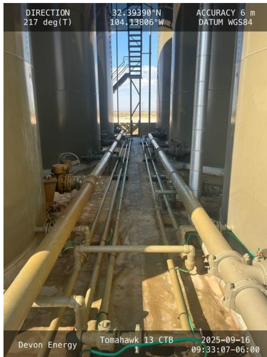
Photo 5 View of containment towards South.
