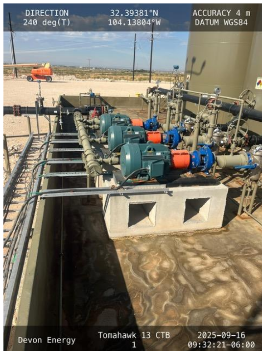
Photo 1 View of containment towards Southwest.
