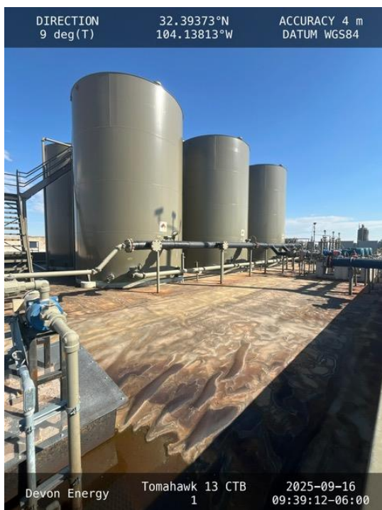
Photo 13 View of containment towards North.
