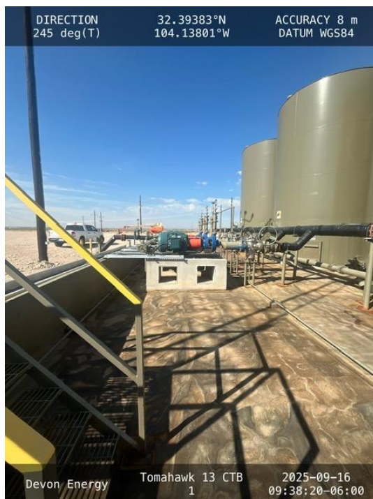
Photo 11 View of containment towards Southwest
