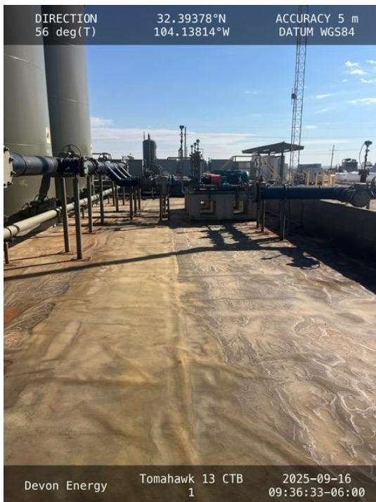
Photo 7 View of containment towards East
