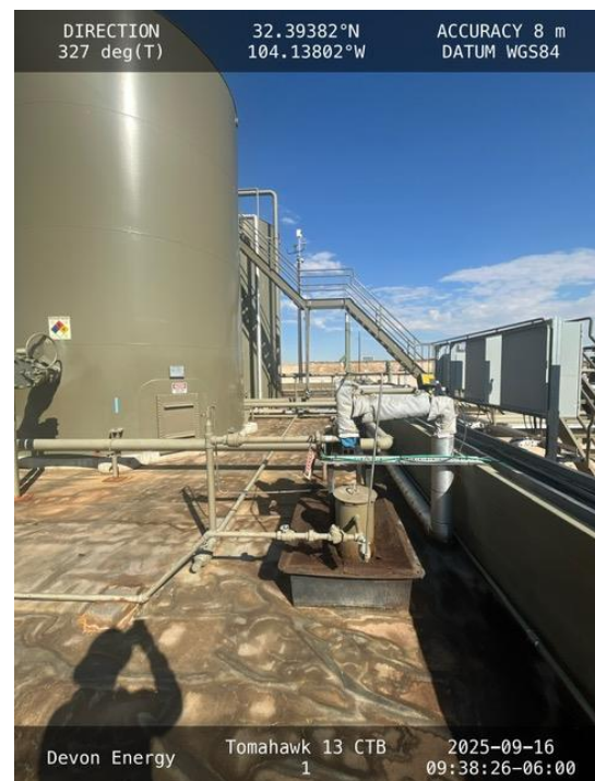
Photo 12 View of containment towards Northwest.
