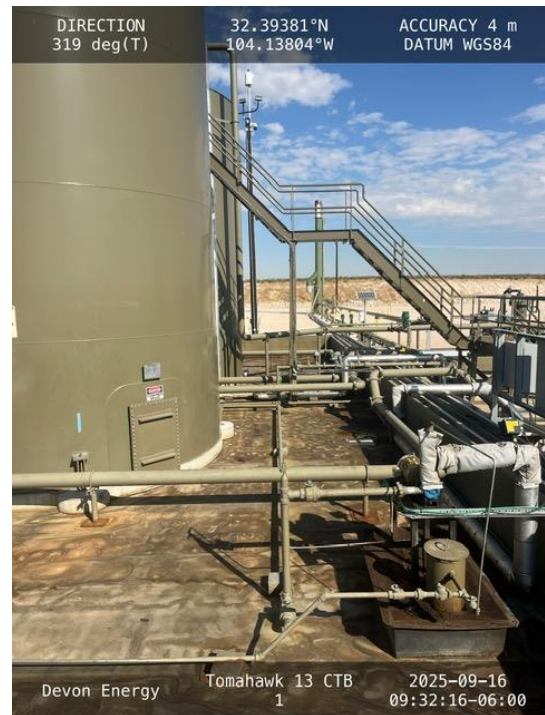
Photo 2 View of containment towards northwest.
