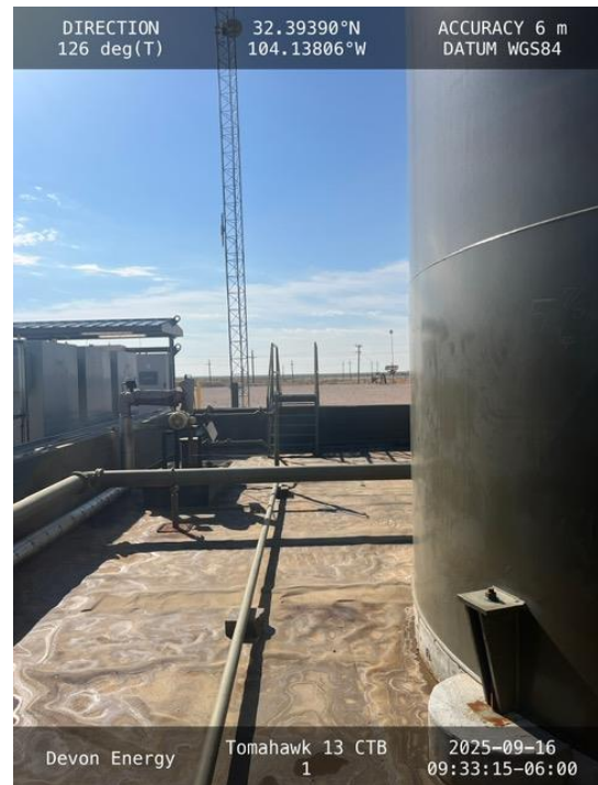
Photo 6 View of Southeast corner of containment.
