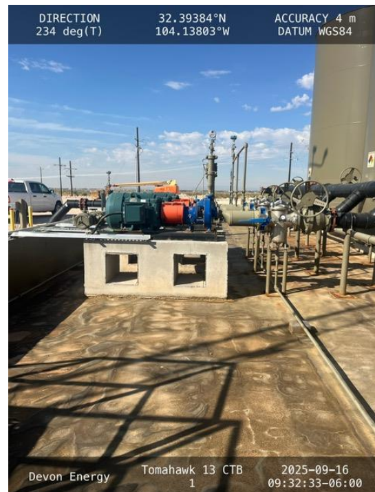
Photo 2 View of containment towards Southwest.
