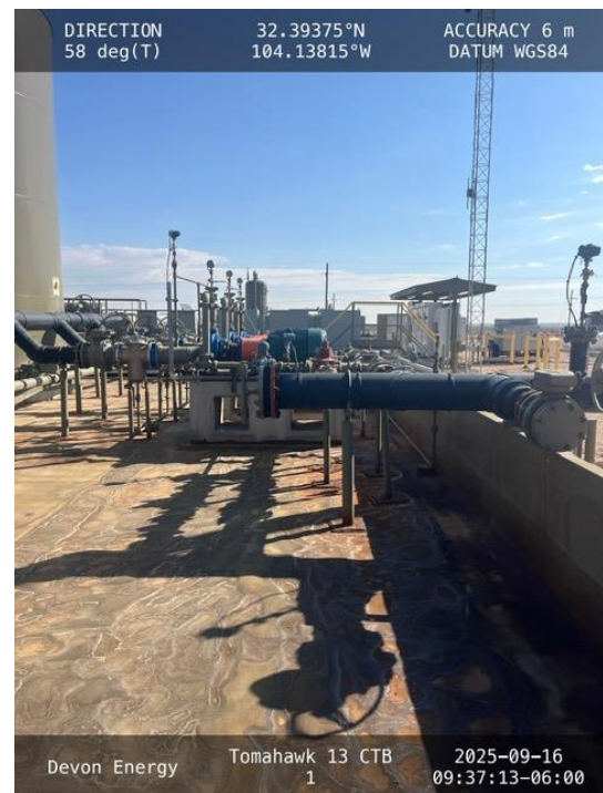
Photo 10 View of containment towards East.
