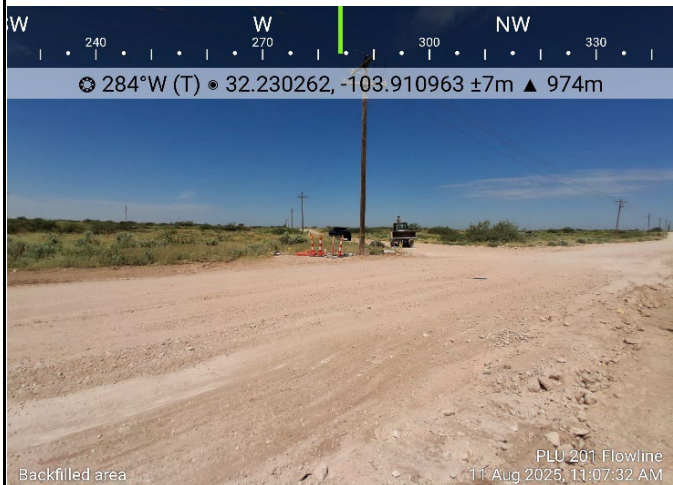
Photograph: 4 Date: 8/11/2025 Description: Backfilling activities View: West
