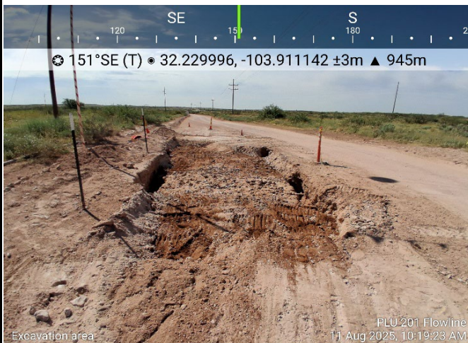
Photograph: 3 Date: 8/11/2025 Description: Excavation activities View: Southeast
