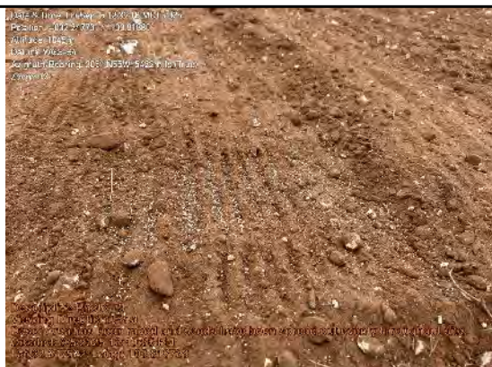
Area has been raked and seeds have been spread out evenly throughout site. Close up view of seeds
