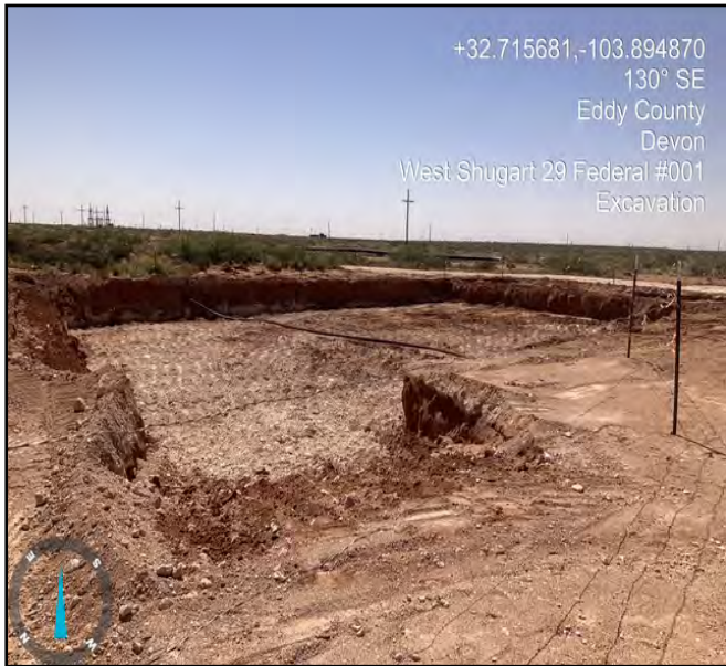
Photograph taken during the excavation process facing southeast.
