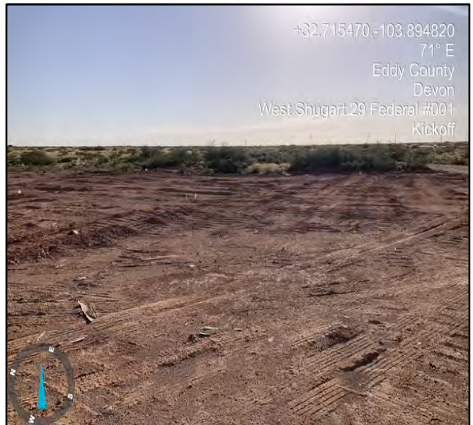
Photograph taken pre- excavation process, facing east.
