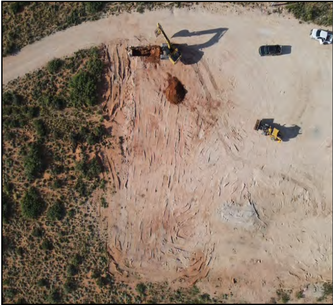
Aerial kickoff photos.
