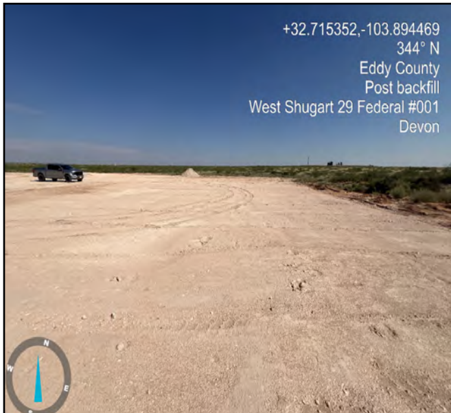
Photograph taken post excavation , facing north.
