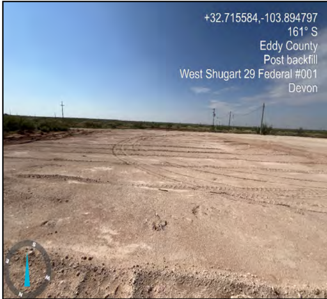
Photograph taken post excavation , facing south.
