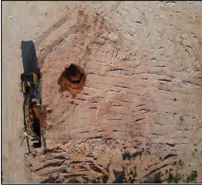
Aerial kickoff photos.
