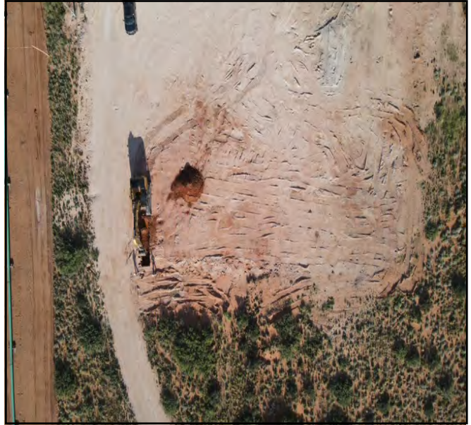
Aerial kickoff photos.
