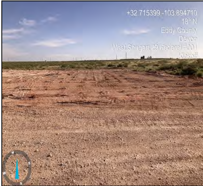
Photograph taken pre- excavation process, facing north.
