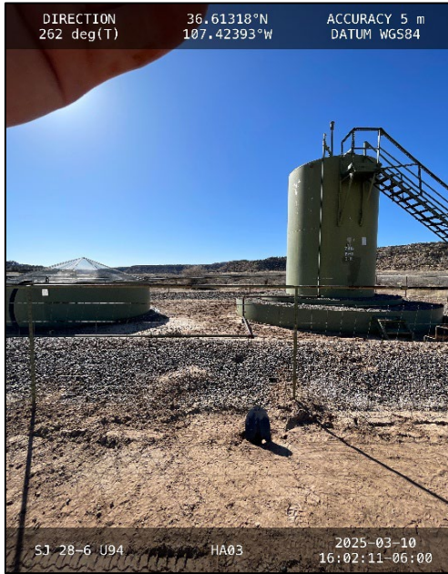
Photograph: 1 Date: 3/10/2025 Description: HA03, outside berm, near HA02 View: West
