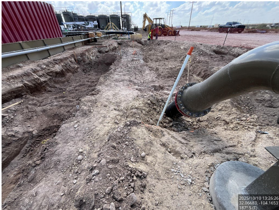
Excavated area, viewing south.
