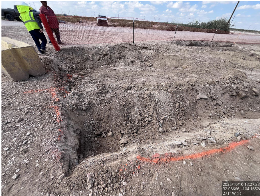
Excavated area, viewing west.
