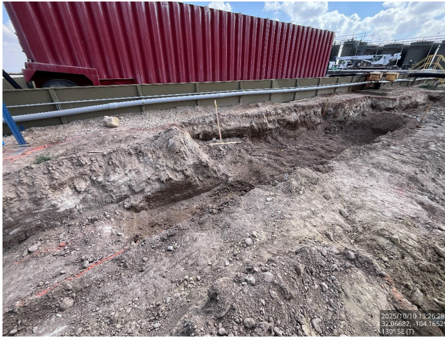
Excavated area, viewing southeast.
