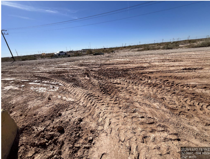
Backfilled area, viewing west.
