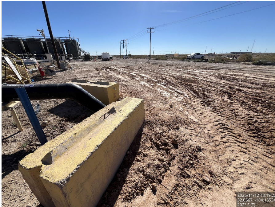
Backfilled area, viewing south.
