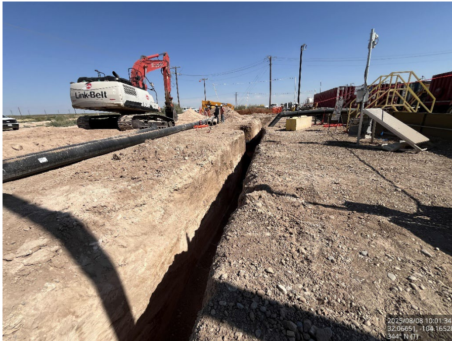
Trench through remediation area, viewing north.
