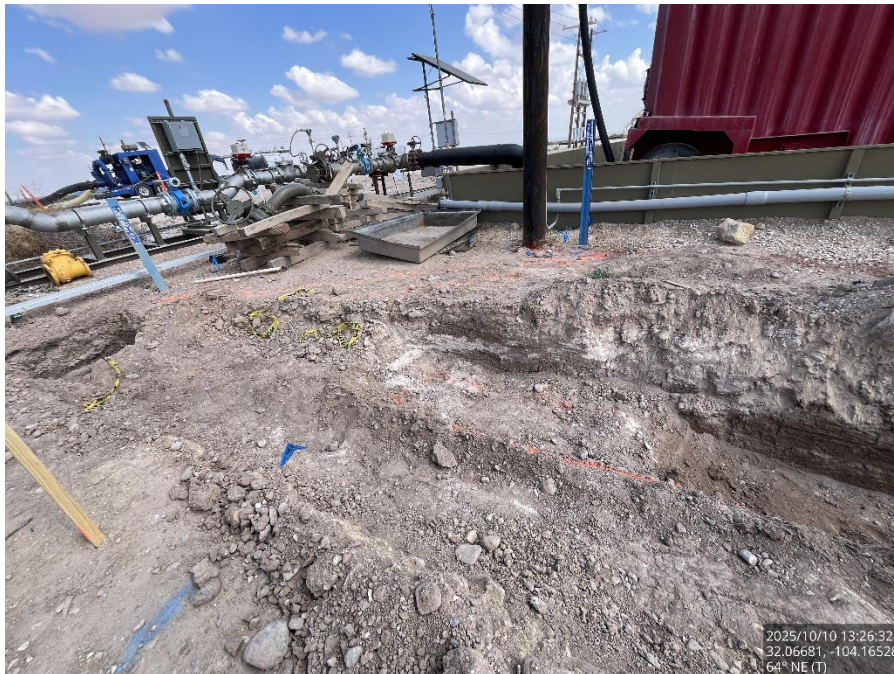
Excavated area, viewing northeast.
