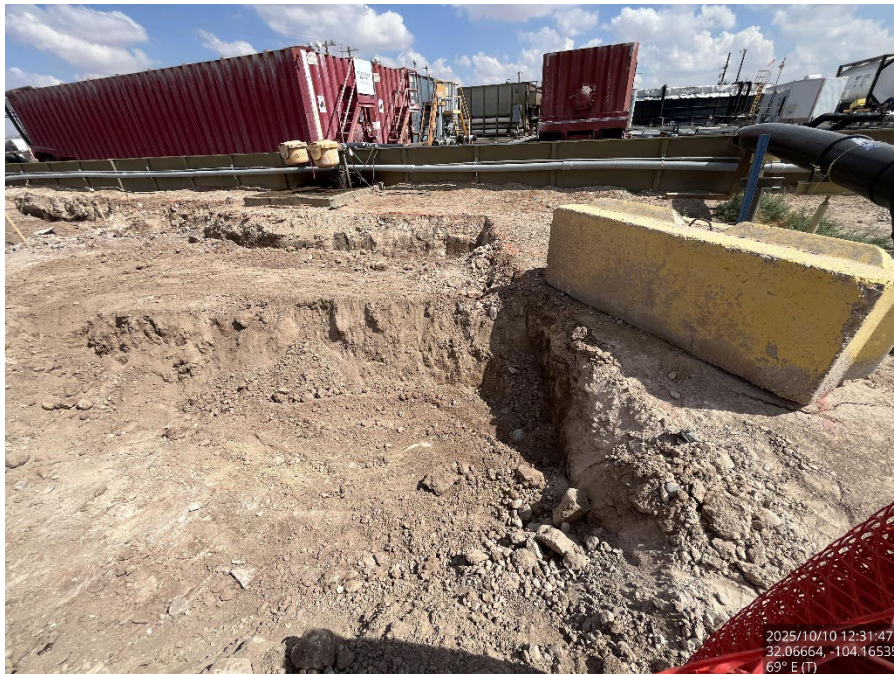
Excavated area, viewing east.
