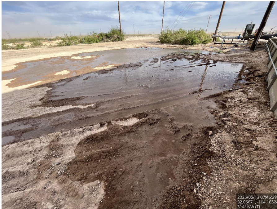
Spill area, viewing northwest.
