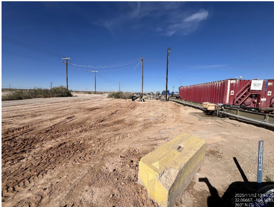
Backfilled area, viewing north.
