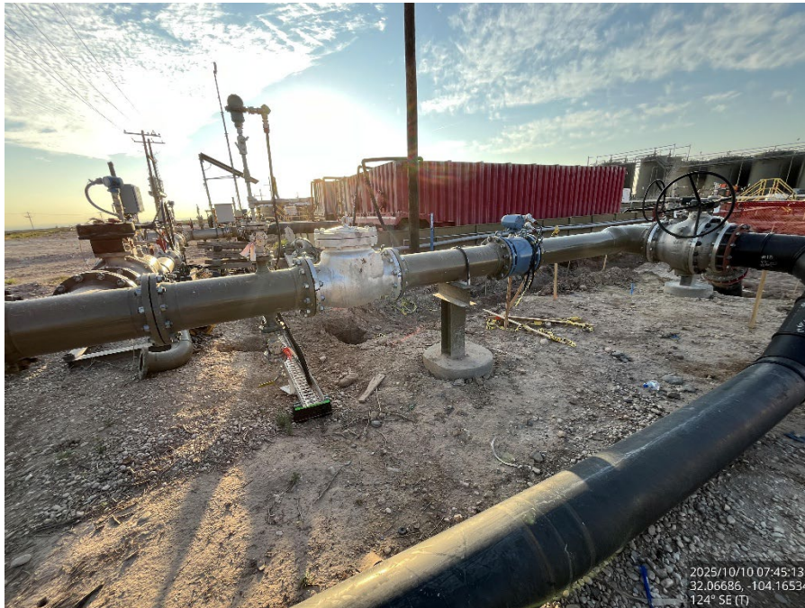
Excavated area, viewing southeast.
