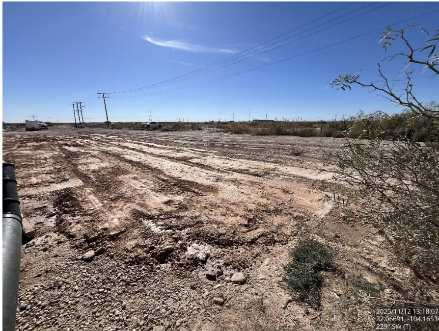
Backfilled area, viewing southwest.
