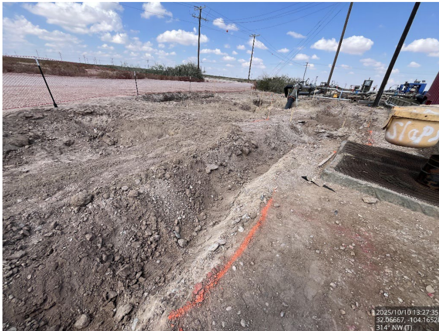
Excavated area, viewing northwest.
