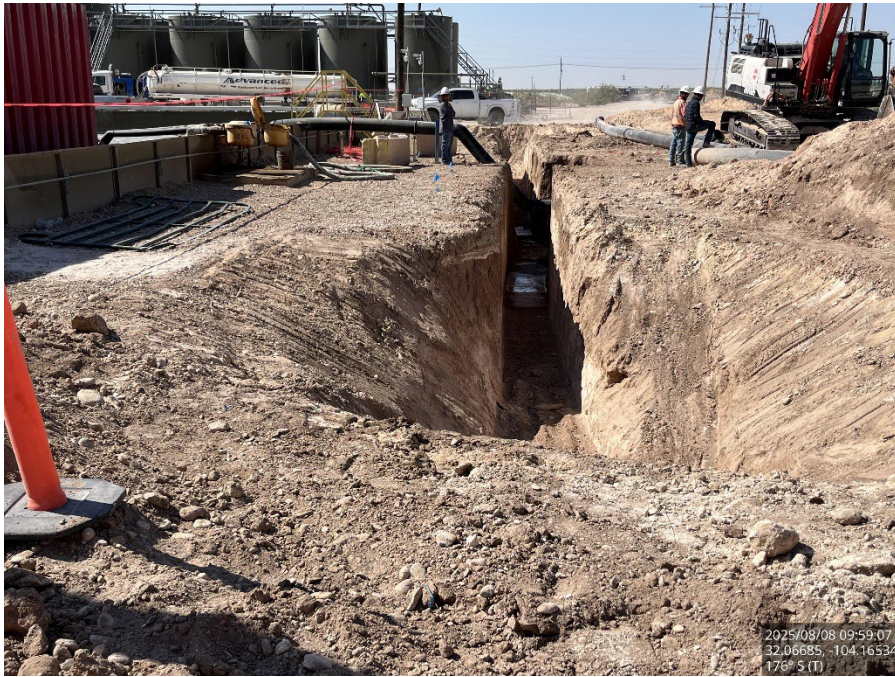
Trench through remediation area, viewing south.
