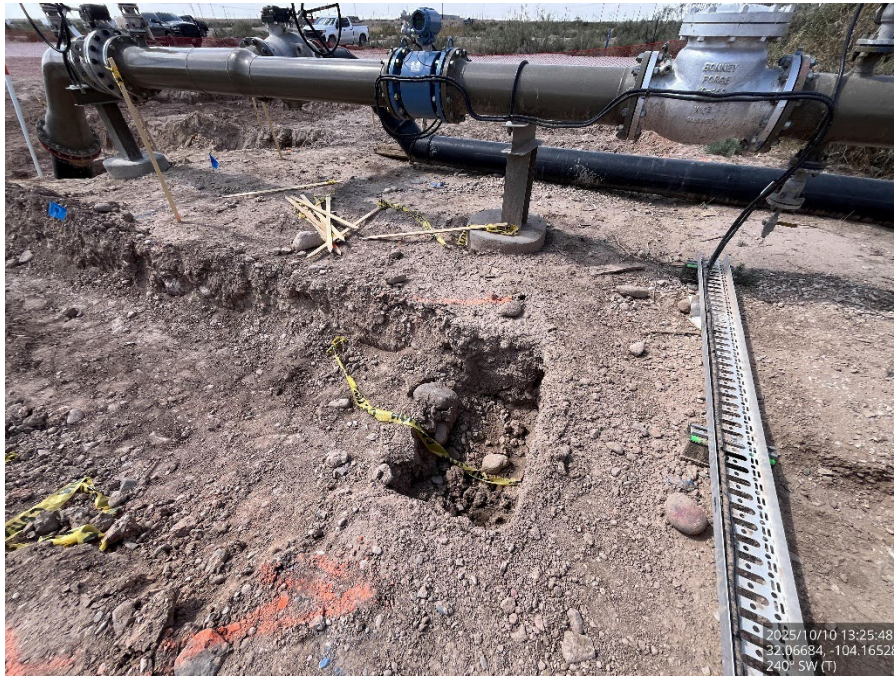
Excavated area, viewing southwest.
