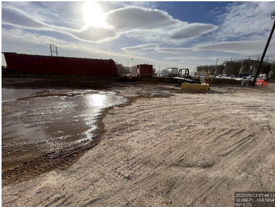
Spill area, viewing east.
