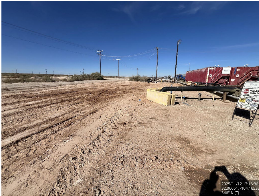
Backfilled area, viewing north.
