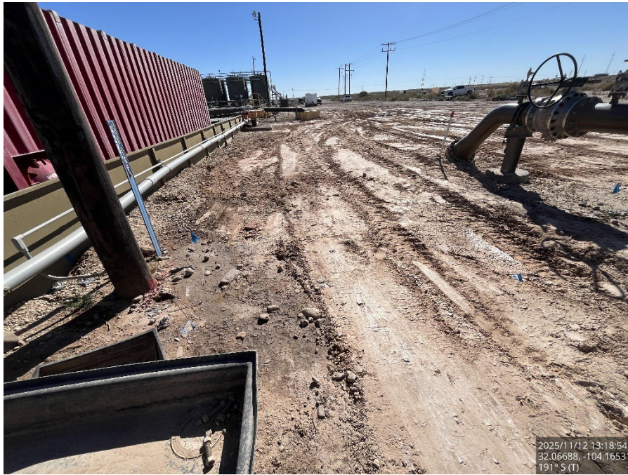
Backfilled area, viewing south.
