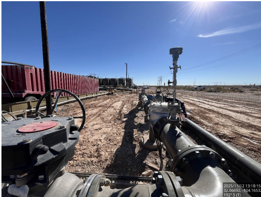
Backfilled area, viewing south.
