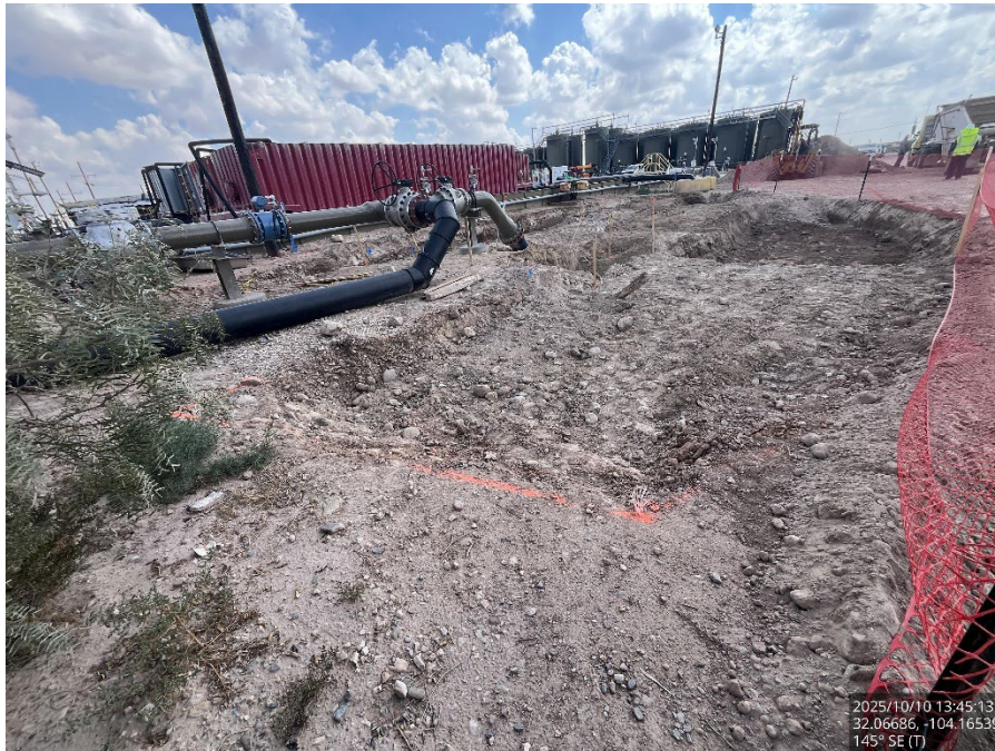
Excavated area, viewing southeast.
