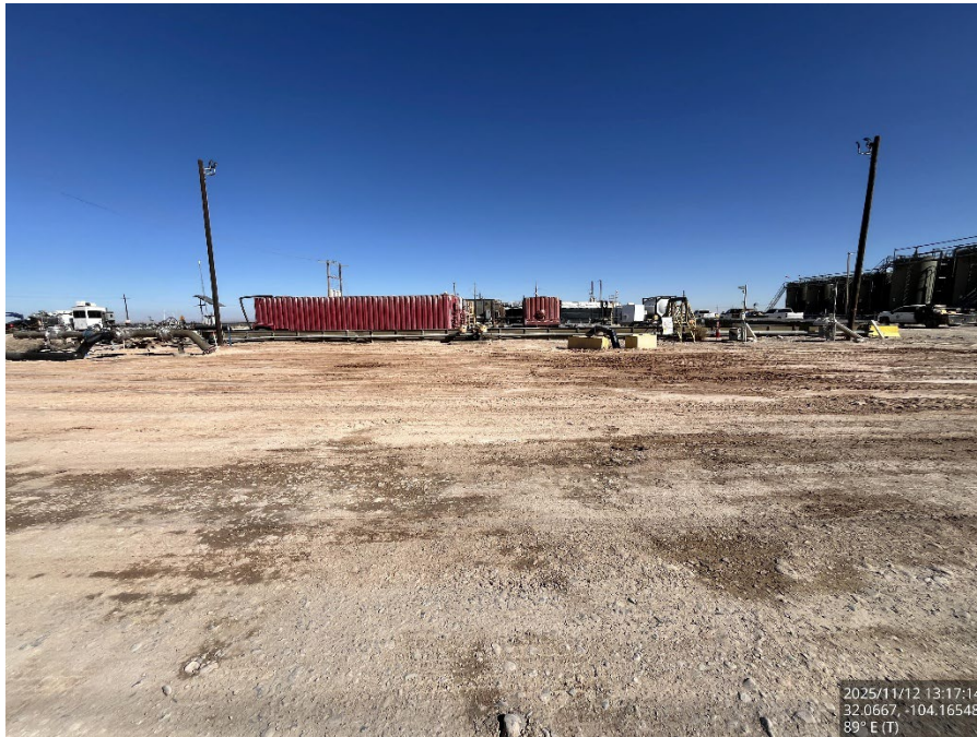
Backfilled area, viewing east.
