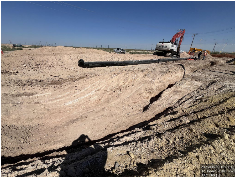
Trench through remediation area, viewing northwest.
