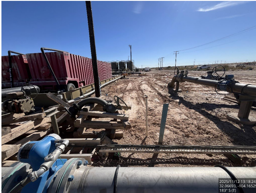
Backfilled area, viewing south.
