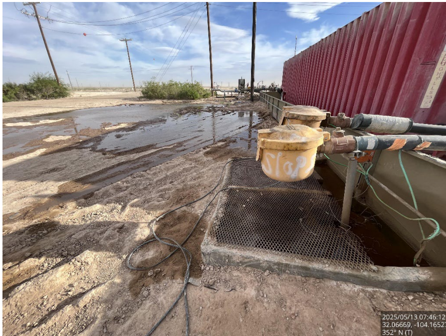
Spill area, viewing north.
