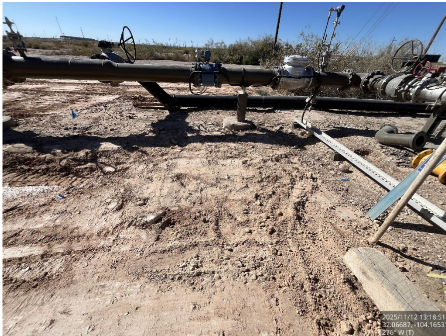
Backfilled area, viewing west.
