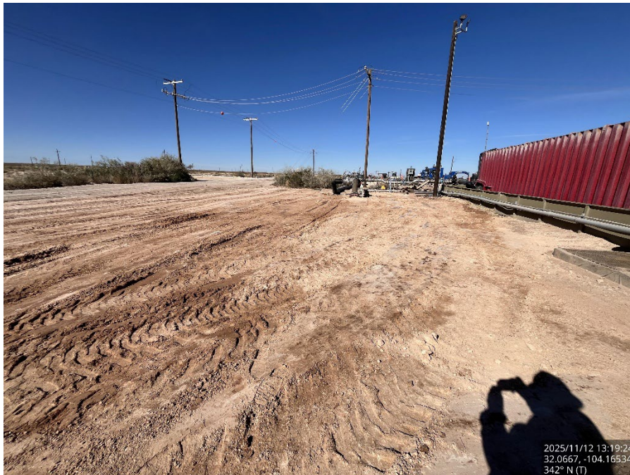
Backfilled area, viewing north.
