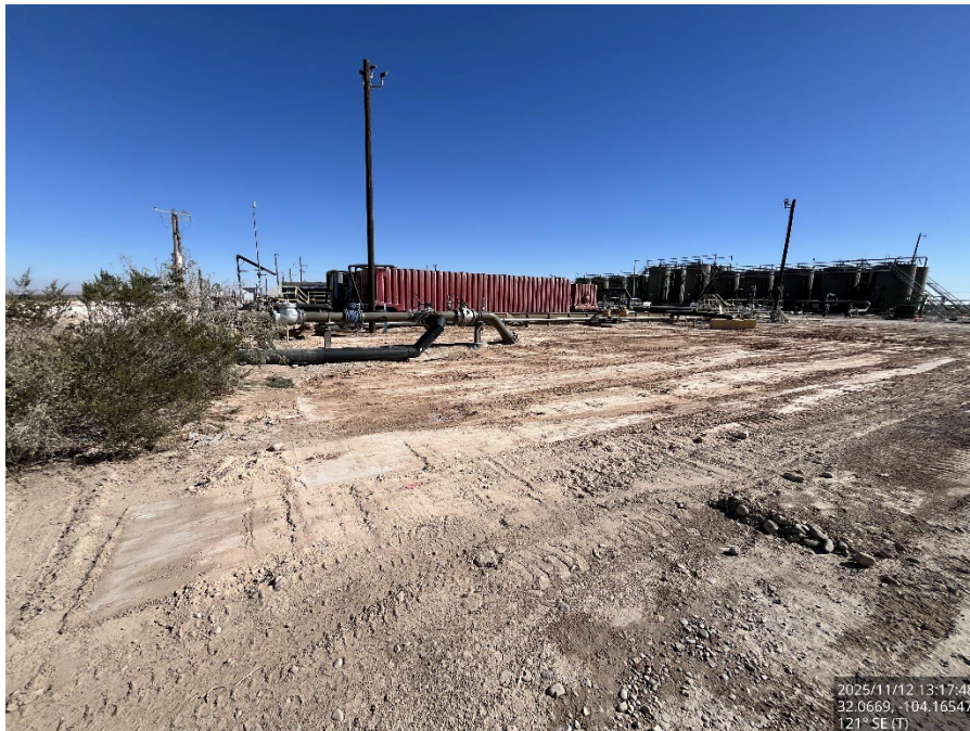
Backfilled area, viewing southeast.
