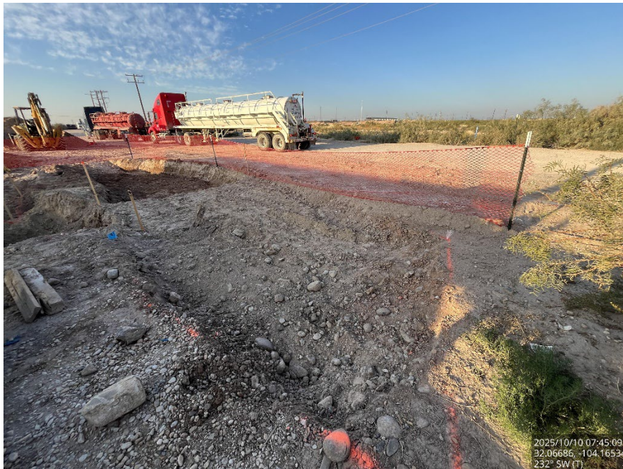
Backfilled area, viewing southwest.
