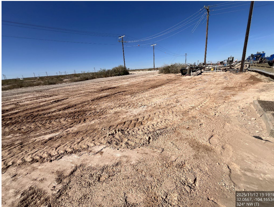
Backfilled area, viewing west.
