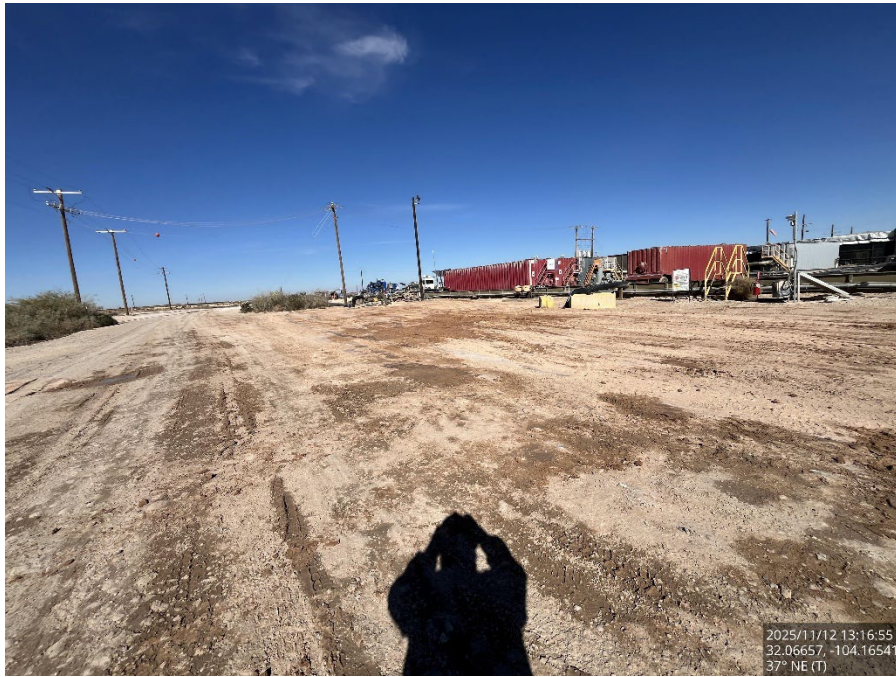
Backfilled area, viewing northeast.
