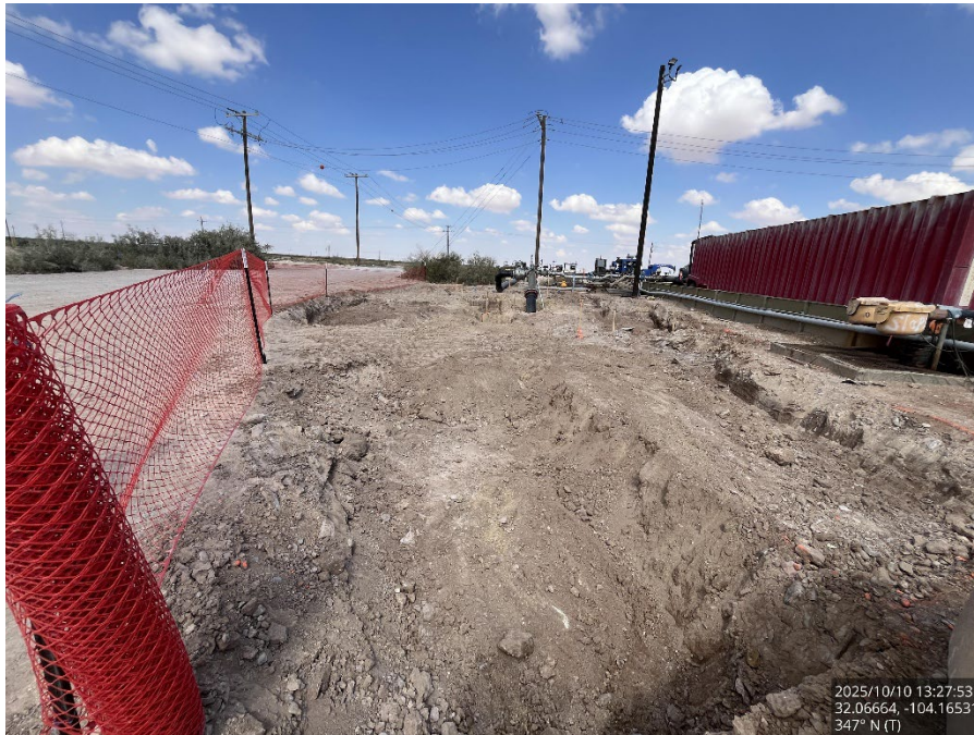
Excavated area, viewing north.
