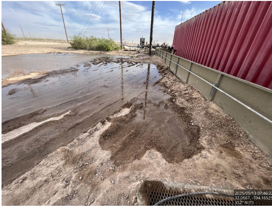
Spill area, viewing north.
