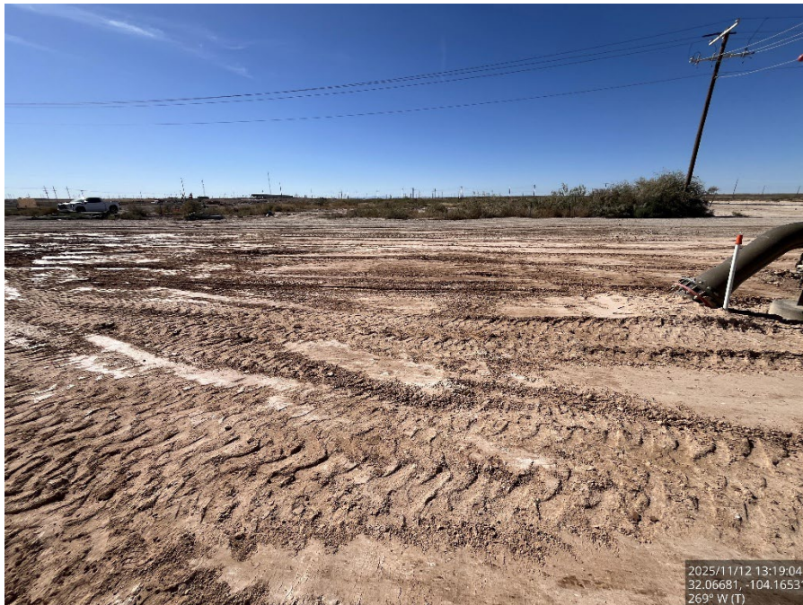
Backfilled area, viewing west.
