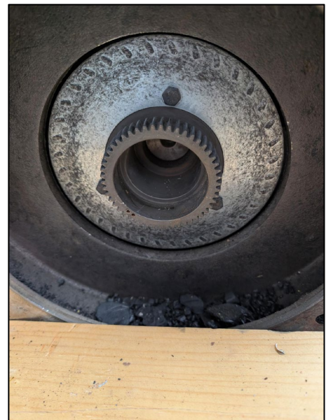
Photograph: 4 Description: Coupling removed – Blower side View: NA
