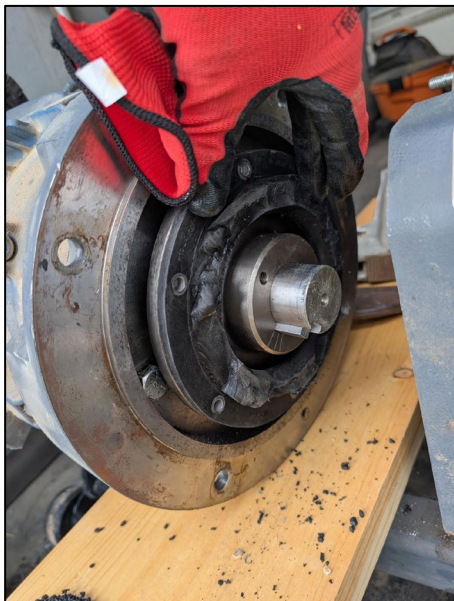
Photograph: 3 Description: Failed coupling, motor side View: NA
