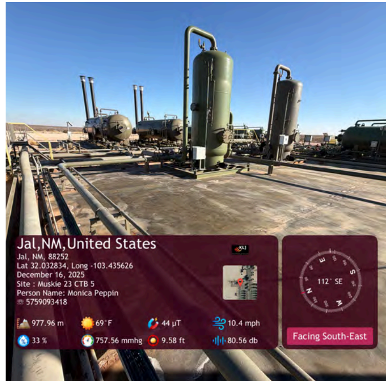
Liner in open area of separator containment.
