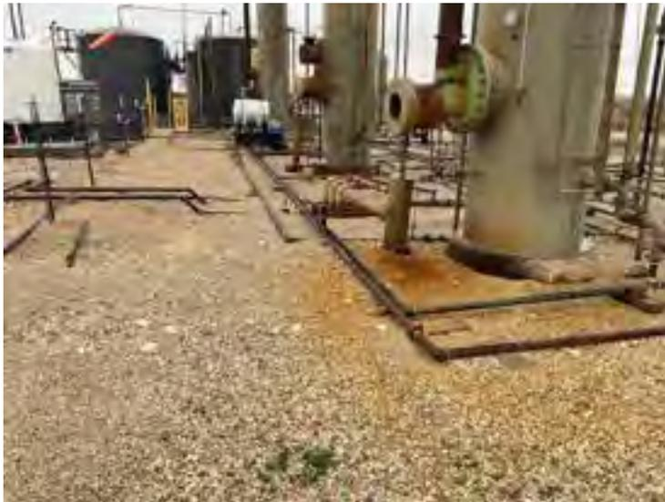
**Photograph 3:** Surficial staining between equipment.
