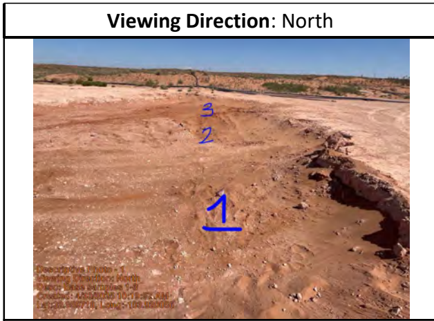
Base samples 1-3 to the east most area of the excavation
