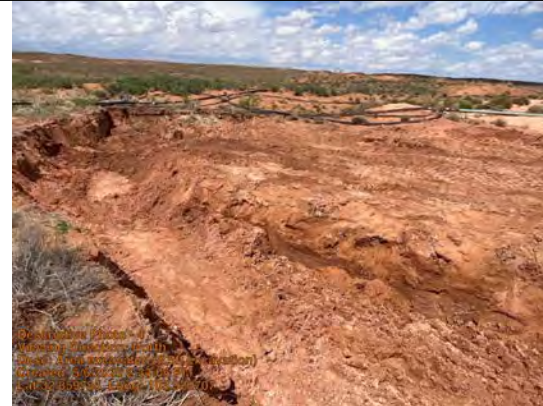
Area excavated (2.5ft excavation)
