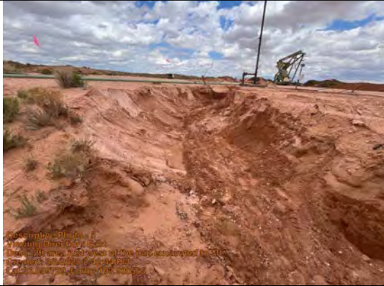
2ft area just west of the pad excavated to 3ft
