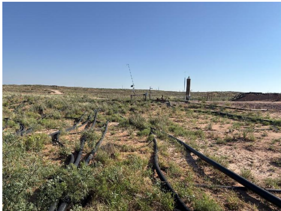
Figure 16. Oil and gas facility and infrastructure
