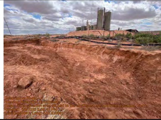
4ft excavation area off pad to the northwest area of the excavation. Field screened in compliance of criteria
