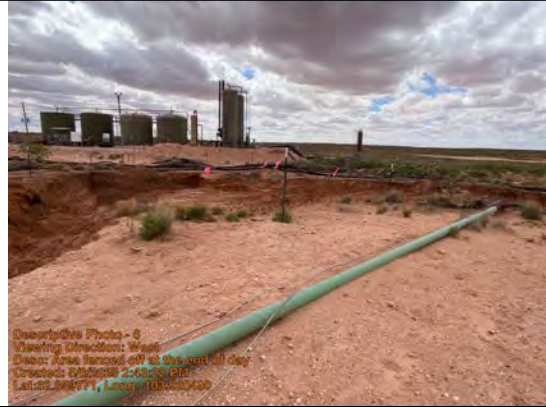
Area fenced off at the end of day
