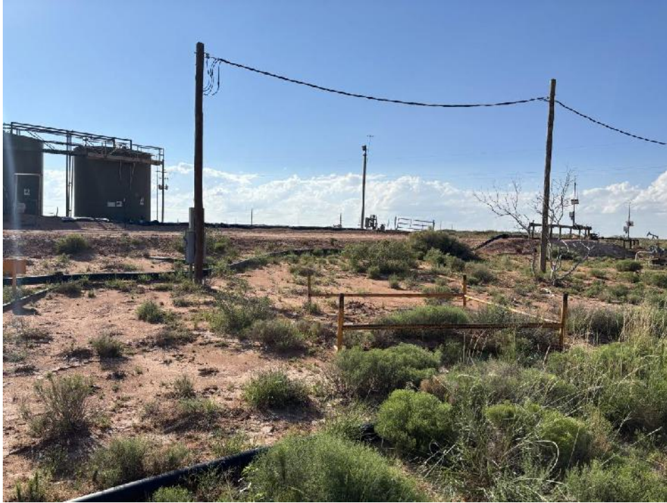
Figure 17. Pipelines, powerlines, and vegetation at site
