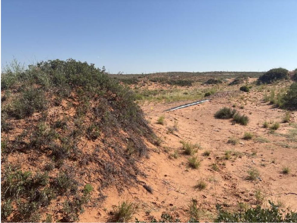
Figure 11. Sandy dune blowout with exposed pipeline
