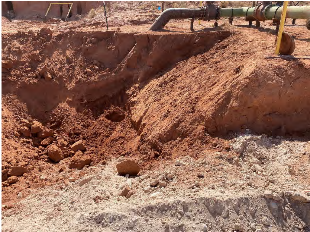
Photograph 2: View southeast of the above ground production equipment adjacent to sidewall SW08.
