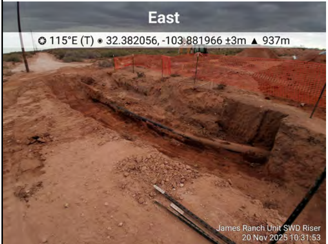
Photograph: 8 Date: 11/20/2025 Description: Excavation activities near FS07 View: East
