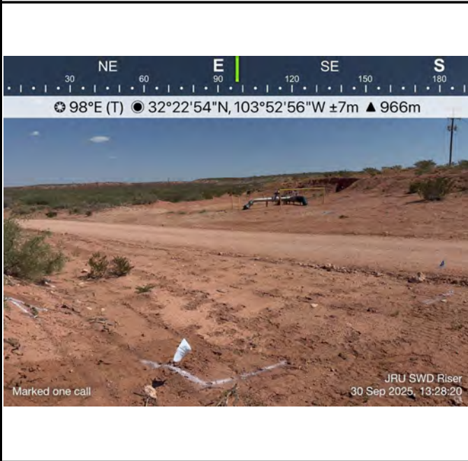
Photograph: 1 Date: 9/30/2025 Description: Access road, SWD riser. View: East
