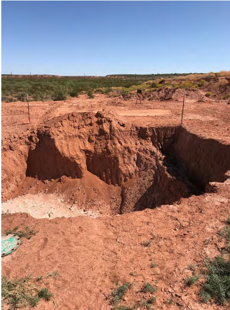
Northern view of final excavation extent during confirmation soil sampling activities.
