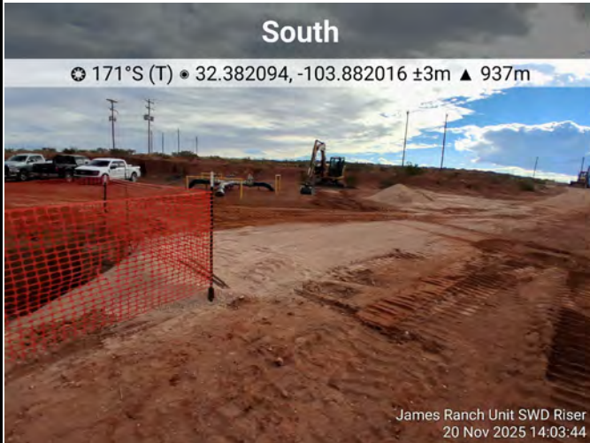
Photograph: 7 Date: 11/20/2025 Description: Backfill near FS06 View: South
