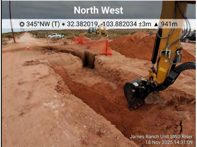
Photograph: 6 Date: 11/18/2025 Description: Excavation area near FS06 View: East
