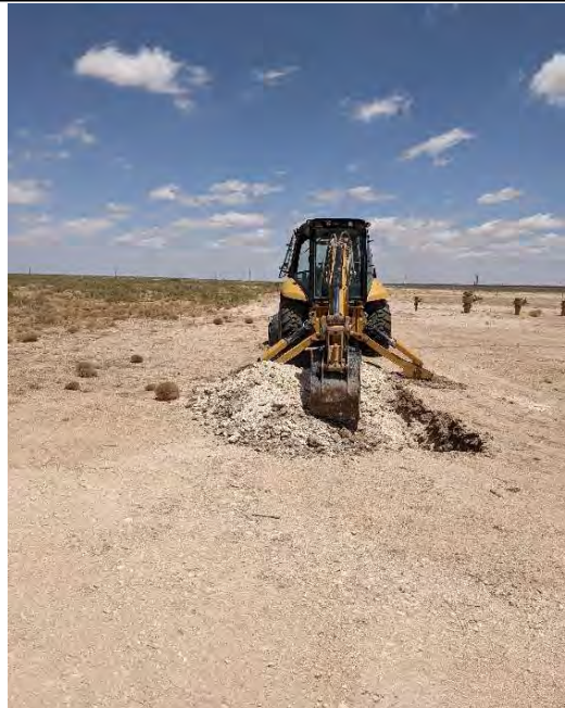
Photograph: 4 Date: 6/3/2022 Description: Delineation activities; near PH03 View: North
