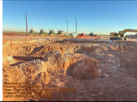
View of excavations from the south side.
