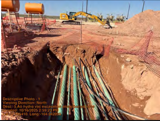
5' hydro vac excavation along buried lines.
