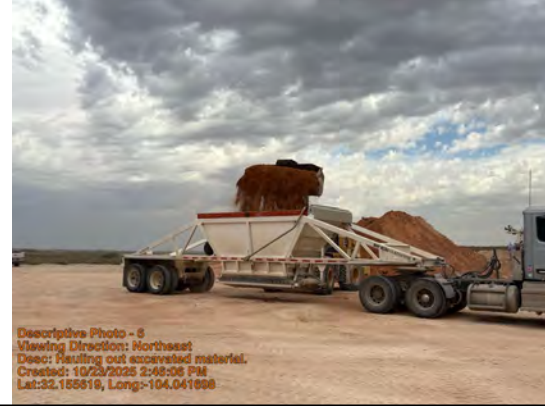
Hauling out excavated material.
