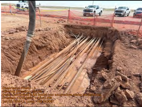
Continued 5' hydro vac excavation along buried lines.
