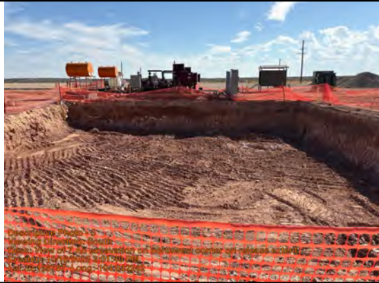
View of 7' excavation on northwest corner on release extent.
