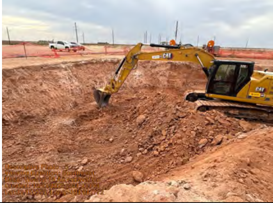
View of 14' excavation.
