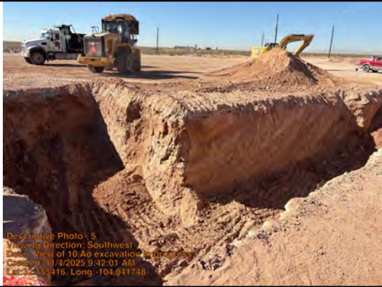
View of 10' excavation in progress.
