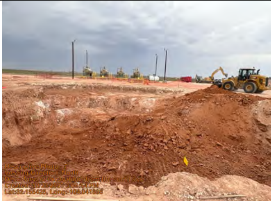
View of excavations from the south side.
