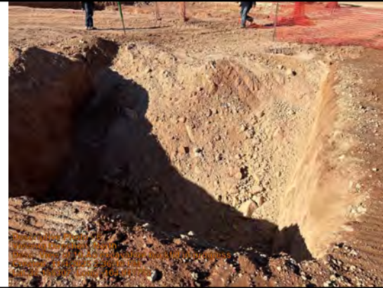
View of 10' excavation backfill in progress.
