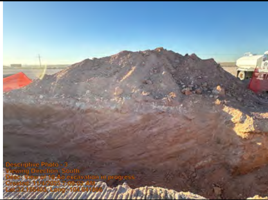
View of 10' excavation in progress.
