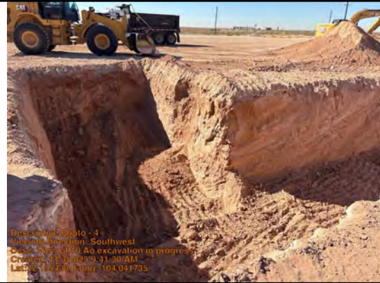
View of 10' excavation in progress.
