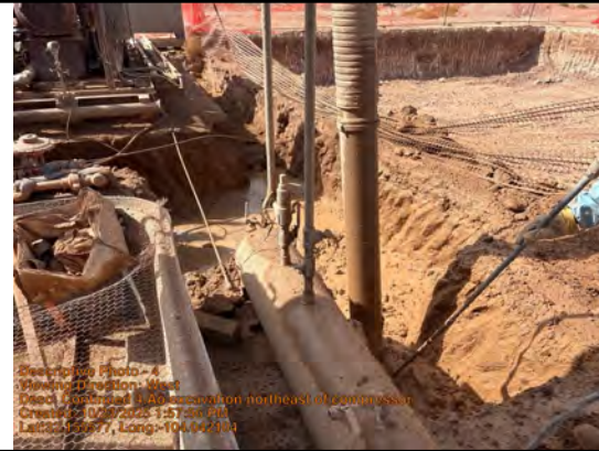
Continued 4' excavation northeast of compressor.
