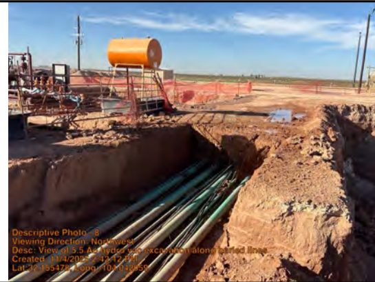
View of 5.5' hydro vac excavation along buried lines.
