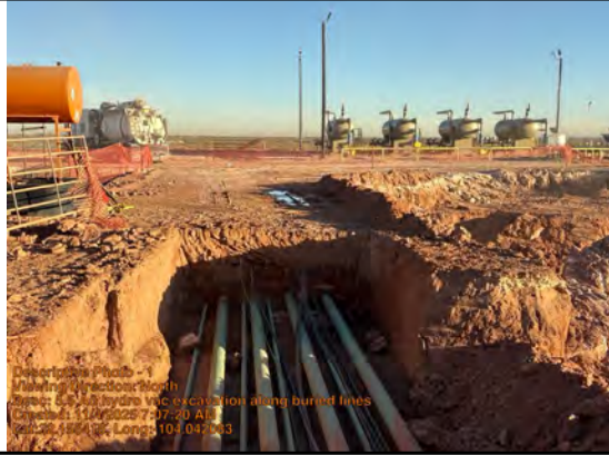
5.5' hydro vac excavation along buried lines.
