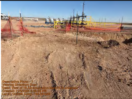
View of 10' excavation backfill in progress.
