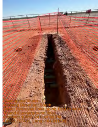
Hydrovac lines going East to west Found 8 underground lines
