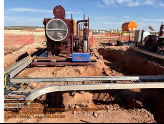
4' hydro vac excavation around compressors.
