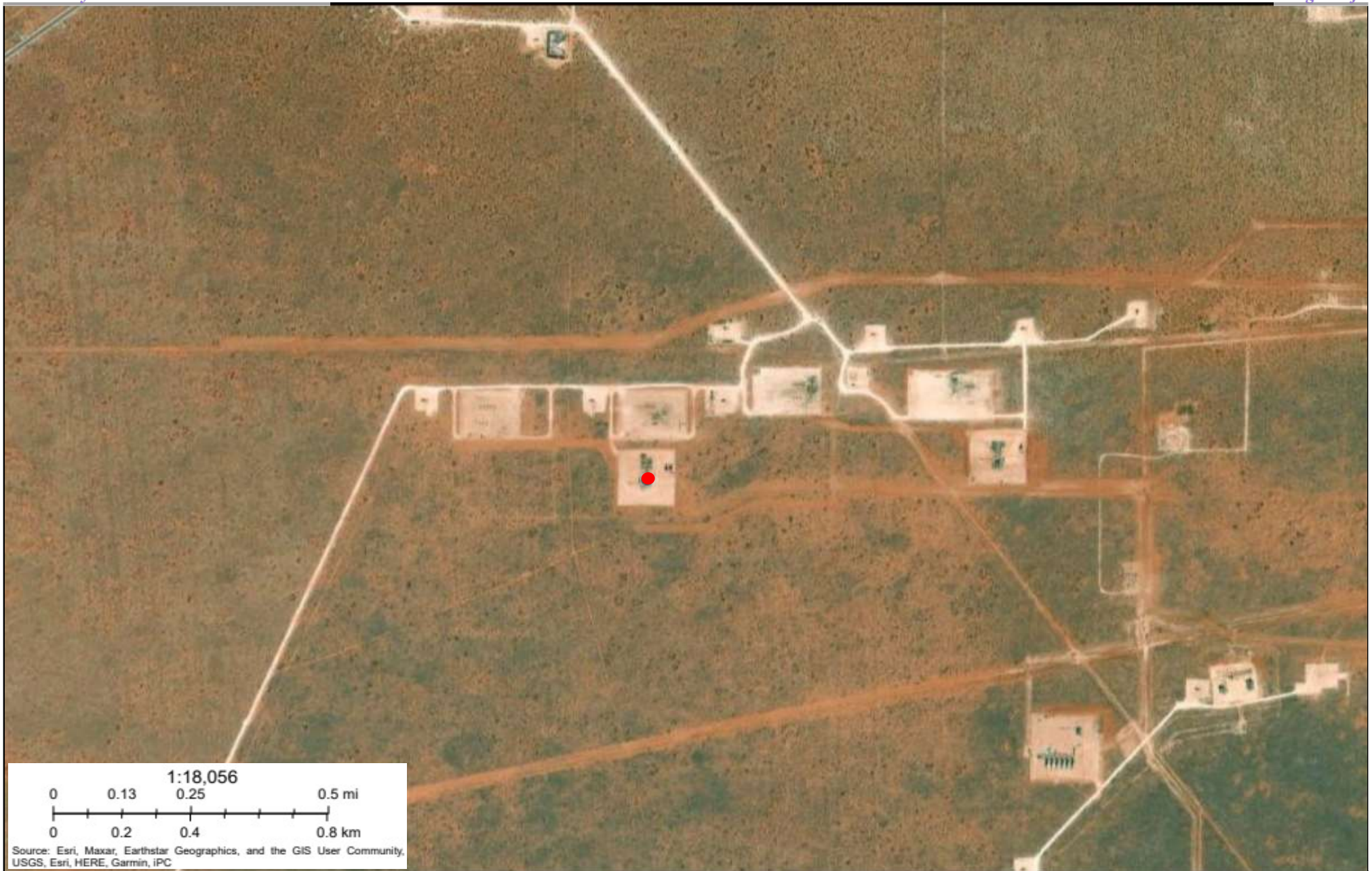
Figure 2 OSE POD Locations Map Devon Energy Production Company, LP Cotton Draw Unit 26 CTB 2 GPS: 32.192712, -103.748725 Eddy County
