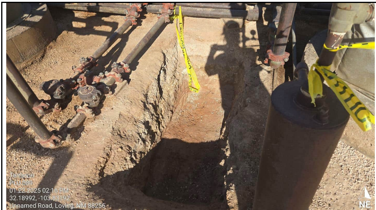
Photo of the additional remediation efforts
