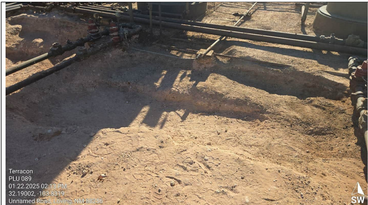
Photo of the additional remediation efforts
