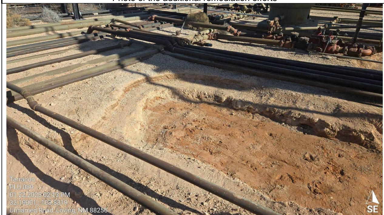
Photo of the additional remediation efforts
