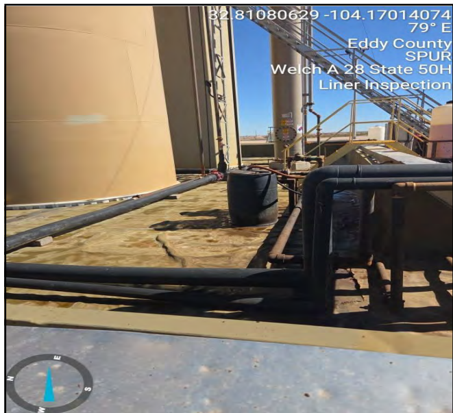
Photo of liner taken during liner inspection facing east.
