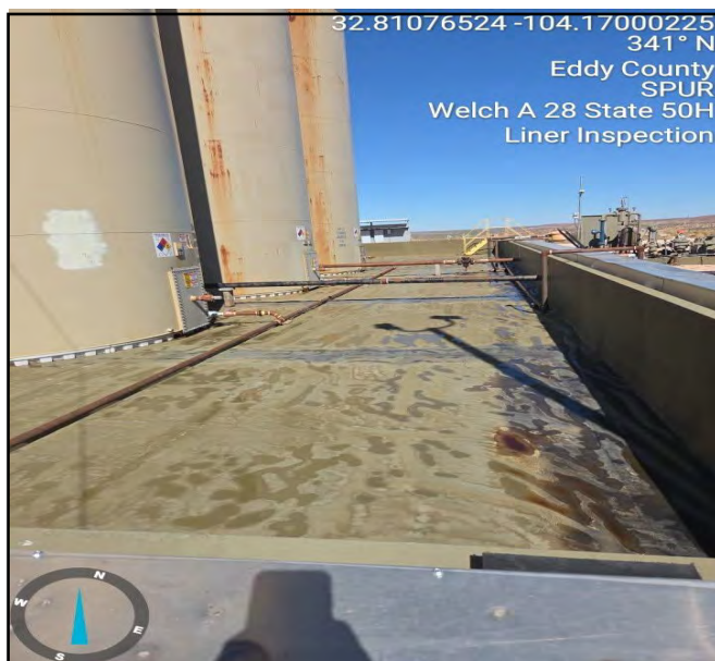
Photo of liner taken during liner inspection facing north.
