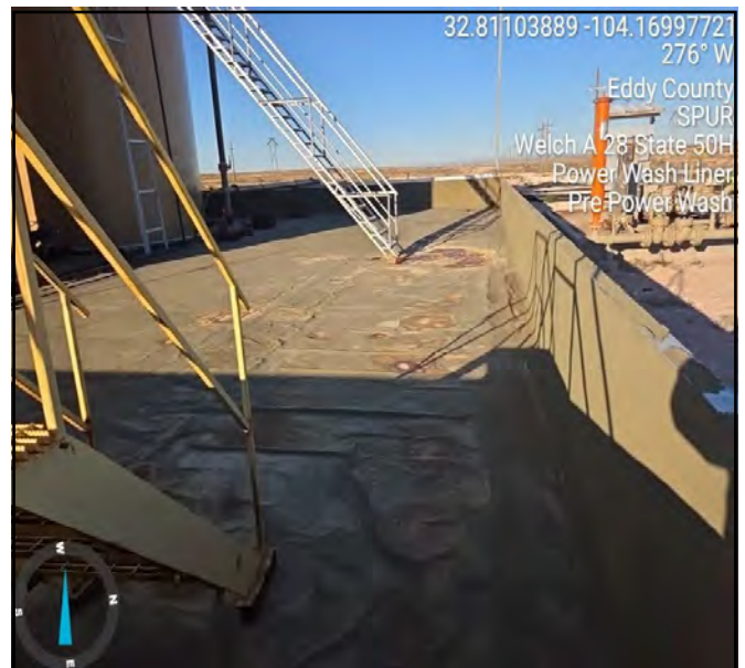
Photograph taken pre power-wash process facing west.
