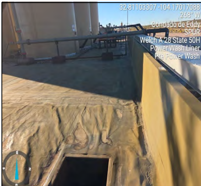
Photograph taken pre power-wash process facing west.
