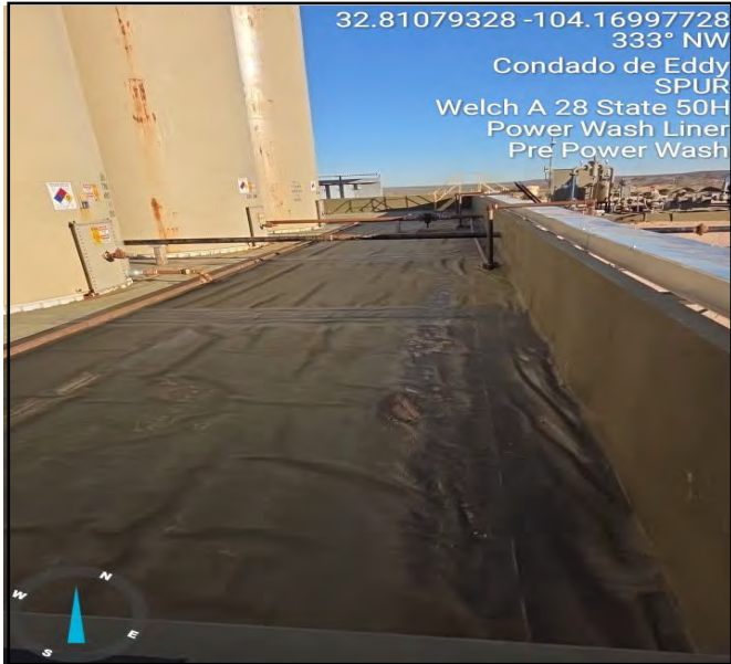
Photograph taken pre power-wash process facing northwest.
