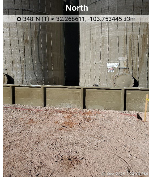
Photograph: 22 Date: 12/31/2025 Description: Delineation Activities at LS01 View: North
