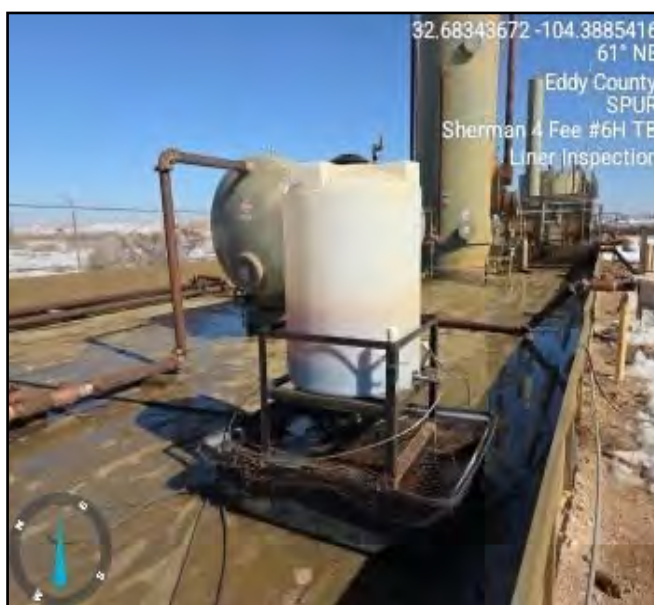
Photograph taken during liner inspection facing northeast.
