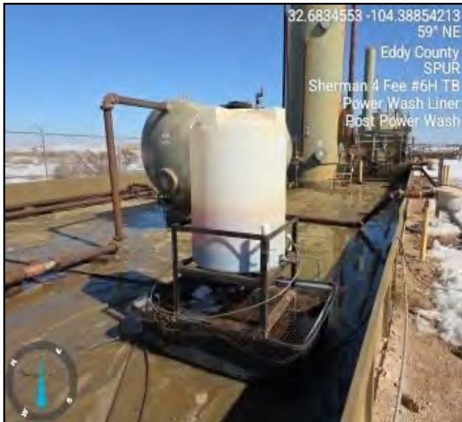
Photo of location taken post power wash facing northeast.
