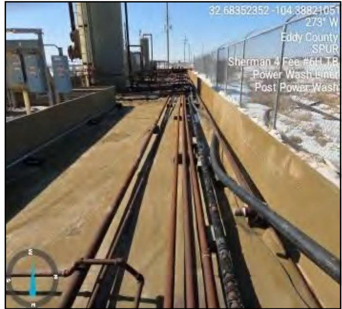
Photo of location taken post power wash facing west.
