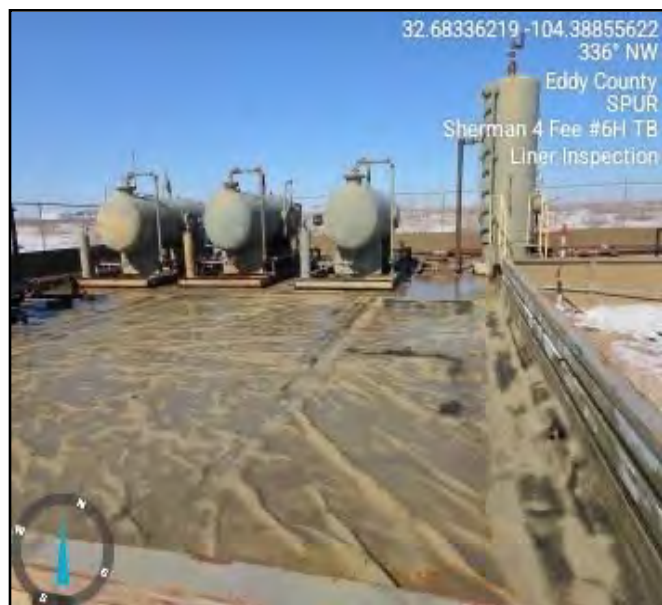
Photograph taken during liner inspection facing northwest.
