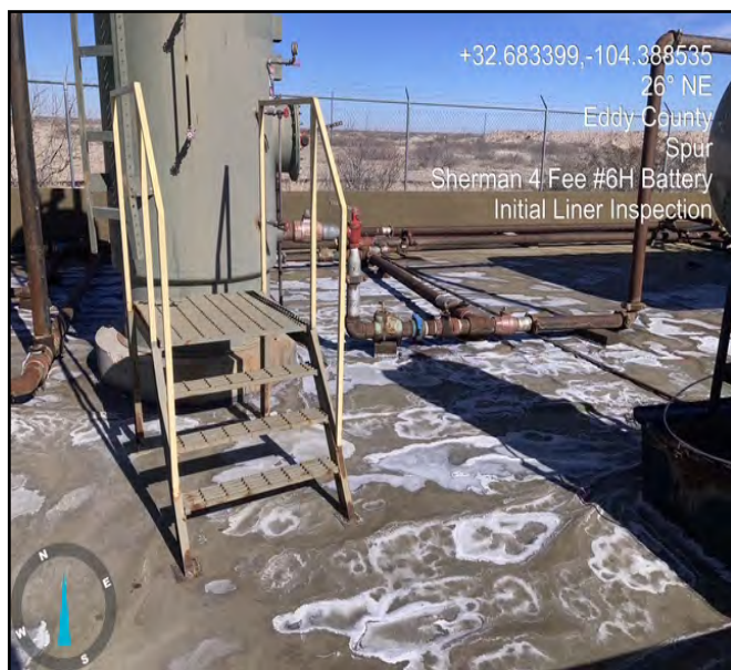
Photo of liner taken during initial liner inspection facing northeast.
