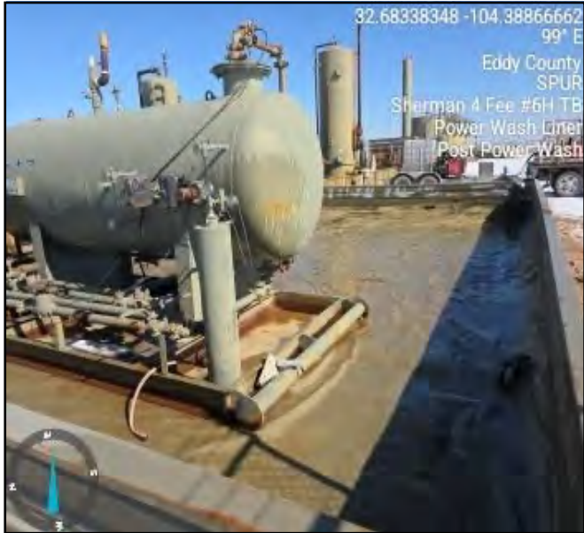
Photo of location taken post power wash facing east.
