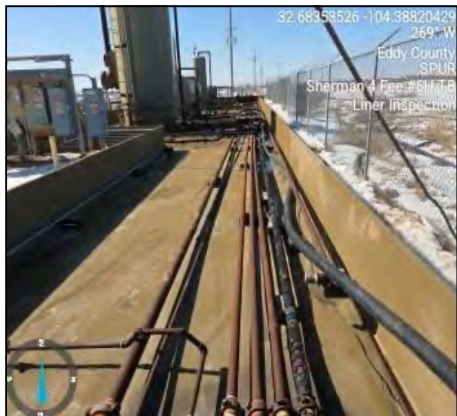
Photograph taken during liner inspection facing west.
