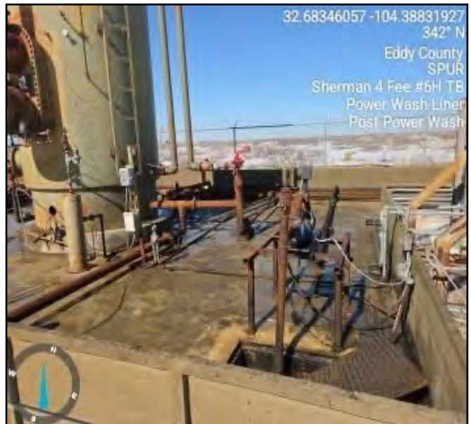
Photo of location taken post power wash facing north.
