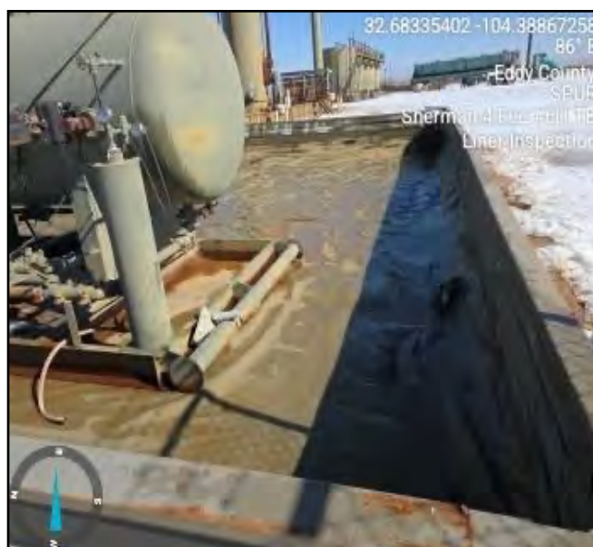
Photograph taken during liner inspection facing east.
