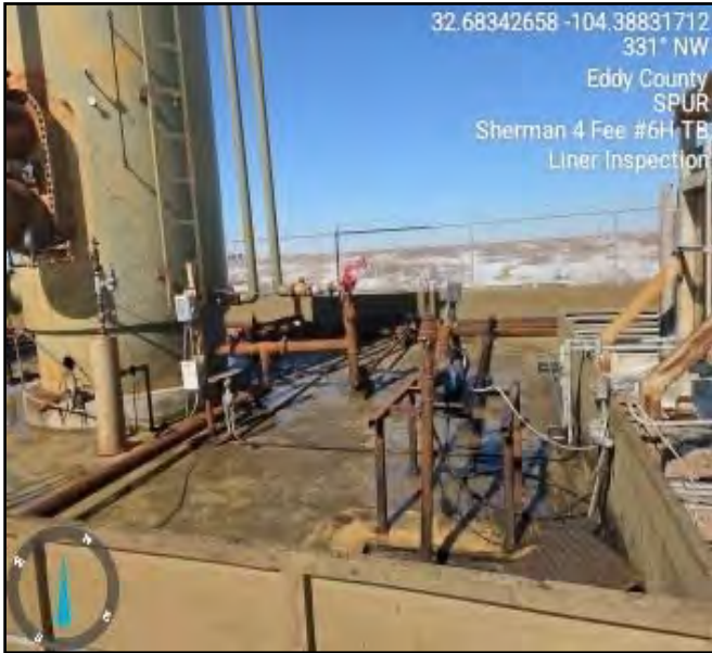
Photograph taken during liner inspection facing northwest.
