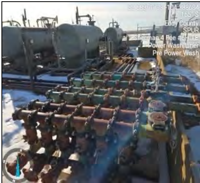
Photograph taken pre- powerwash process facing south.
