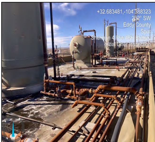
Photo of liner taken during initial liner inspection facing southwest.
