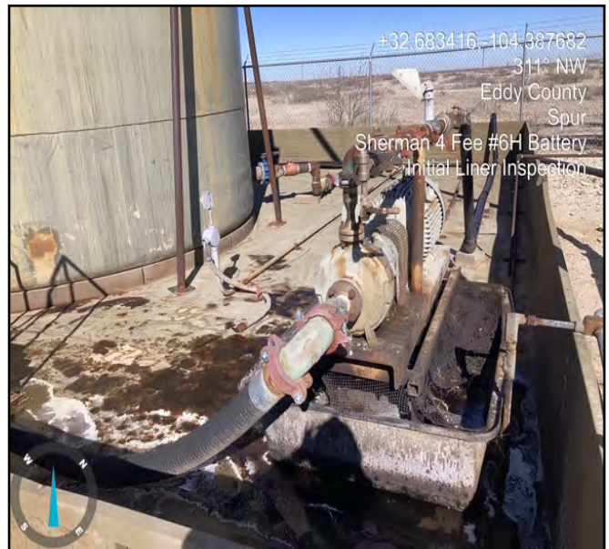
Photo of liner taken during initial liner inspection facing northwest.
