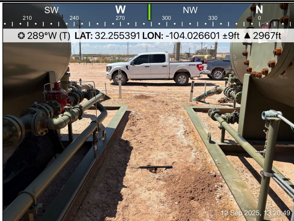
PHOTO 4: Northwestern view during initial delineation activities. 9/12/2025
