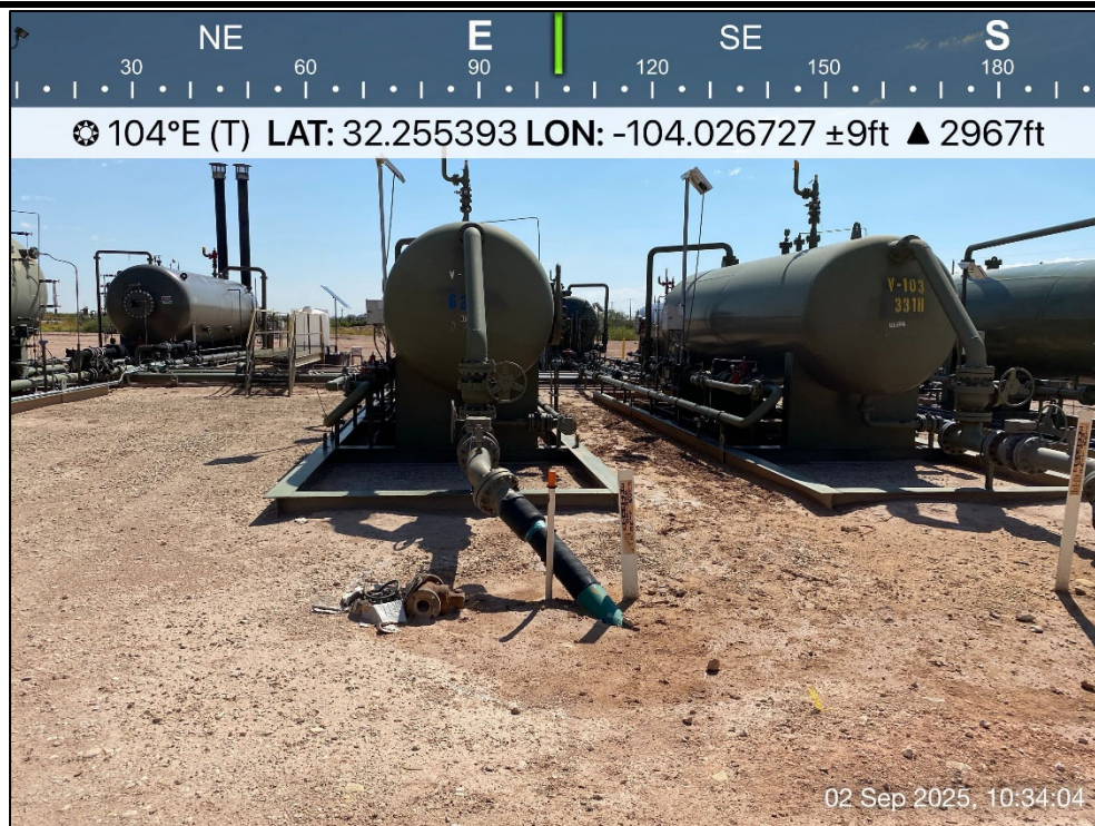
PHOTO 2: Southeastern view during initial site assessment activities. 9/2/2025
