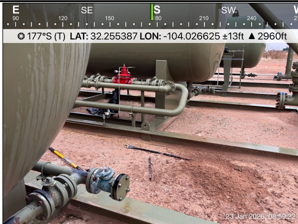
PHOTO 8: Southern view during additional delineation activities. 1/23/2026
