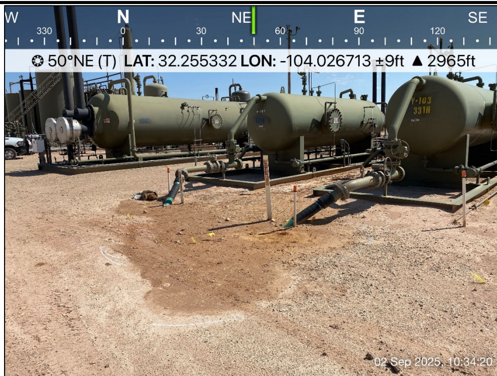
PHOTO 1: Northeastern view during initial site assessment activities. 9/2/2025
