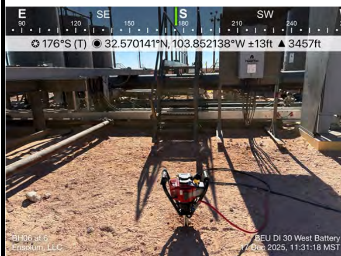
Photograph: 11 Date: 12/17/2025 Description: Delineation activities, near BH06 View: South
