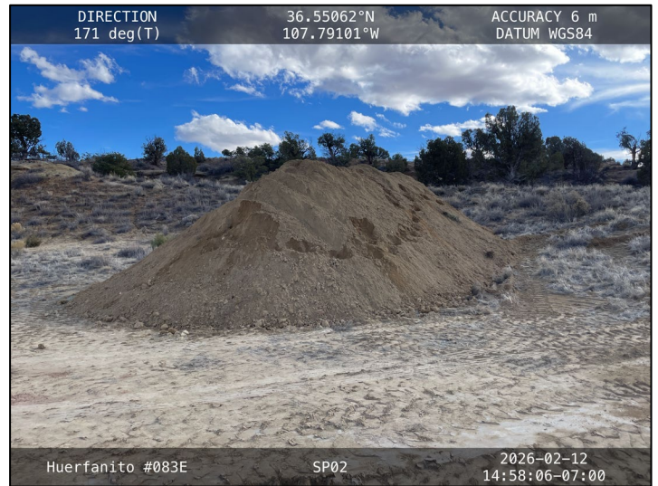
Photograph: 10 Date: 02/12/2026 Description: Overburden that that screened as clean, sampled as SP02 and stored for backfill. View: South
