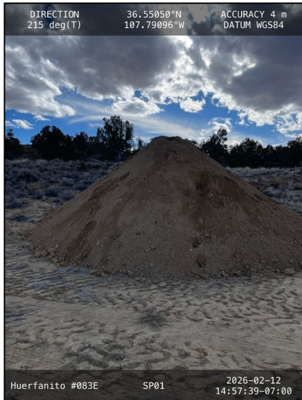
Photograph: 9 Date: 02/12/2026 Description: Overburden that that screened as clean, sampled as SP01 and stored for backfill. View: Southwest
