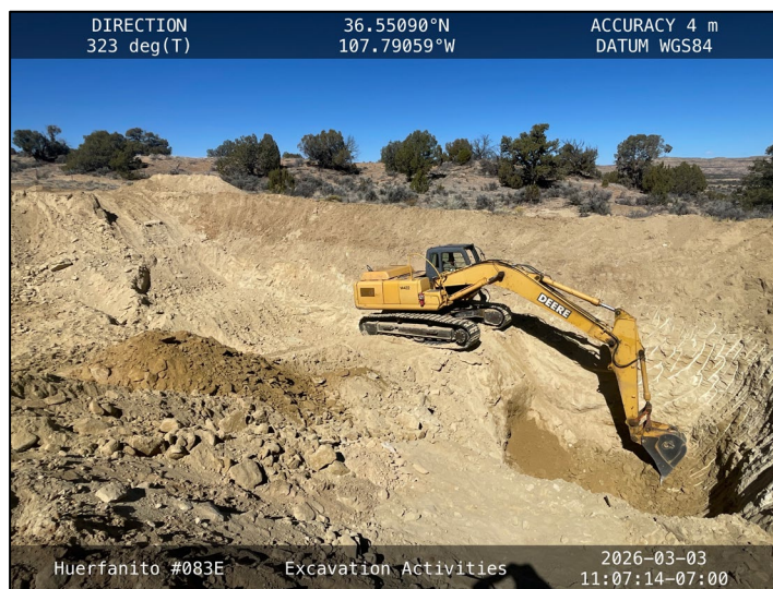
Photograph: 6 Date: 03/03/2026 Description: Removing contaminated floor FS06 and sampling the newly exposed floors and sidewalls. View: Northwest
