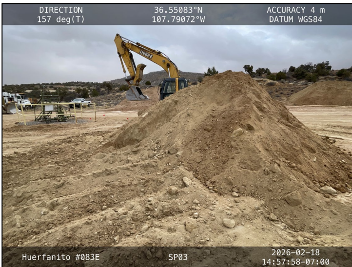
Photograph: 9 Date: 02/12/2026 Description: Overburden that that screened as clean, sampled as SP01 and stored for backfill. View: Southwest
