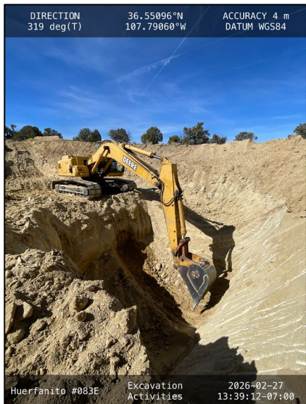
Photograph: 5 Date: 02/27/2026 Description: Removing contaminated floor sample FS19 and sampling the newly exposed floor. View: Northwest
