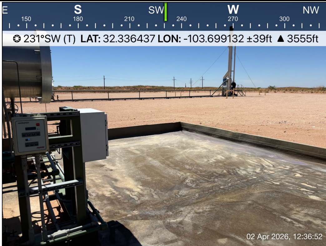
PHOTO 10: Southwestern view during liner inspection activities. 4/2/2026
