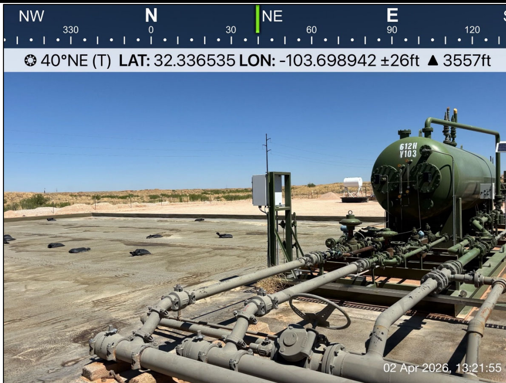
PHOTO 17: Northeastern view during liner inspection activities. 4/2/2026
