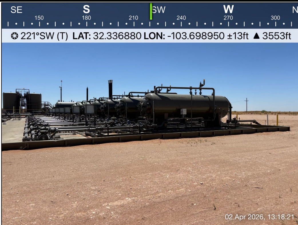
PHOTO 8: Southwestern view outside of containment during liner inspection activities. 4/2/2026
