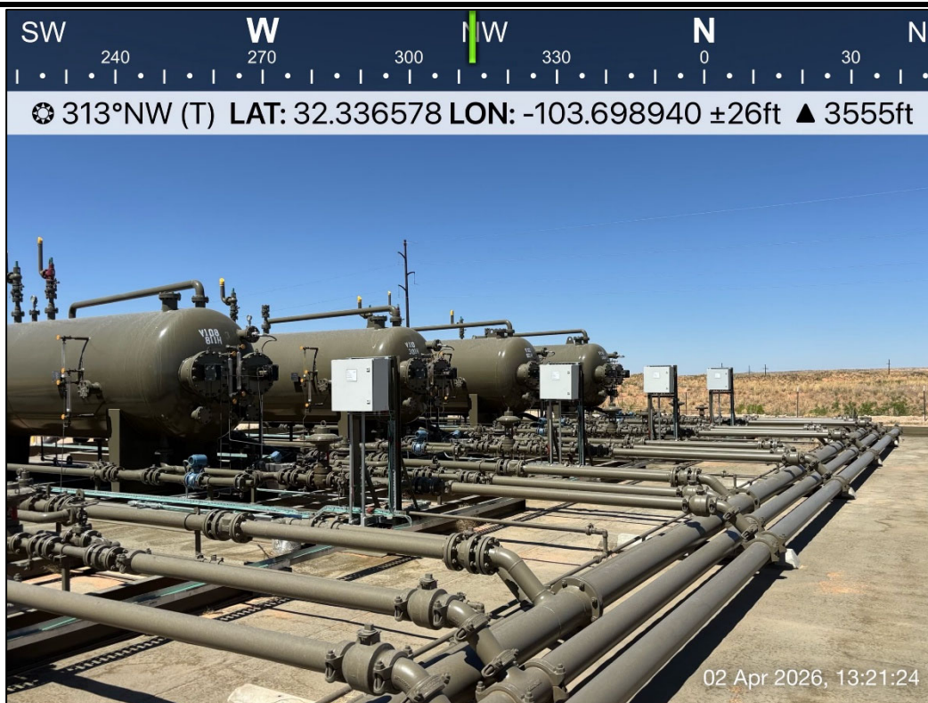
PHOTO 18: Northwestern view during liner inspection activities. 4/2/2026
