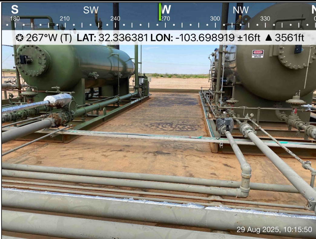
PHOTO 18: Western view during liner inspection activities. 8/29/2025
