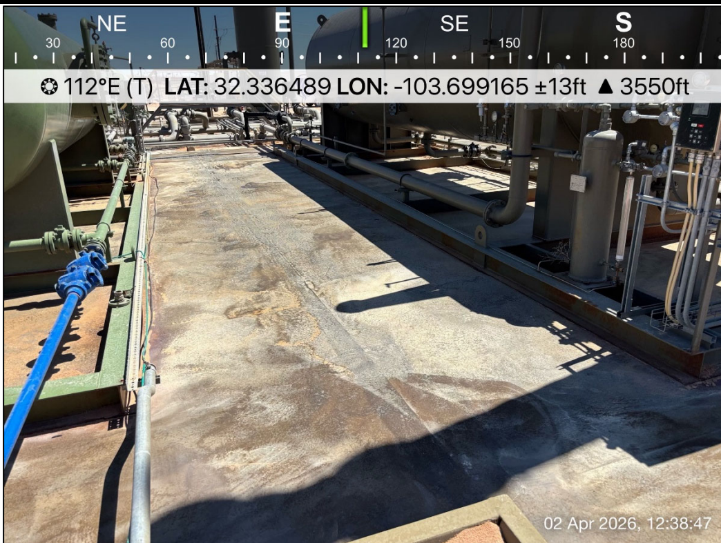
PHOTO 16: Southeastern view during liner inspection activities. 4/2/2026
