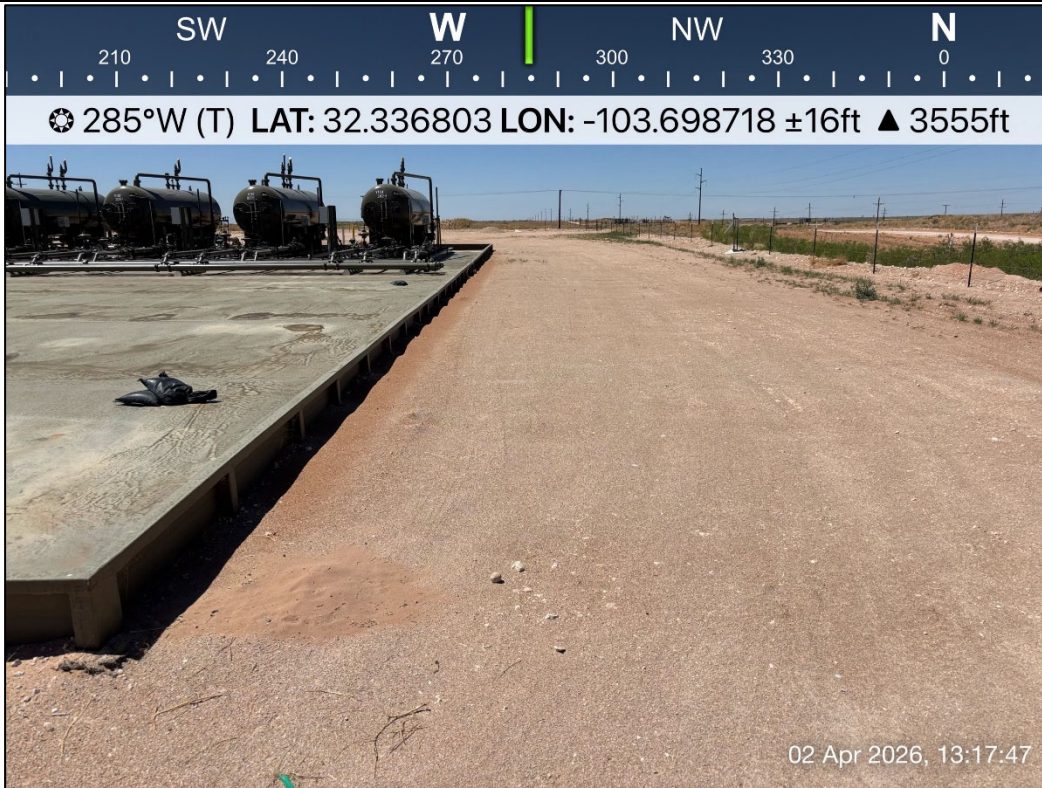
PHOTO 7: Northwestern view outside of containment during liner inspection activities. 4/2/2026
