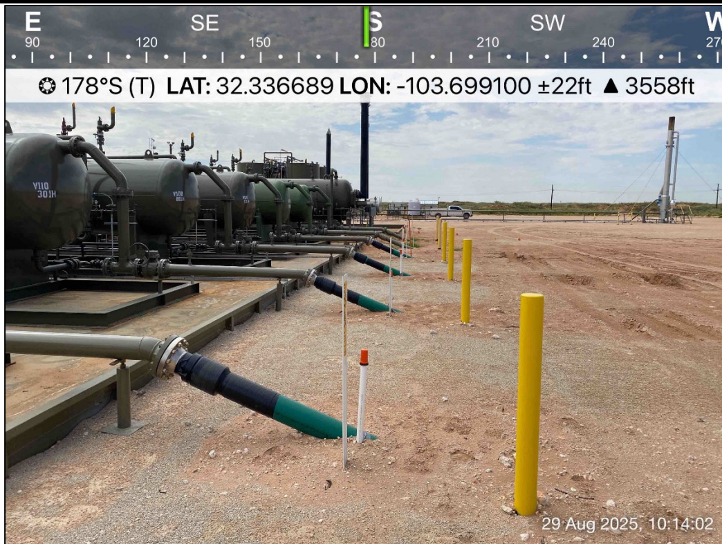
PHOTO 8: Southwestern view outside of containment during liner inspection activities. 8/29/2025
