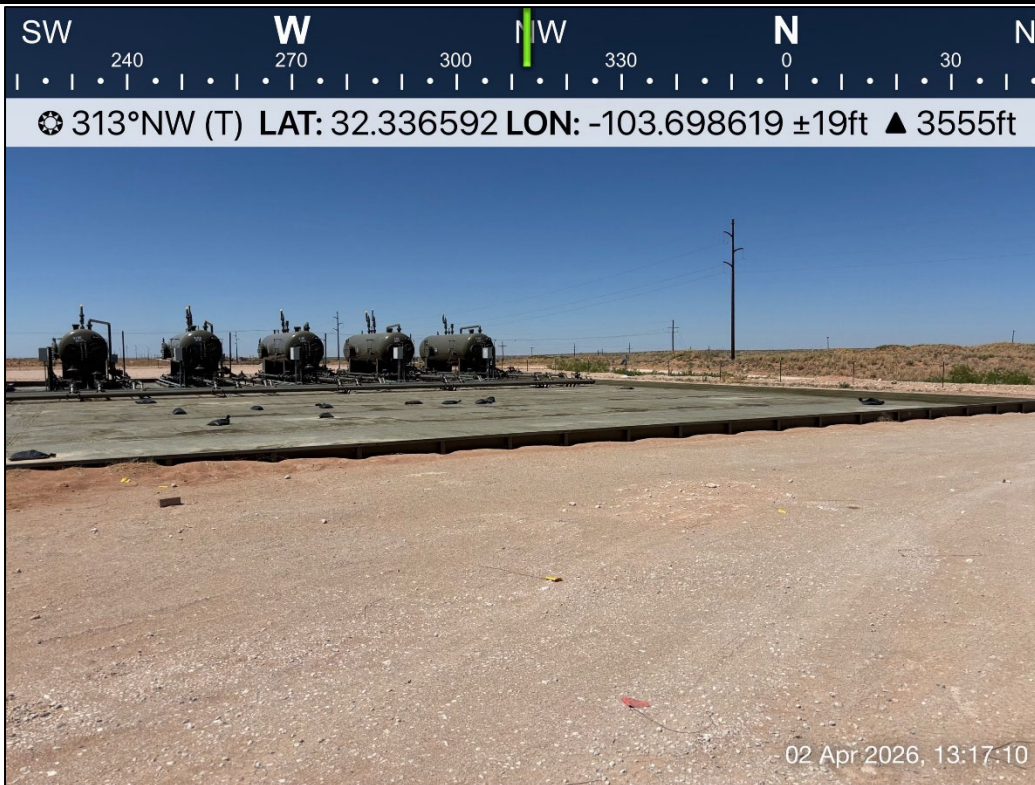
PHOTO 6: Northwestern view outside of containment during liner inspection activities. 4/2/2026
