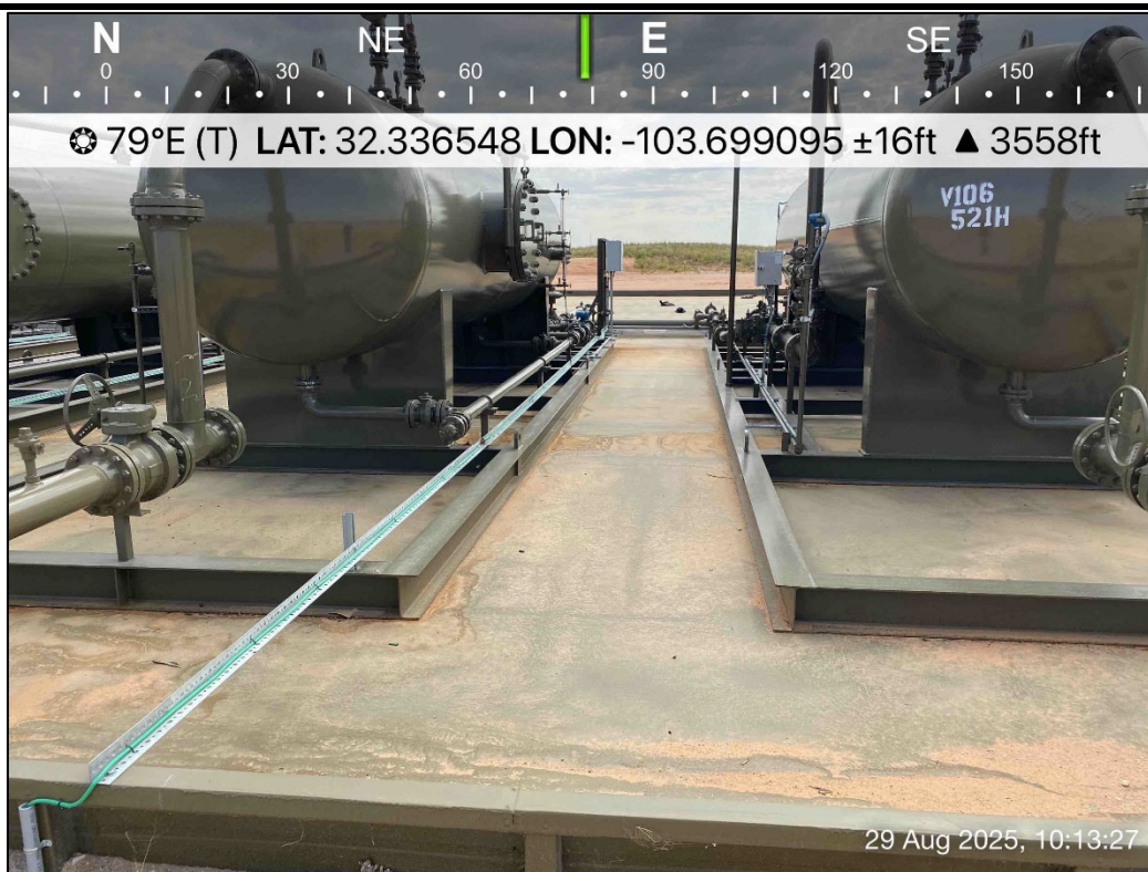
PHOTO 19: Northeastern view during liner inspection activities. 8/29/2025
