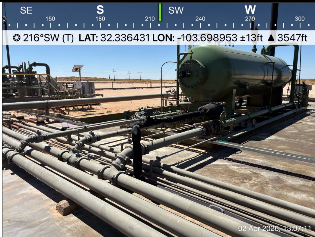
PHOTO 14: Southwestern view during liner inspection activities. 4/2/2026
