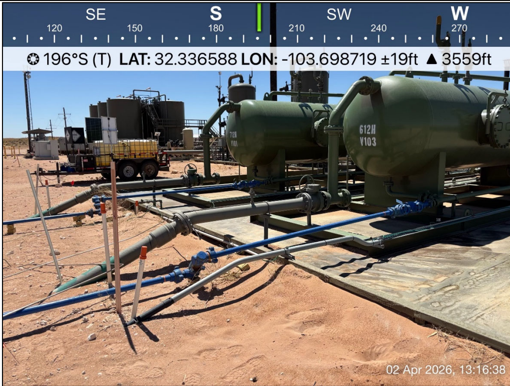
PHOTO 5: Southwestern view outside of containment during liner inspection activities. 4/2/2026
