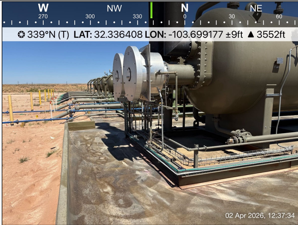
PHOTO 11: Northwestern view during liner inspection activities. 4/2/2026
