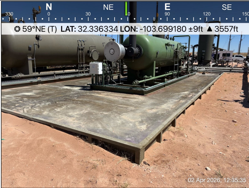
PHOTO 3: Northeastern view outside of containment during liner inspection activities. 4/2/2026
