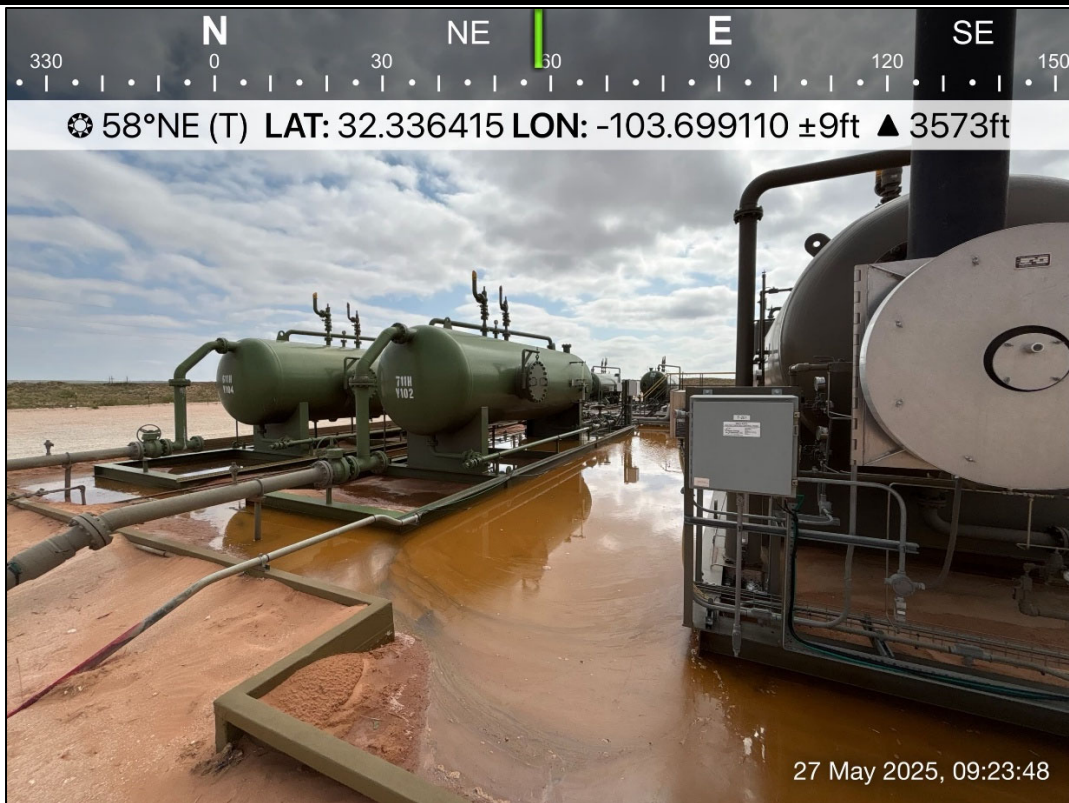
PHOTO 2: Northeastern view during initial site assessment activities. 5/27/2025
