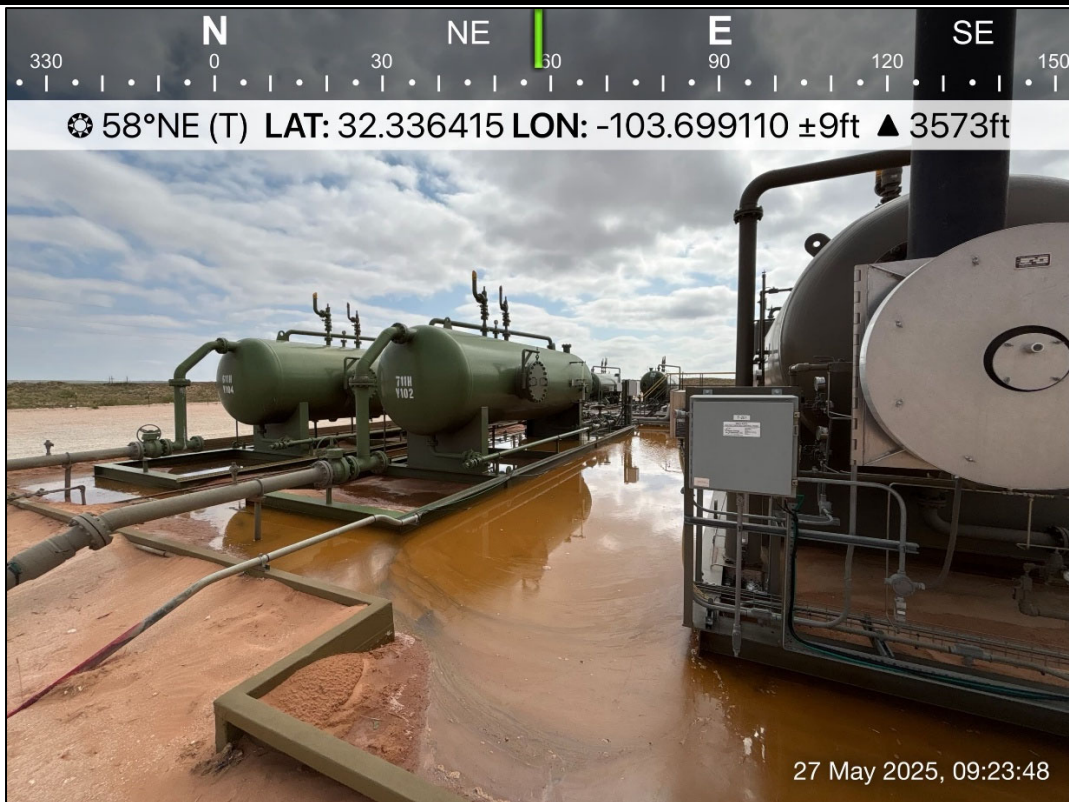
PHOTO 2: Northeastern view during initial site assessment activities. 5/27/2025
