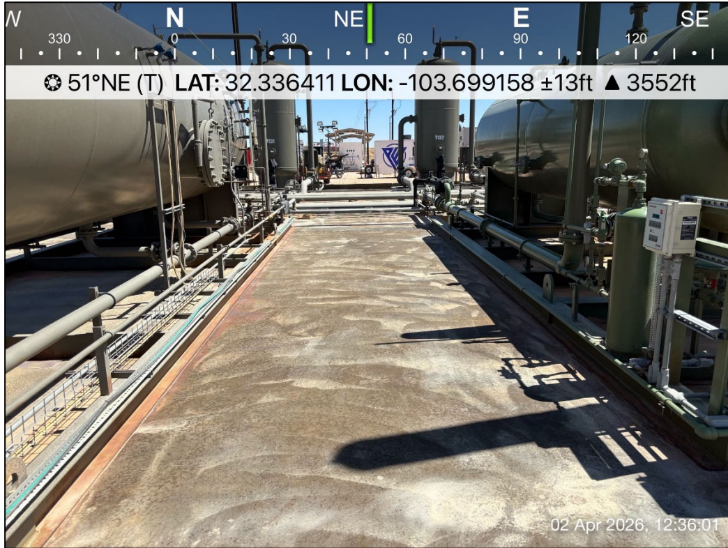
PHOTO 9: Northeastern view during liner inspection activities. 4/2/2026
