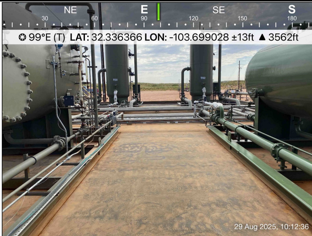
PHOTO 10: Southeastern view during liner inspection activities. 8/29/2025
