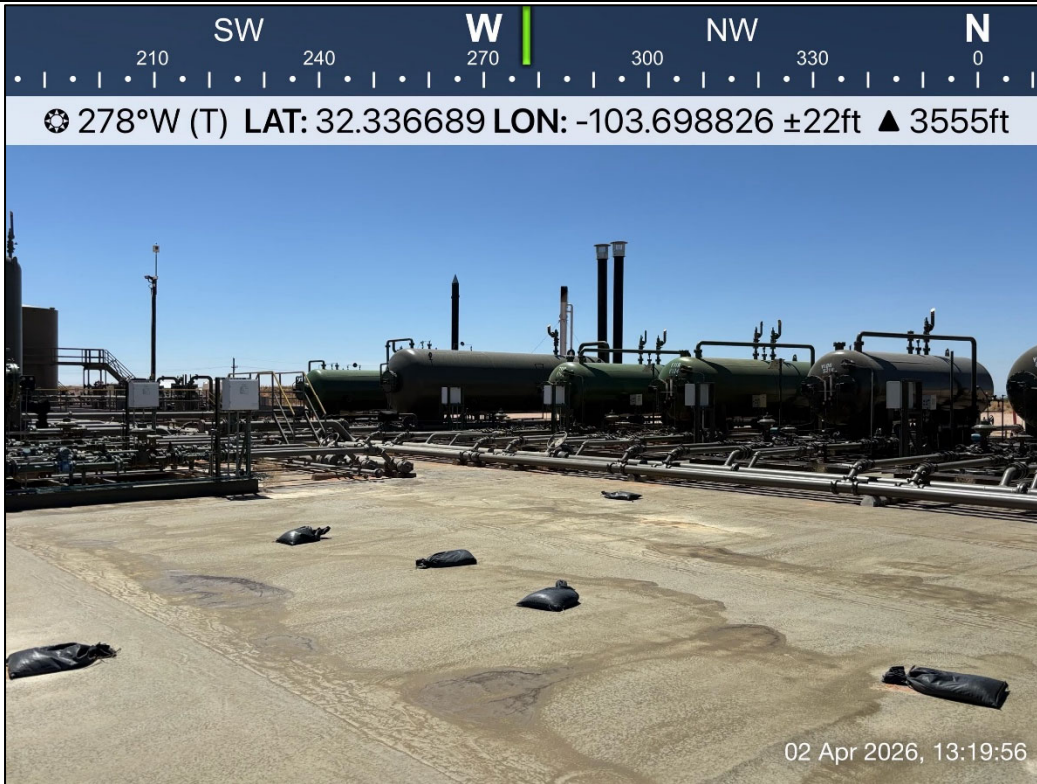
PHOTO 19: Northwestern view during liner inspection activities. 4/2/2026
