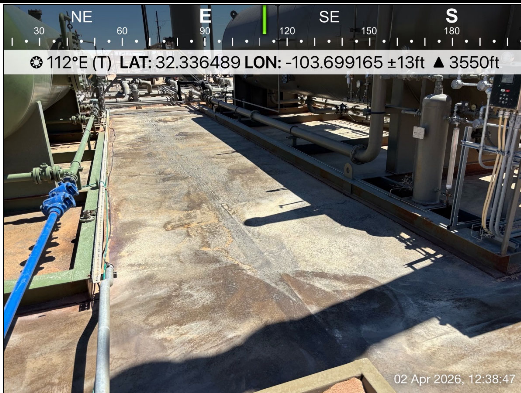
PHOTO 12: Southeastern view during liner inspection activities. 4/2/2026
