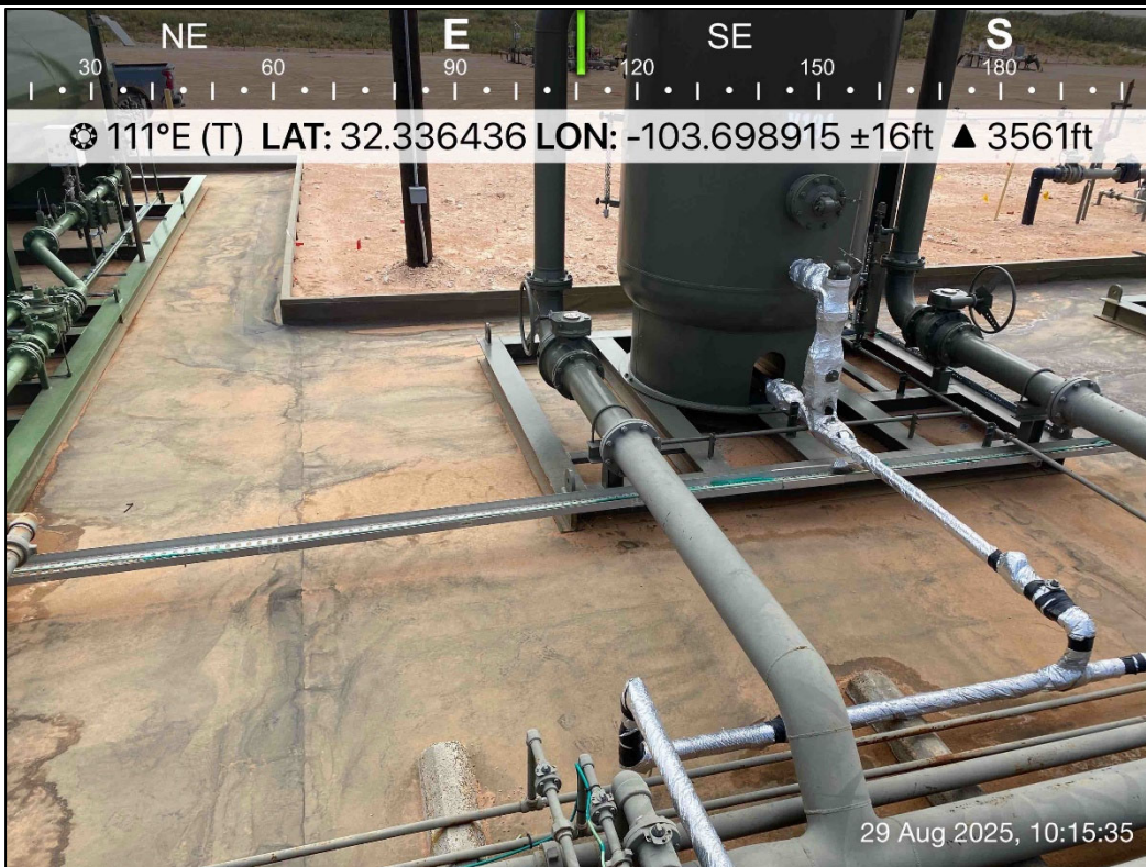
PHOTO 14: Southeastern view during liner inspection activities. 8/29/2025
