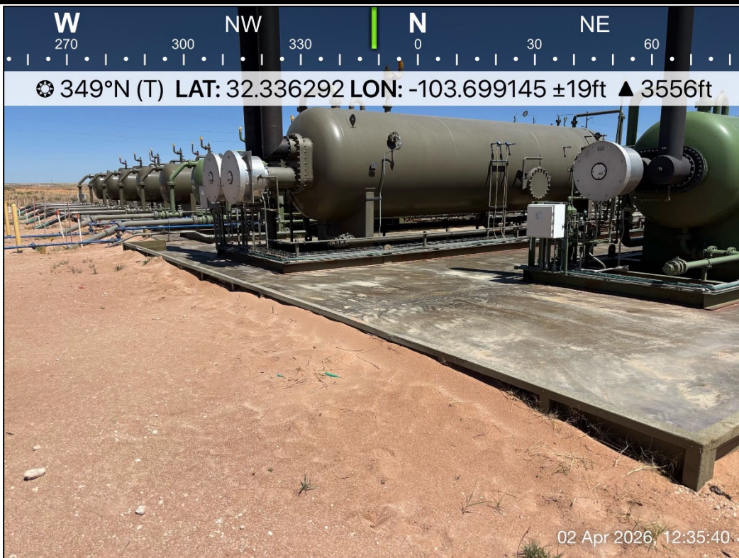
PHOTO 4: Northwestern view outside of containment during liner inspection activities. 8/29/2025
