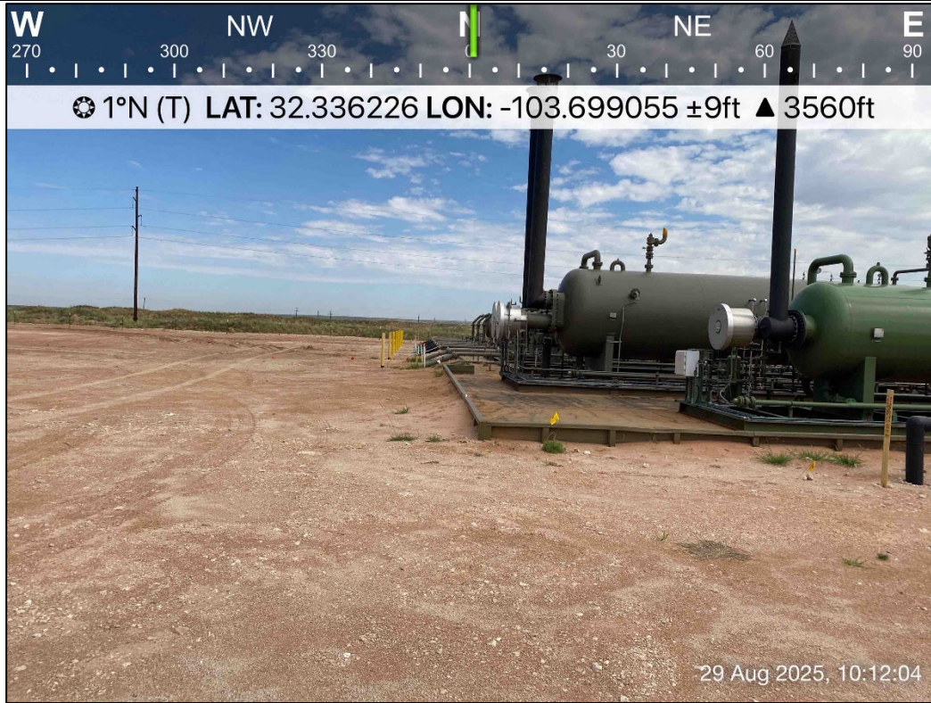
PHOTO 7: Northern view outside of containment during liner inspection activities. 8/29/2025
