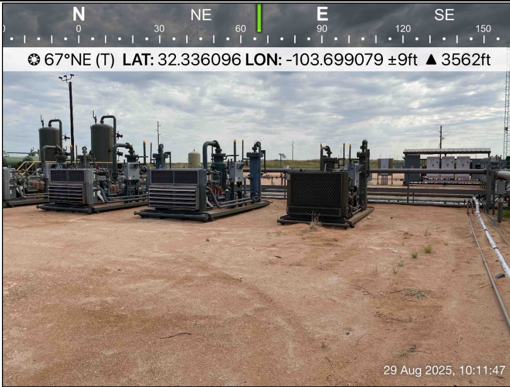
PHOTO 5: Northeastern view outside of containment during liner inspection activities. 8/29/2025
