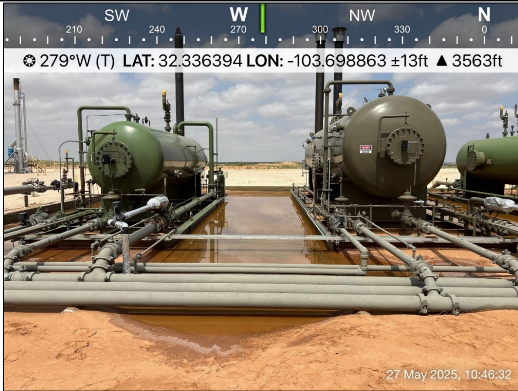
PHOTO 1: Northwestern view during initial site assessment activities. 5/27/2025
