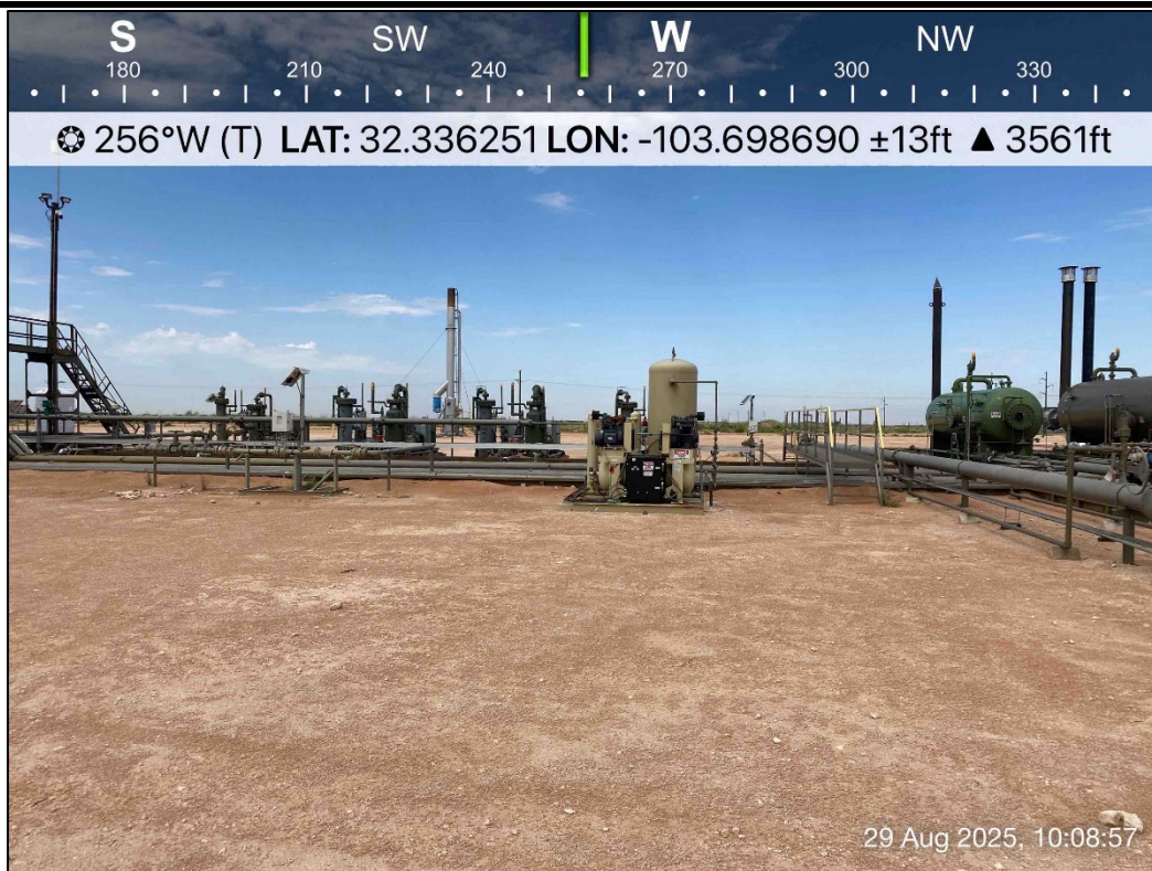
PHOTO 4: Southwestern view outside of containment during liner inspection activities. 8/29/2025
