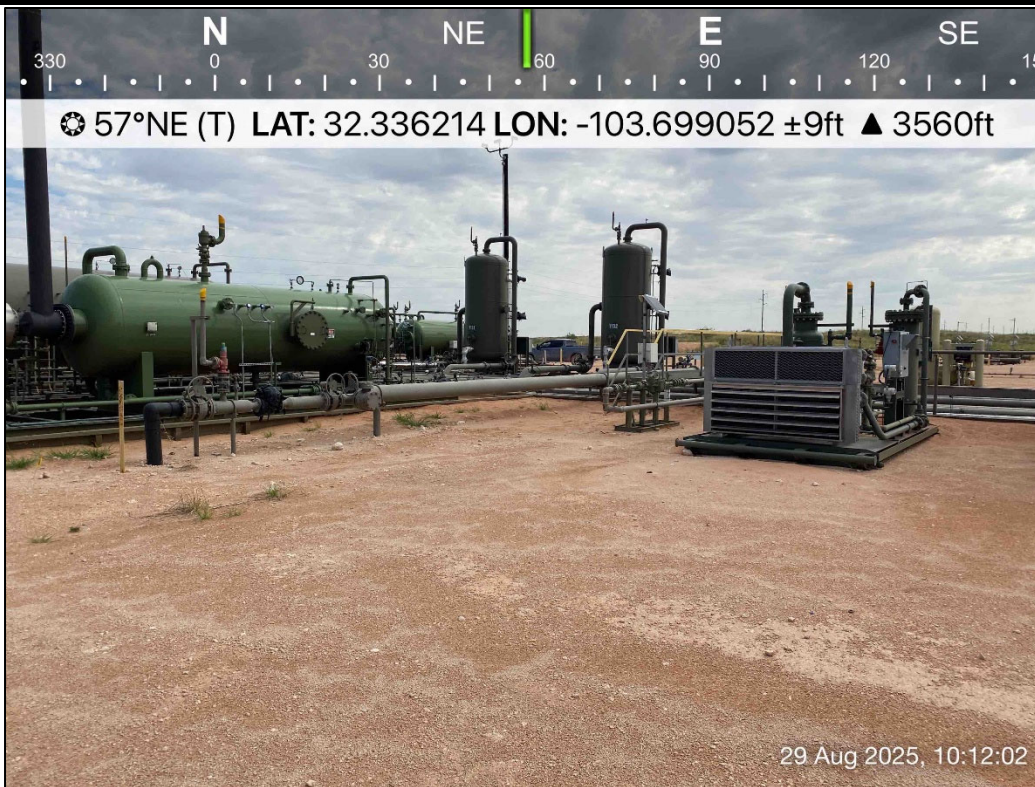
PHOTO 6: Northeastern view outside of containment during liner inspection activities. 8/29/2025
