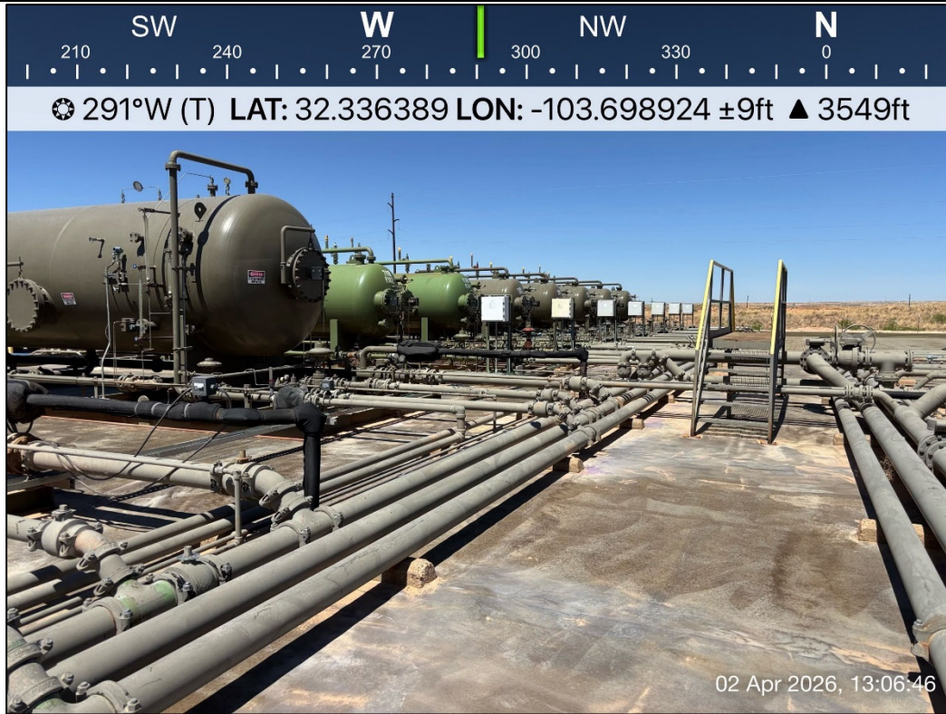
PHOTO 13: Northwestern view during liner inspection activities. 4/2/2026
