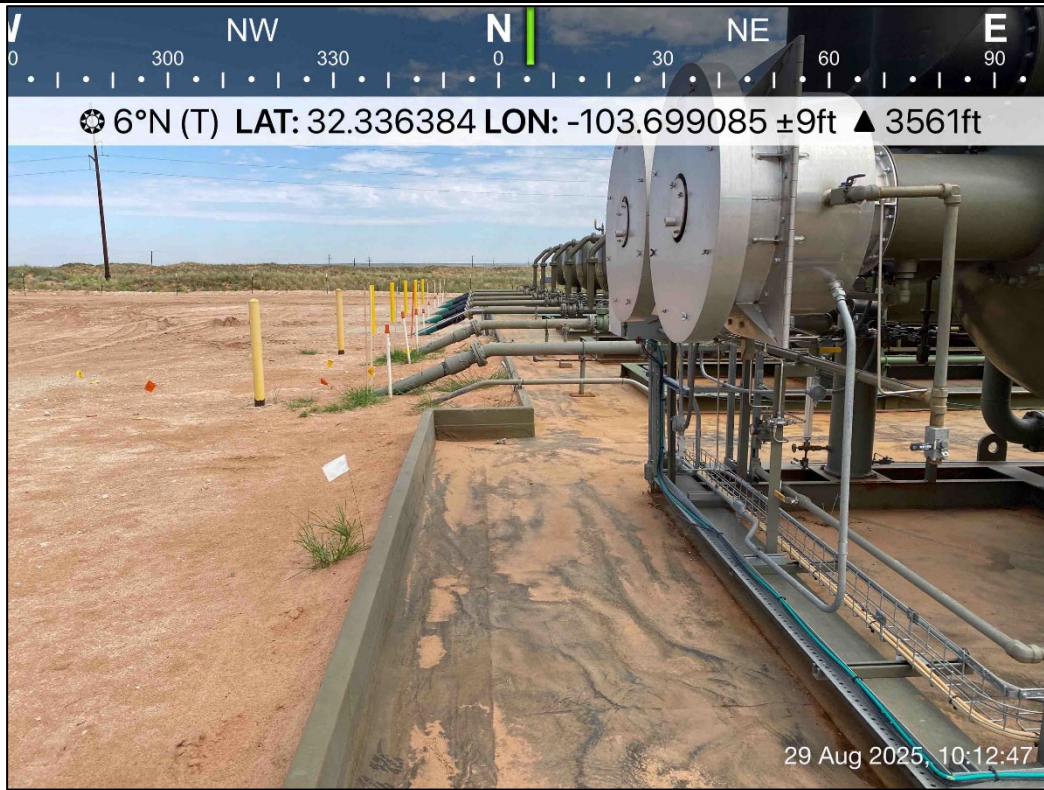
PHOTO 11: Northeastern view during liner inspection activities. 8/29/2025
