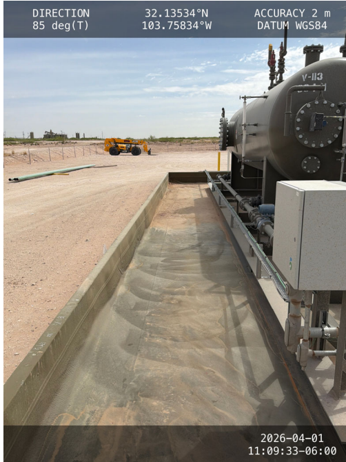
Photo 9 Photo of containment towards east.
