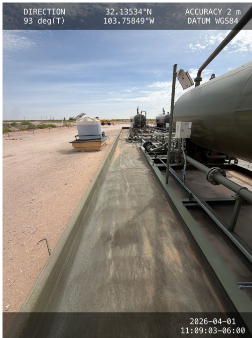
Photo 3 Photo of containment towards east.
