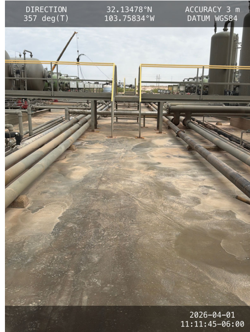
Photo 10 Photo of containment towards north.
