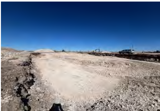
View to N of W excavation wall (2/6/26).
