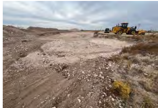
View to N of excavation from S wall (11/20/25).
