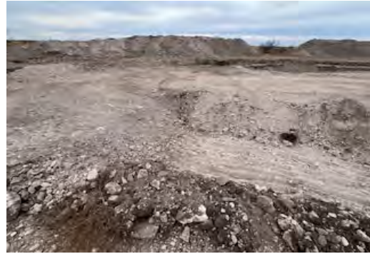
View to NW along S wall of excavation (11/20/25).
