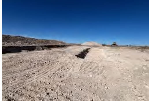
View to N of excavation (2/6/26).
