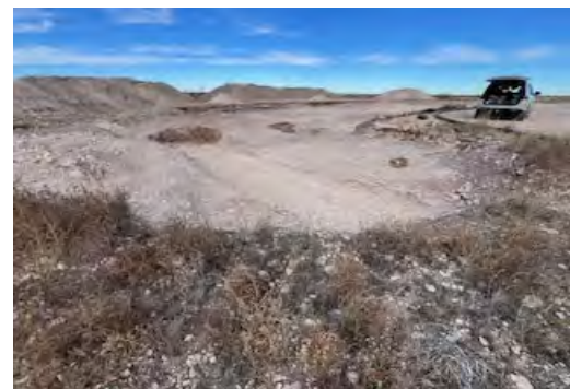
View to NW of S end of excavation (1/13/26).
