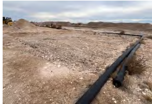
View to SW of NE part of excavation (11/20/25).
