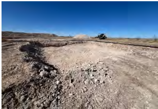
View to NW of NE portion of excavation (2/6/26).
