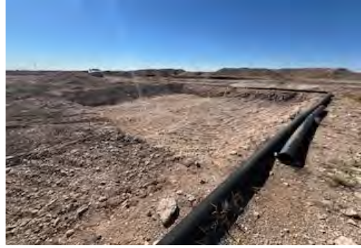
View to SW of NE portion of excavation (2/6/26).
