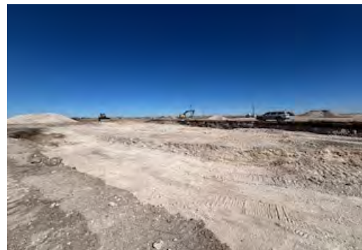
View to NE of E excavation wall (2/6/26).
