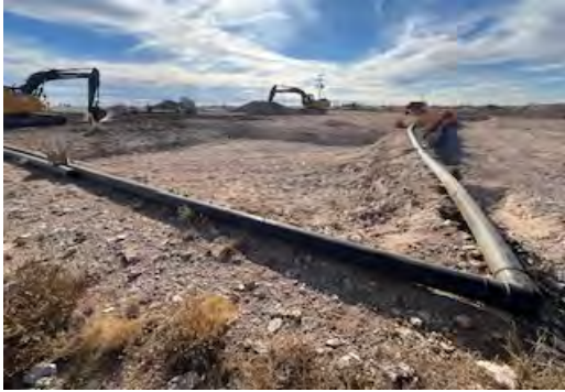
View to S of NE part of excavation (1/13/26).
