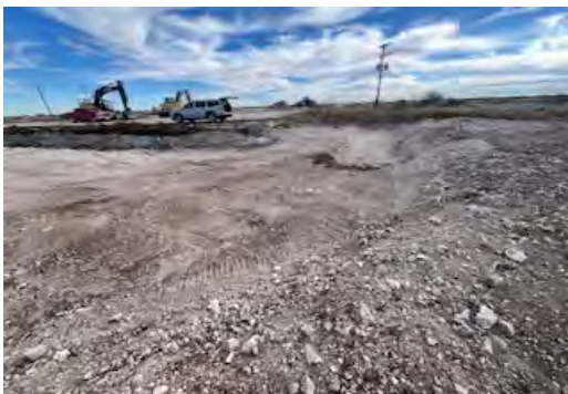
View to E of S end of excavation (1/13/26).
