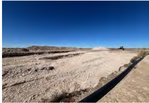
View to NW of excavation (2/6/26).
