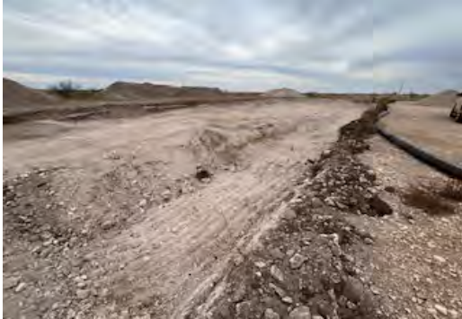
View to N of excavation (11/20/25).
