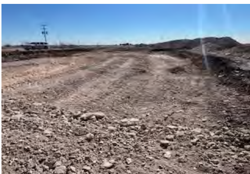
View to S of W excavation wall (2/6/26).
