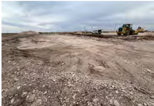
View to N of excavation (11/20/25).
