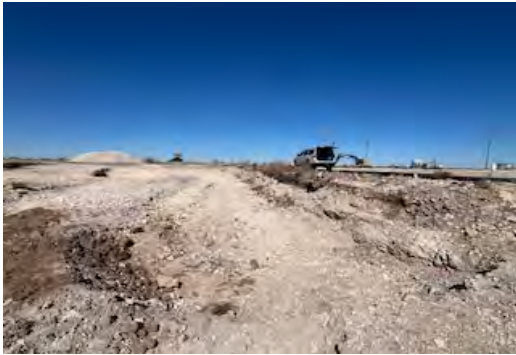
View to N of excavation (2/6/26).
