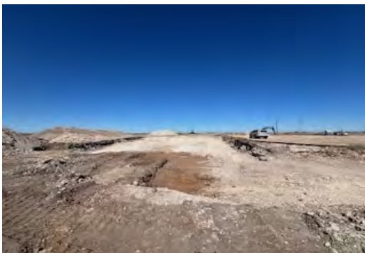
View to N of excavation (2/6/26).
