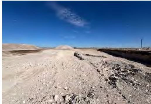
View to N of excavation (3/6/26).
