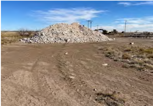
View to N of stockpiled soil (1/13/26).
