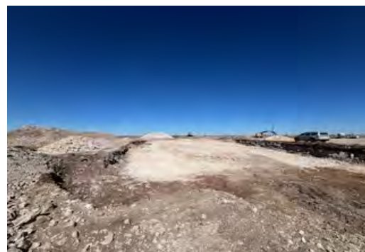
View to N of excavation (2/6/26).
