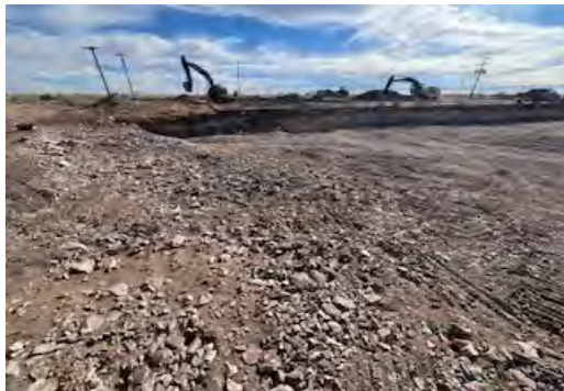
View to E of N side of excavation (1/13/26).
