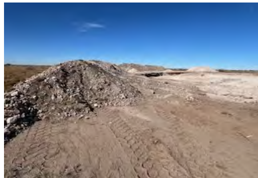
View to N of stockpiled soil (1/13/26).
