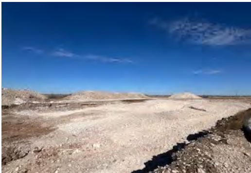
View to NW of excavation (3/6/26).
