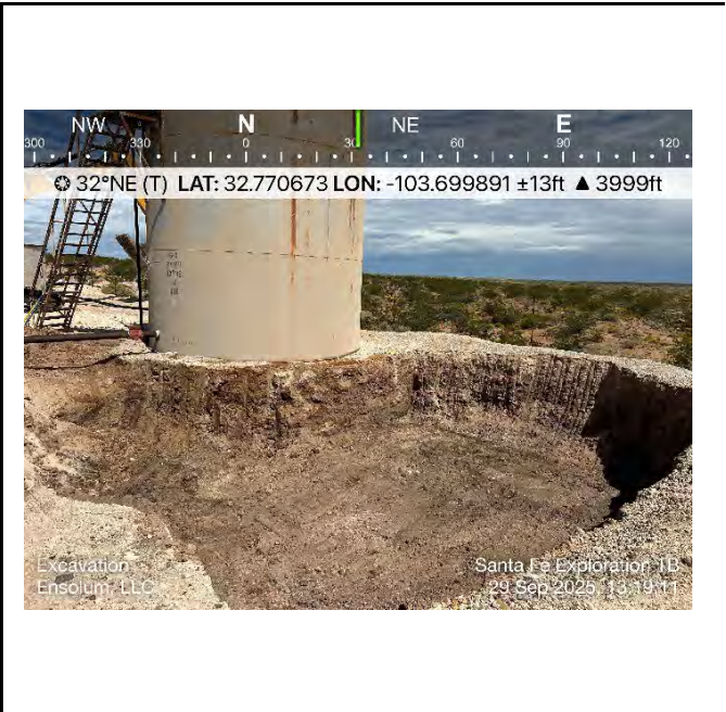
Photograph 20 Date: 9/29/2025 Description: Excavation Activities View: Northeast
