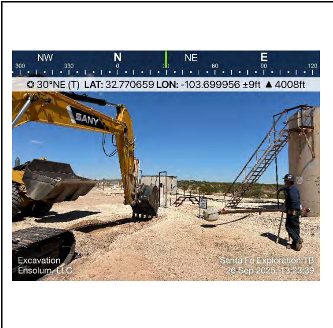
Photograph 19 Date: 9/26/2025 Description: Excavation Activities View: Northeast
