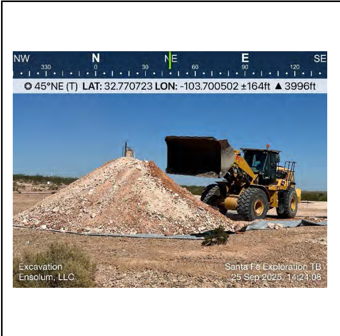
Photograph 17 Date: 9/25/2025 Description: Excavation Activities View: Northeast
