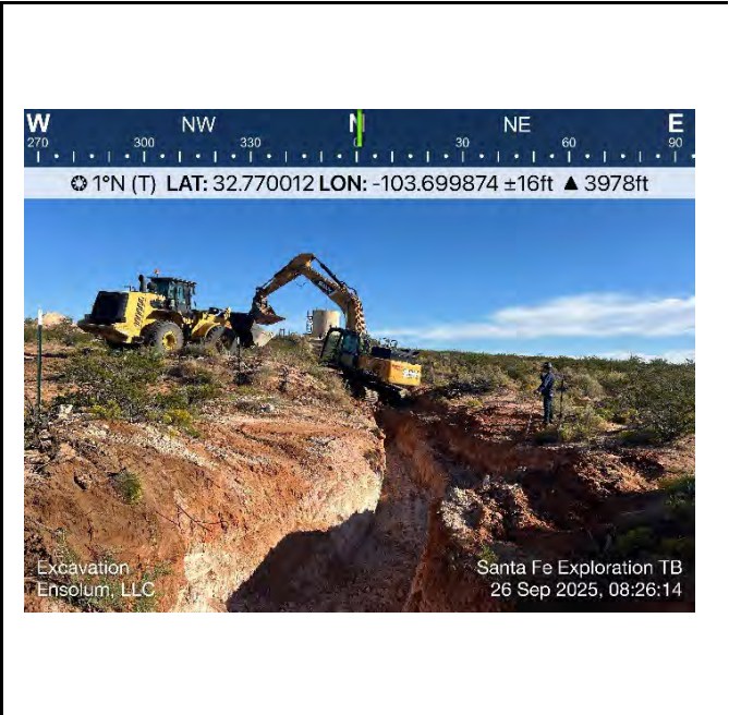
Photograph 18 Date: 9/26/2025 Description: Excavation Activities View: North
