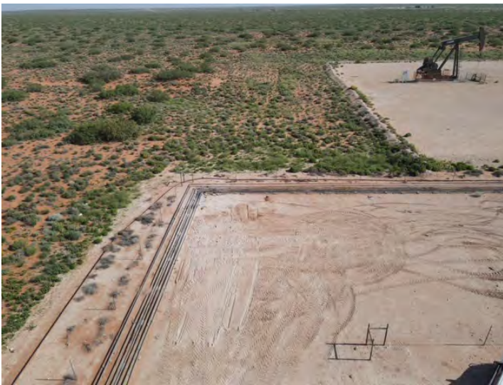
Aerial from south side
