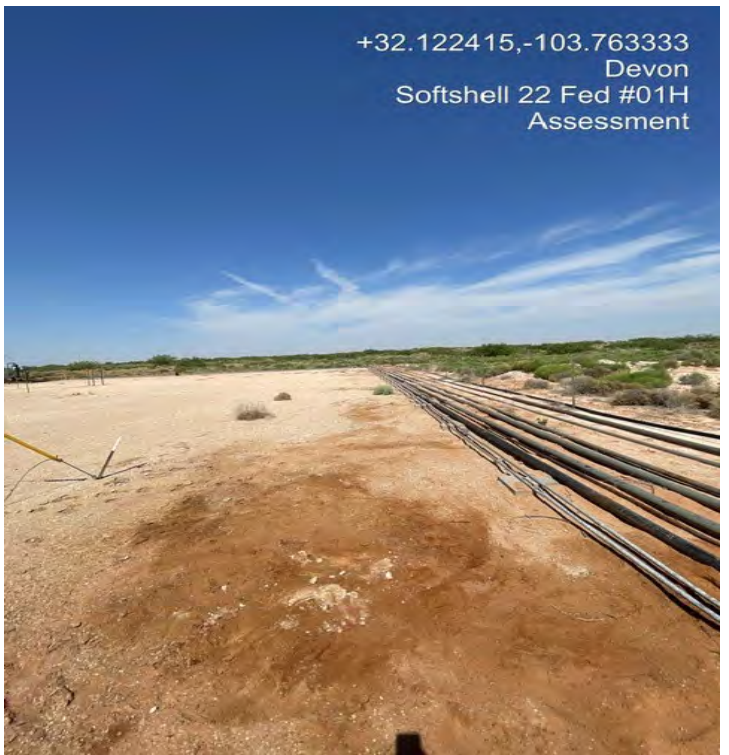
Northeast corner looking west
