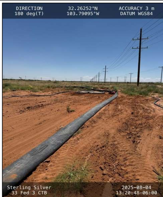
Photograph: 3 Date: 8/4/2025 Description: Reseeding activities View: South
