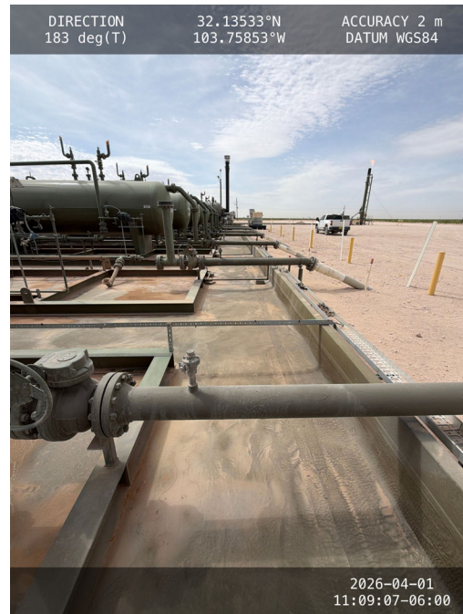
Photo 4 Photo of containment towards south.
