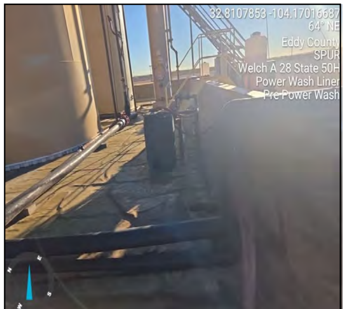
Photograph taken pre power-wash process facing northeast.
