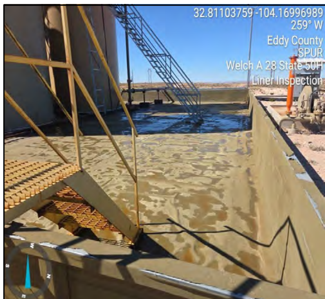
Photo of liner taken during liner inspection facing west.
