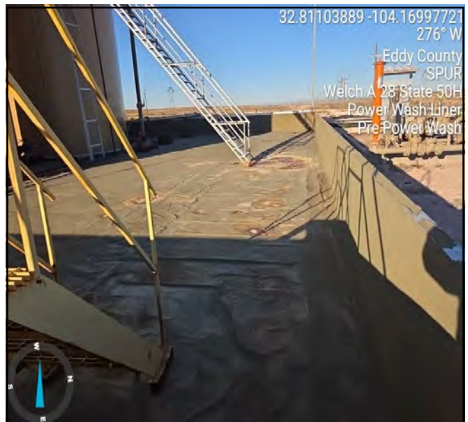
Photograph taken pre power-wash process facing west.
