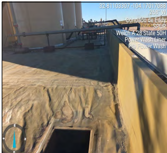
Photograph taken pre power-wash process facing west.
