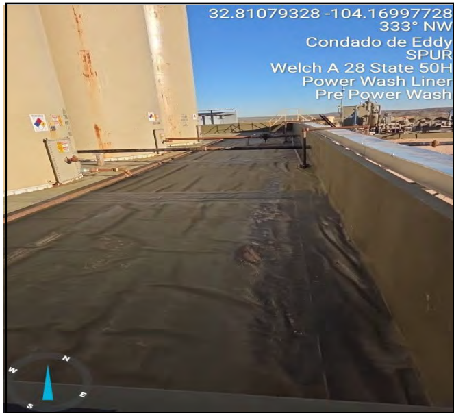
Photograph taken pre power-wash process facing northwest.
