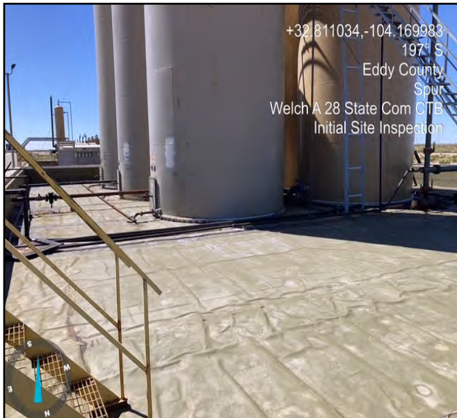
Photo of liner taken during initial liner inspection facing south.
