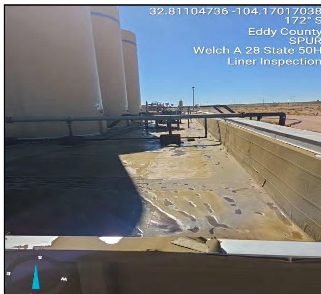
Photo of liner taken during liner inspection facing south.
