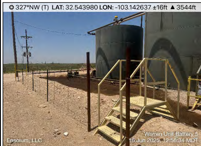
Photograph: 13 Date: 06/16/2025 Description: Initial release near SW06 View: Northwest
