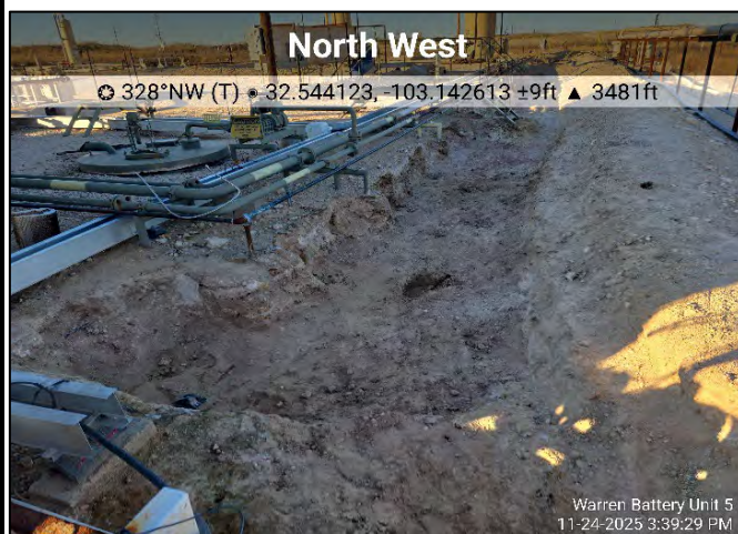
Photograph: 5 Date: 11/24/2025 Description: Excavation activities View: Northwest
