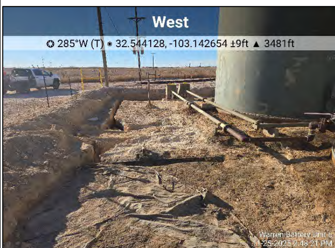
Photograph: 11 Date: 11/25/2025 Description: Excavation activities View: West
