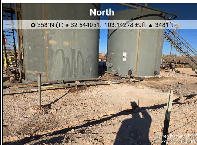
Photograph: 14 Date: 11/24/2025 Description: Excavation activities near SW06 View: North
