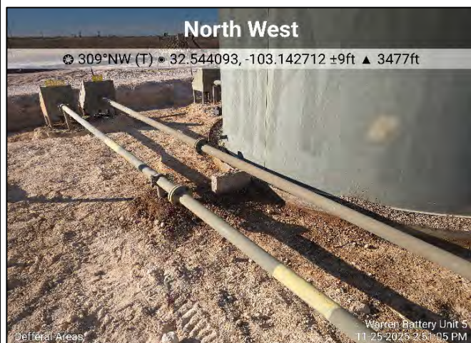
Photograph: 9 Date: 11/25/2025 Description: Excavation activities View: Northwest
