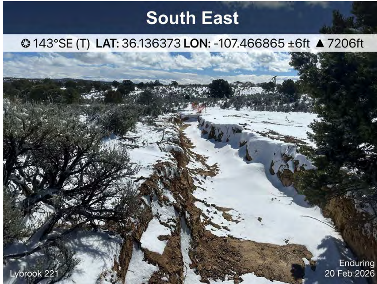
Photo #5 Excavation confirmation soil sampling 2/20/26.
