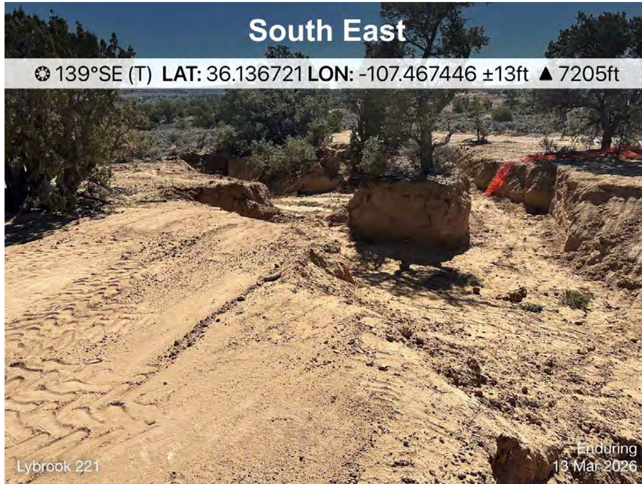
Photo #8 Additional excavation around SW30, confirmation sampling 3/13/26.
