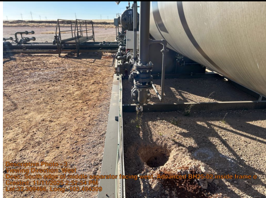
South edge of middle separator facing west. Advanced BH25-02 inside frame of middle separator.
