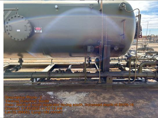
North of south separator facing south. Increased depth of BH25-10.
