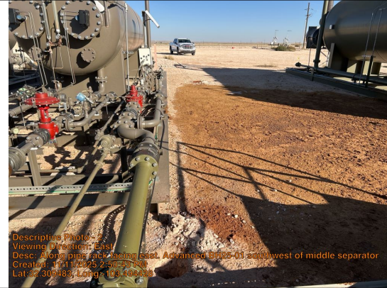
Along pipe rack facing east. Advanced BH25-01 southwest of middle separator.
