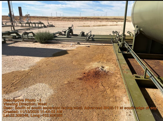
South of south separator facing west. Advanced BH25-11 at south edge of separator.
