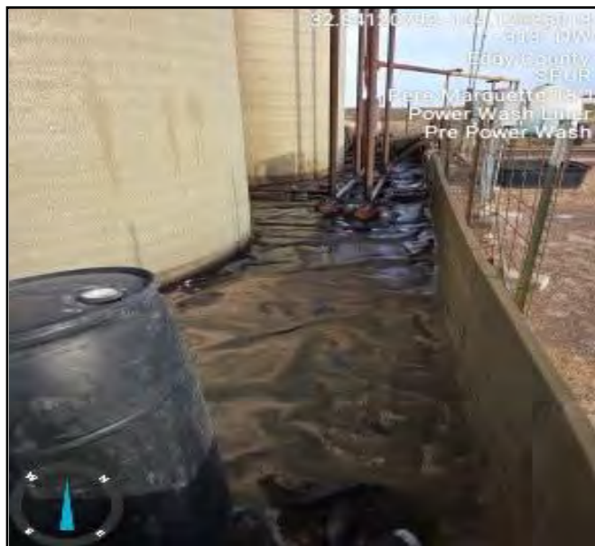
Photograph taken pre-powerwash facing northwest.
