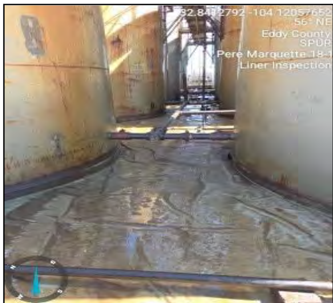
Photograph taken during liner inspection facing northeast.
