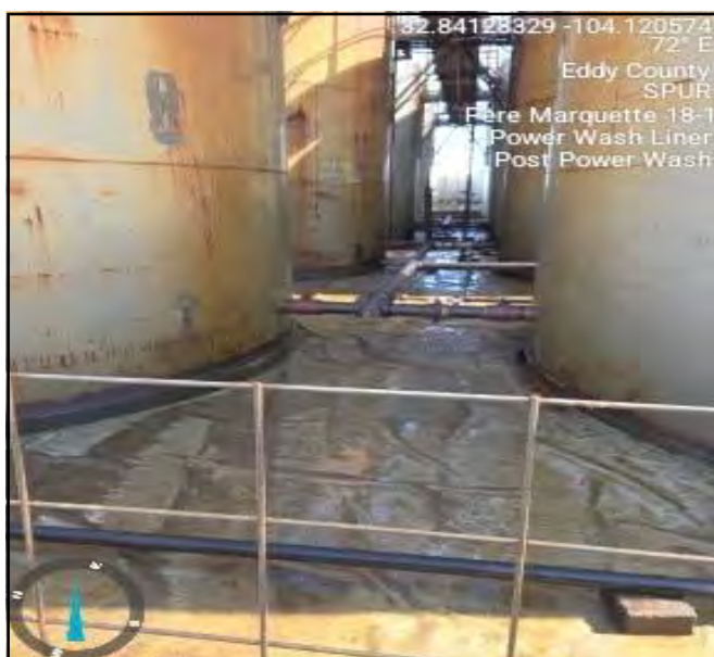
Photograph taken during liner inspection facing east.
