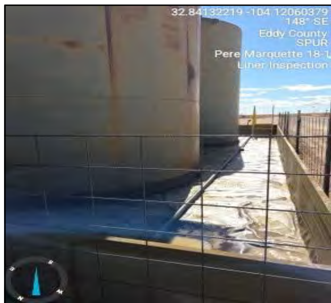
Photograph taken during liner inspection facing southeast.
