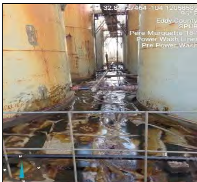
Photograph taken pre-powerwash facing east.
