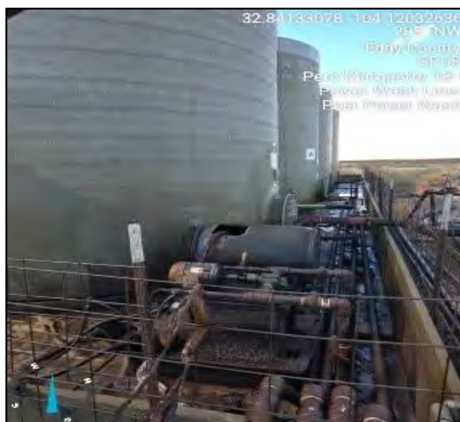
Photograph taken during liner inspection facing northwest.
