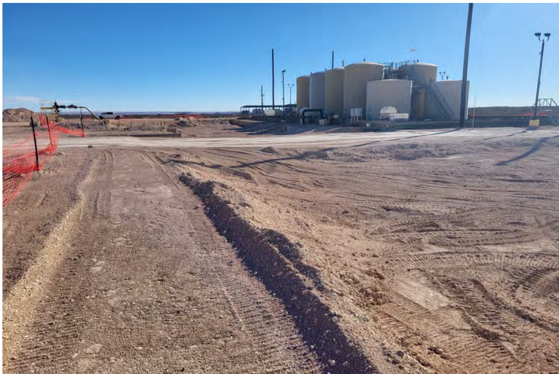
West side of project site 275' long, 85' wide, and 1.5' to 2.0' deep
