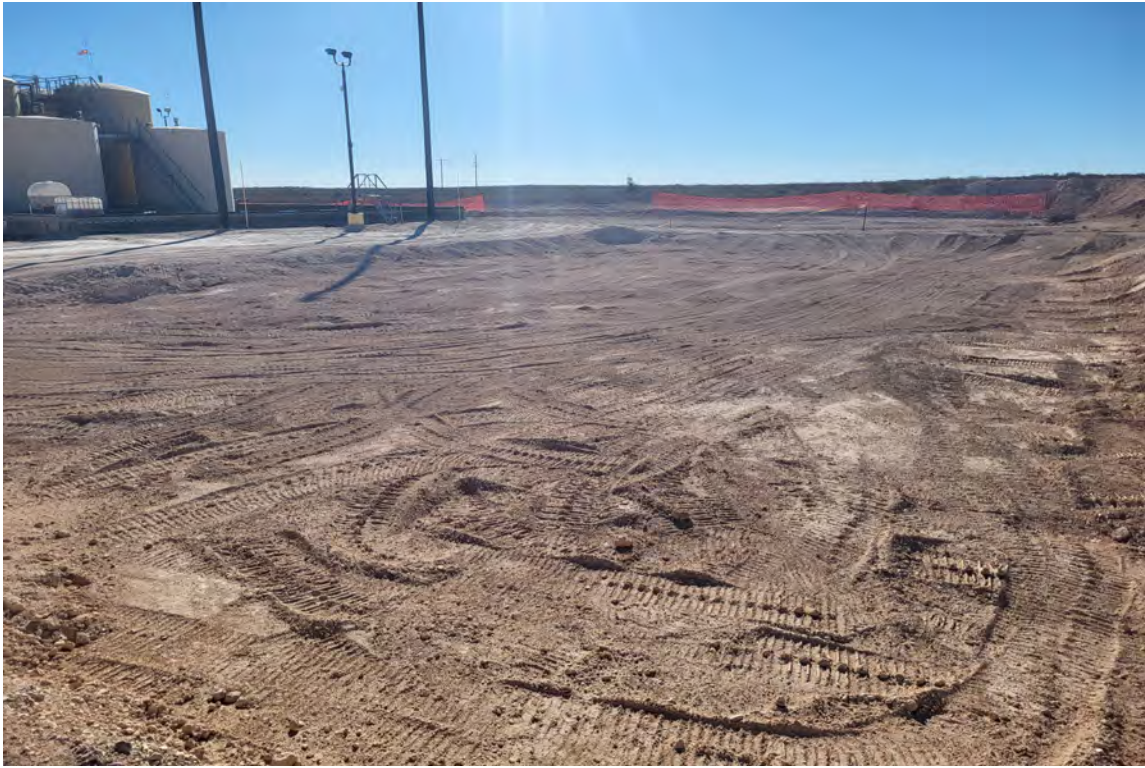
West side of the project site approximately 220' long, 75' wide 1.5' to 2.0' deep
