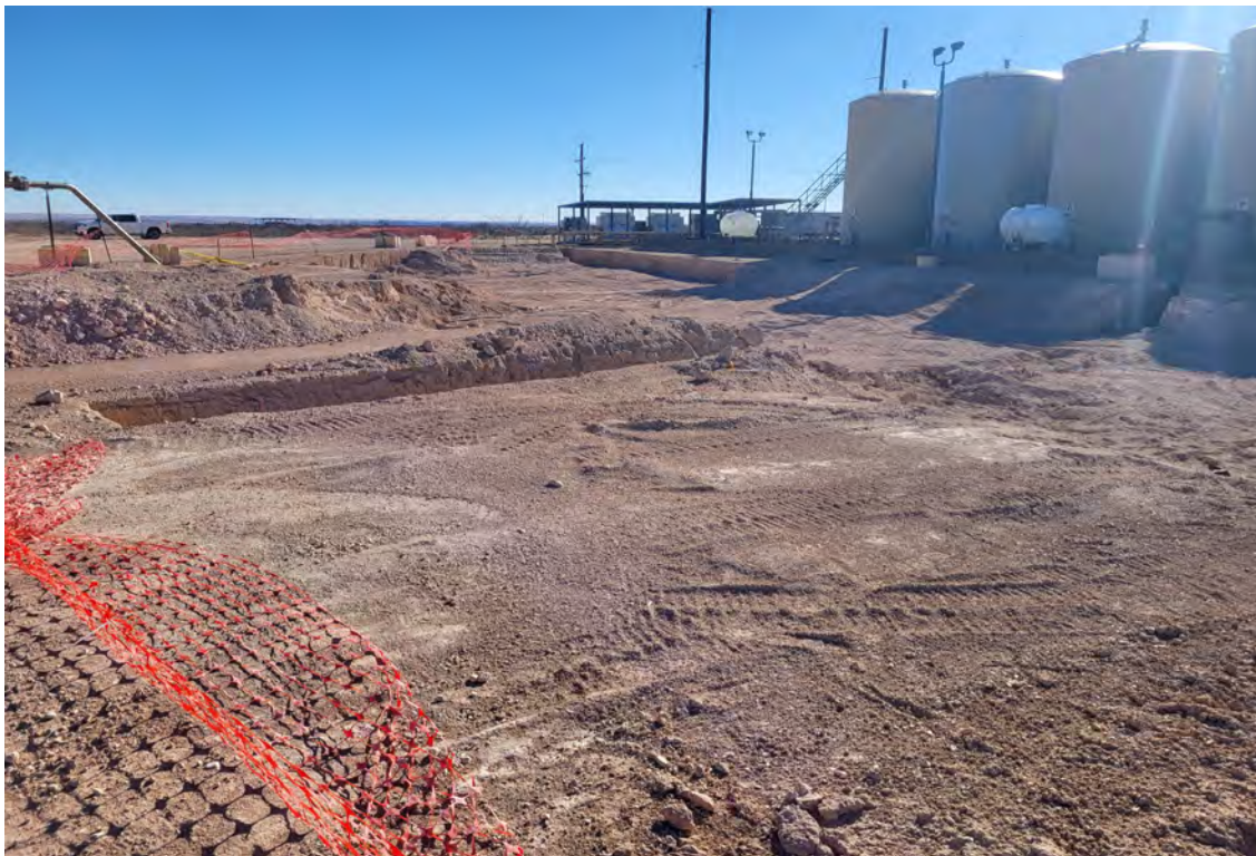
North side of project site approximately 50' wide, 220' long and 1.5' to 2.0' deep
