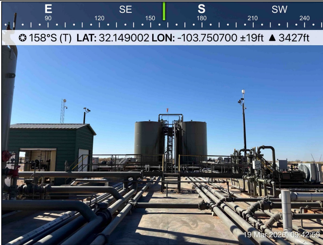
PHOTO 11: Southeastern view during liner inspection activities. 3/19/2026
