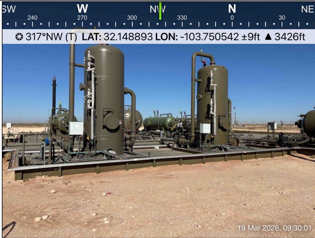
PHOTO 5: Northwestern view outside of containment during liner inspection activities. 3/19/2026
