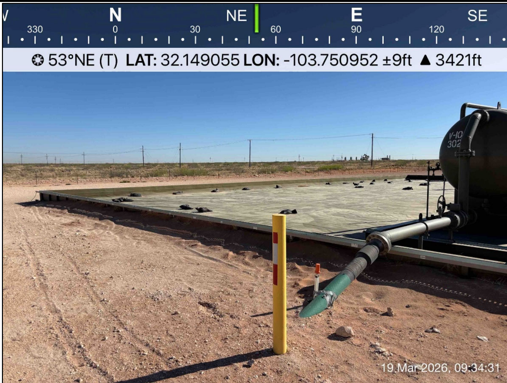
PHOTO 10: Northeastern view outside of containment during liner inspection activities. 3/19/2026
