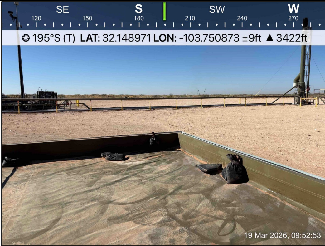
PHOTO 25: Southwestern view during liner inspection activities. 3/19/2026
