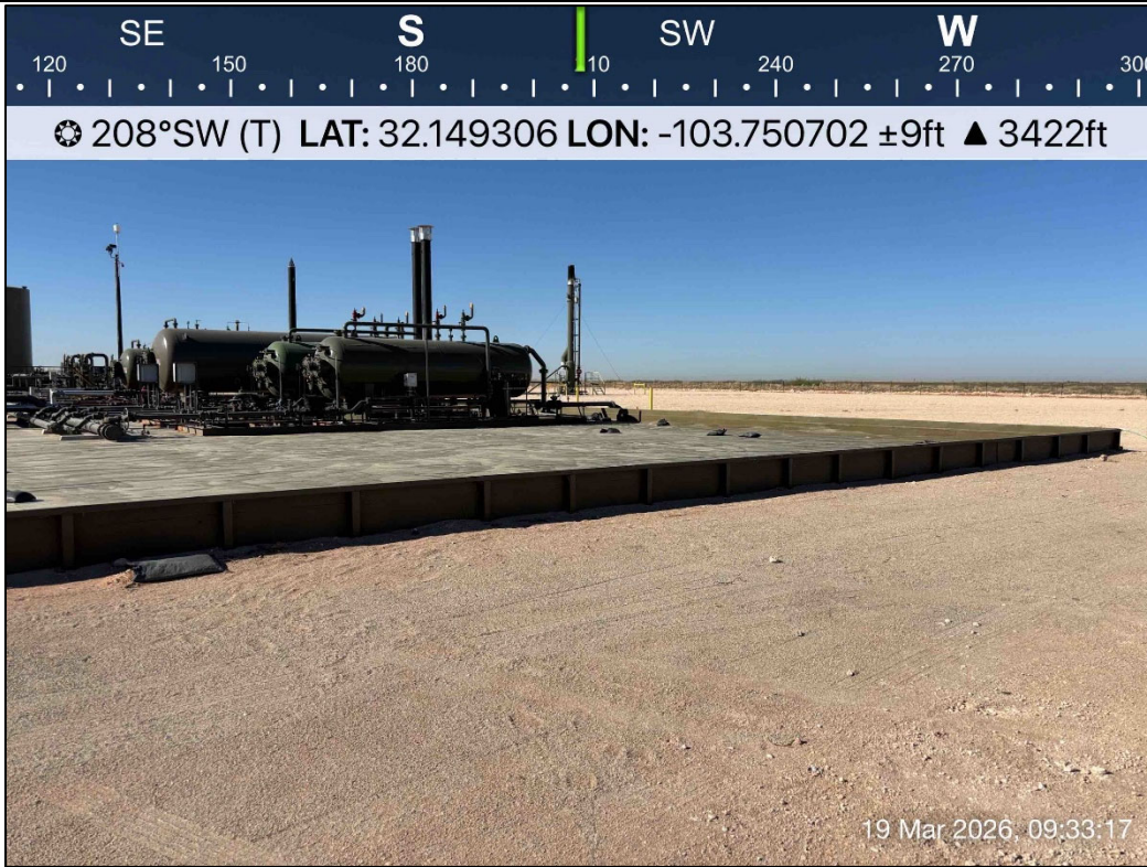
PHOTO 9: Southwestern view outside of containment during liner inspection activities. 3/19/2026
