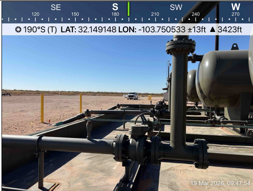
PHOTO 17: Southern view during liner inspection activities. 3/19/2026
