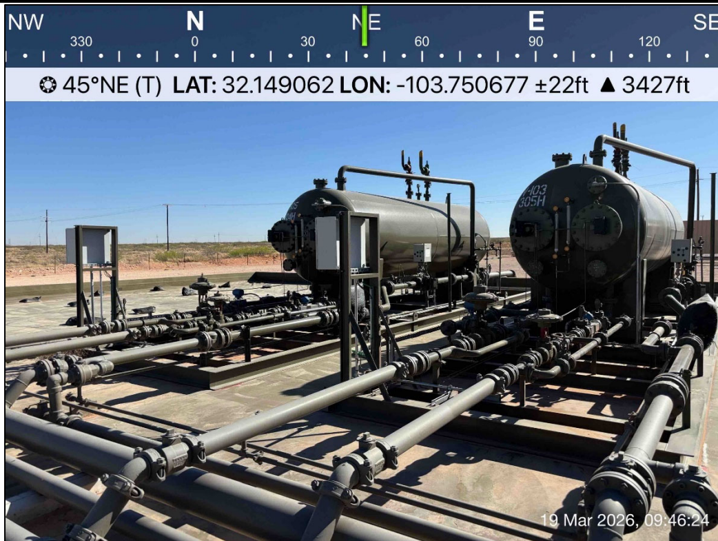
PHOTO 16: Northeastern view during liner inspection activities. 3/19/2026
