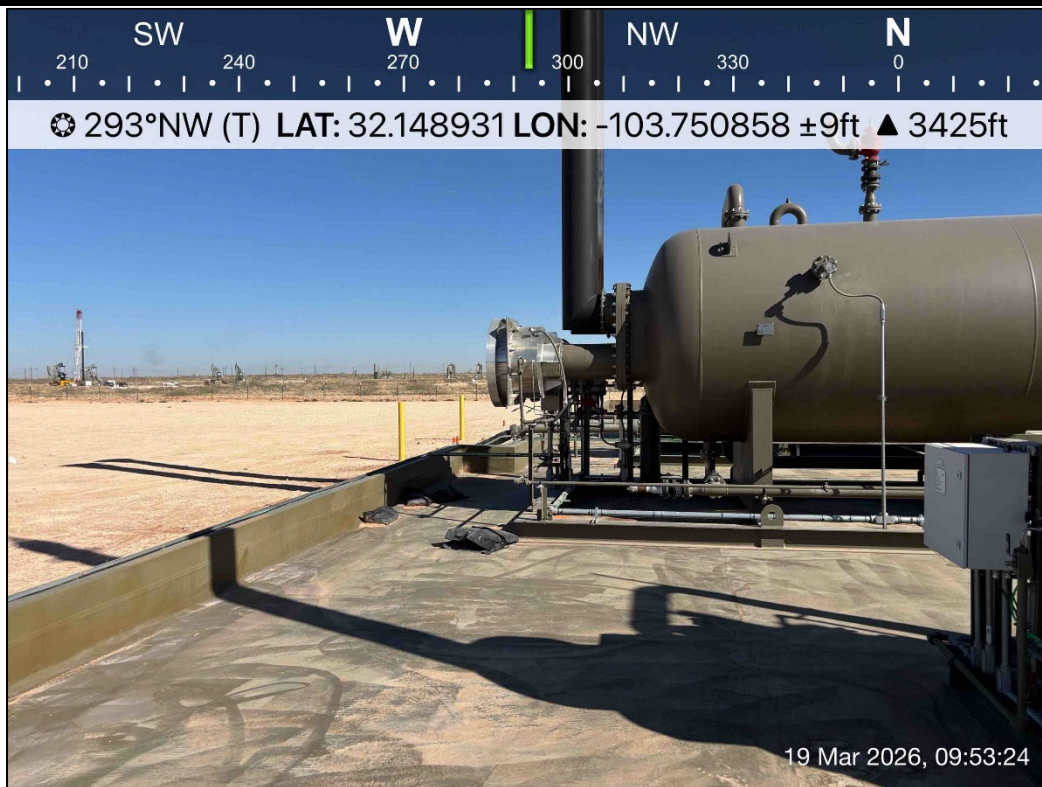
PHOTO 26: Northwestern view during liner inspection activities. 3/19/2026
