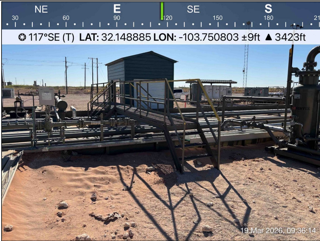
PHOTO 13: Southeastern view outside of containment during liner inspection activities. 3/19/2026
