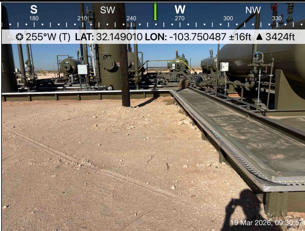
PHOTO 6: Southwestern view outside of containment during liner inspection activities. 3/19/2026
