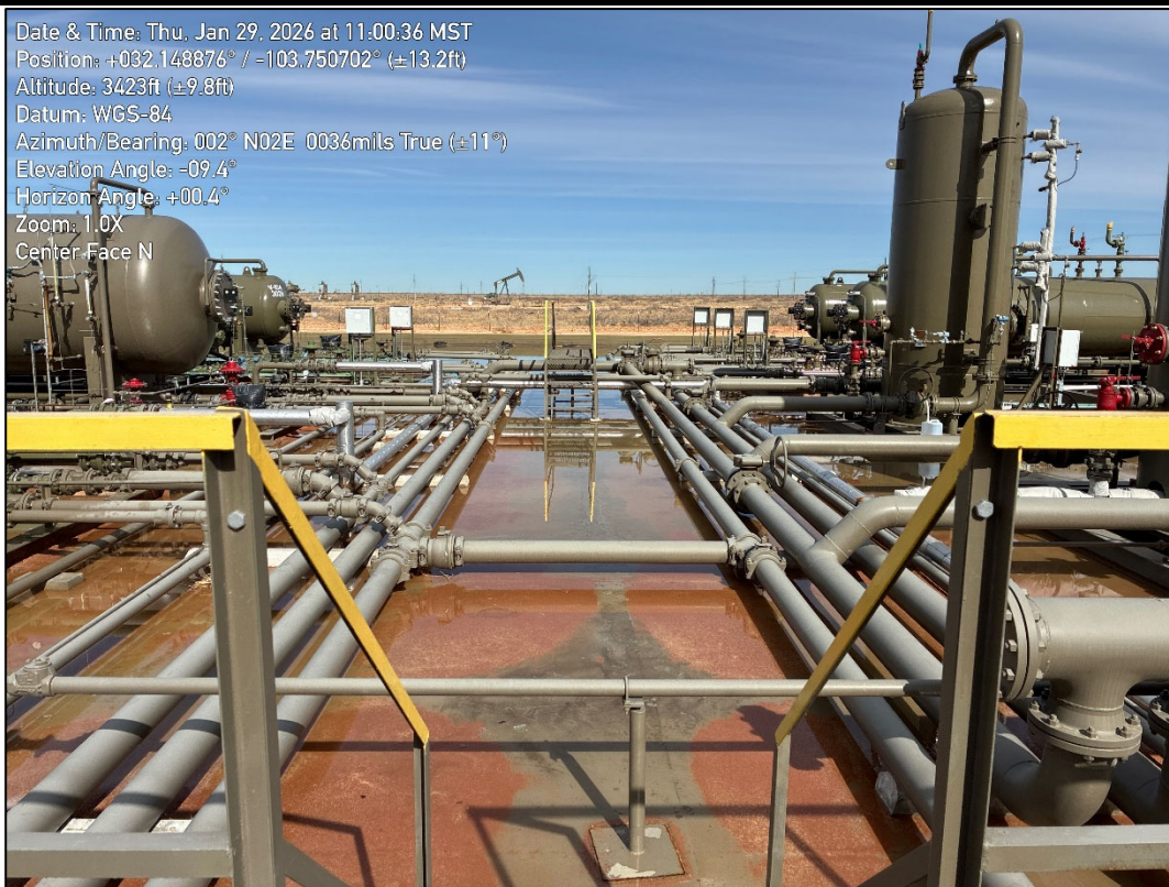
PHOTO 2: Northeastern view during initial site assessment. 1/29/2026
