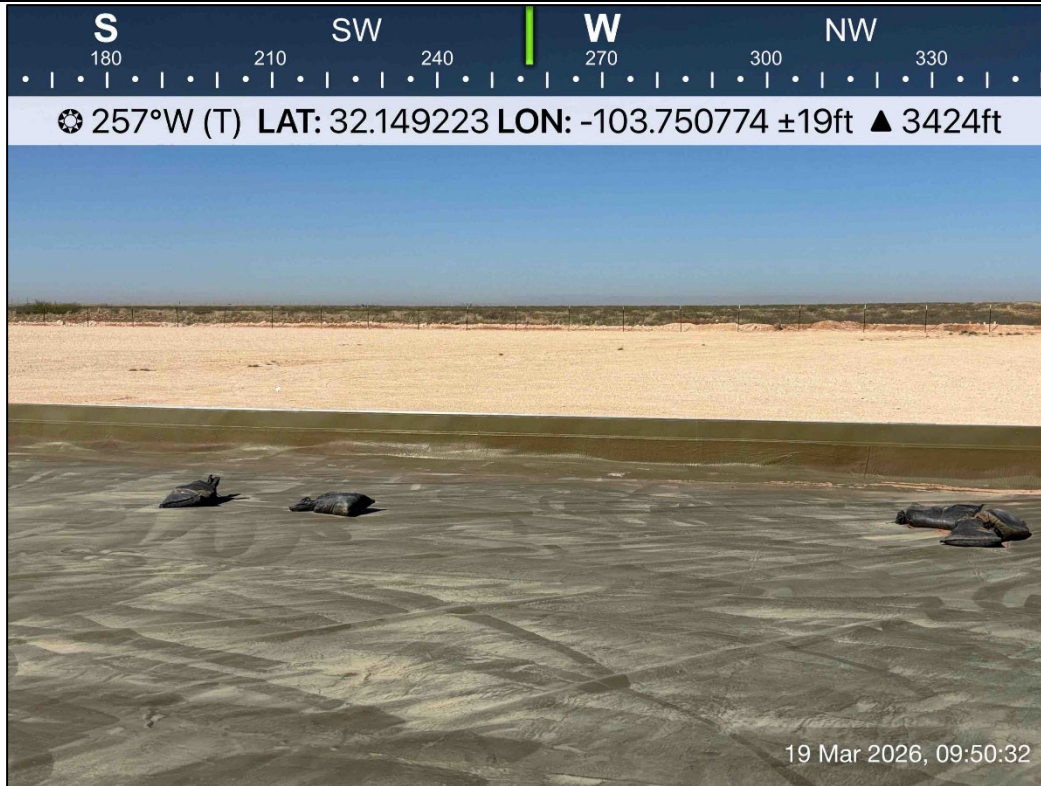
PHOTO 21: Southwestern view during liner inspection activities. 3/19/2026
