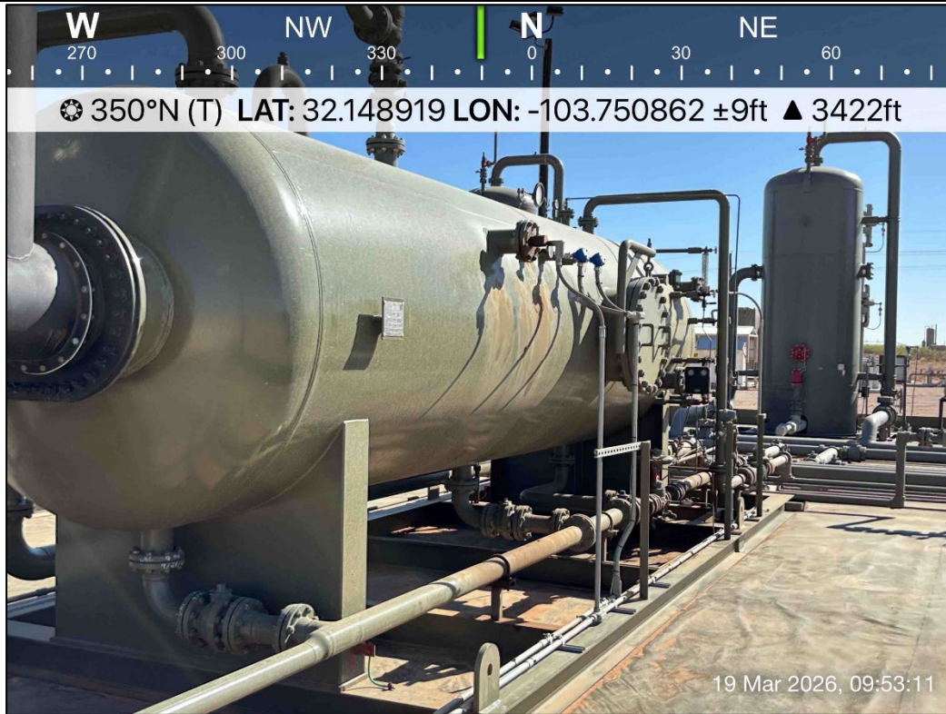
PHOTO 27: Northwestern view during liner inspection activities. 3/19/2026
