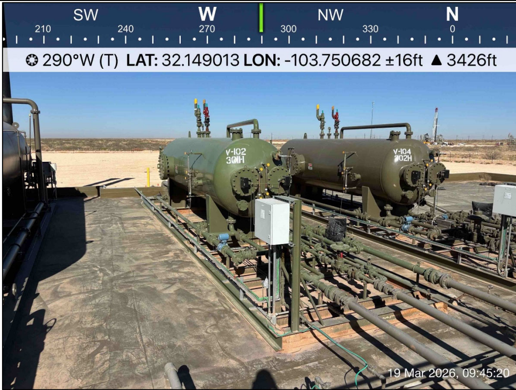
PHOTO 15: Northwestern view during liner inspection activities. 3/19/2026
