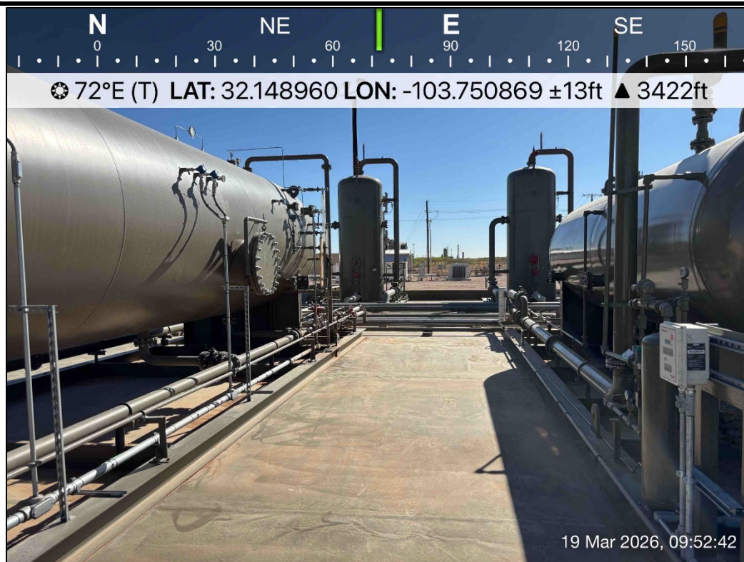
PHOTO 24: Northeastern view during liner inspection activities. 3/19/2026
