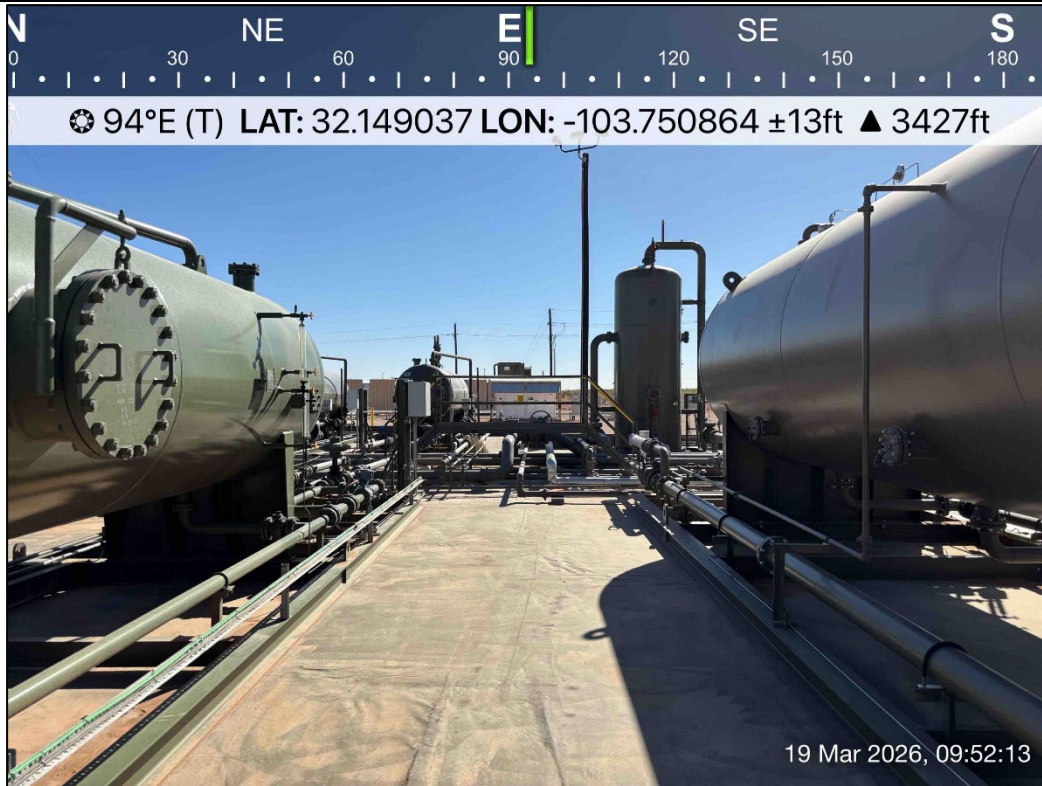
PHOTO 23: Eastern view during liner inspection activities. 3/19/2026
