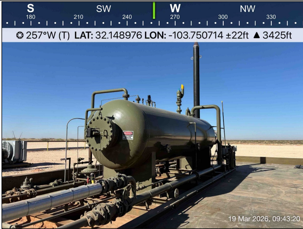
PHOTO 13: Southwestern view during liner inspection activities. 3/19/2026
