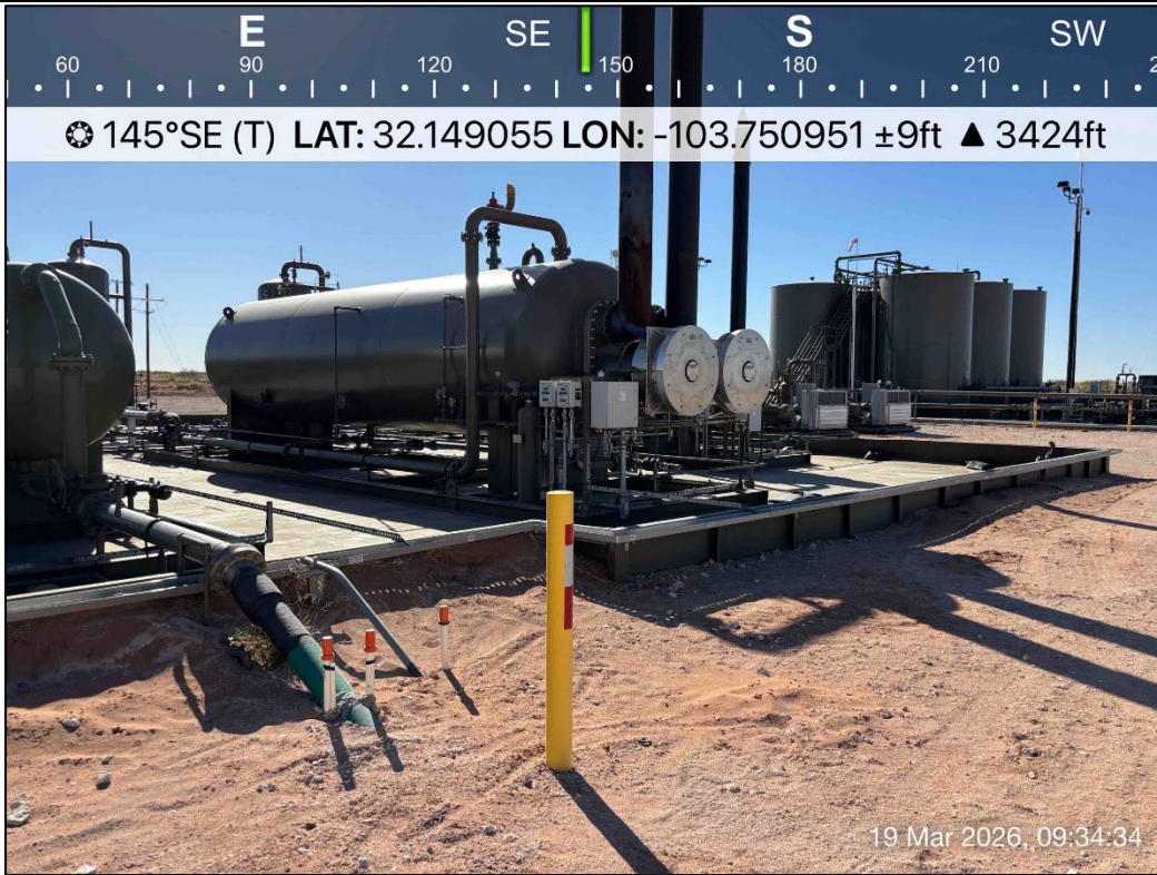
PHOTO 11: Southeastern view outside of containment during liner inspection activities. 3/19/2026
