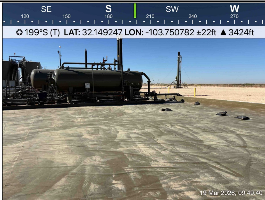
PHOTO 20: Southwestern view during liner inspection activities. 3/19/2026
