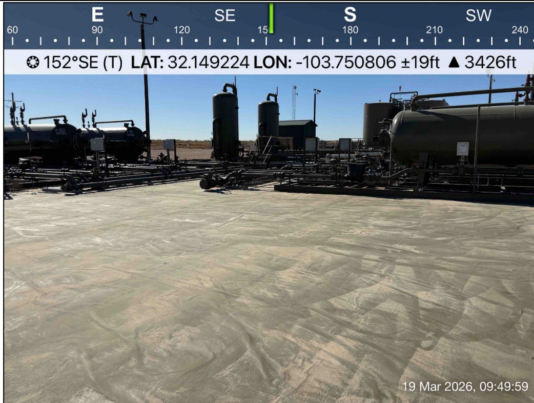
PHOTO 19: Southeastern view during liner inspection activities. 3/19/2026
