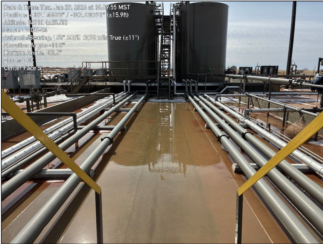
PHOTO 1: Southeastern view during initial site assessment. 1/29/2026
