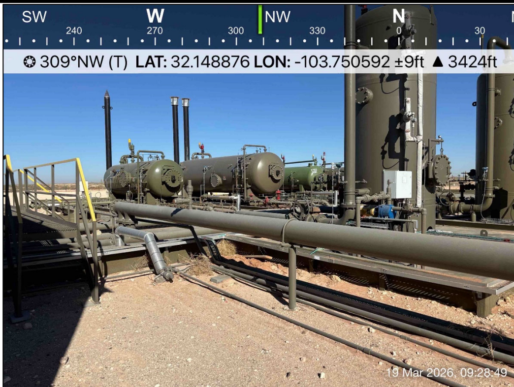
PHOTO 4: Northwestern view outside of containment during liner inspection activities. 3/19/2026
