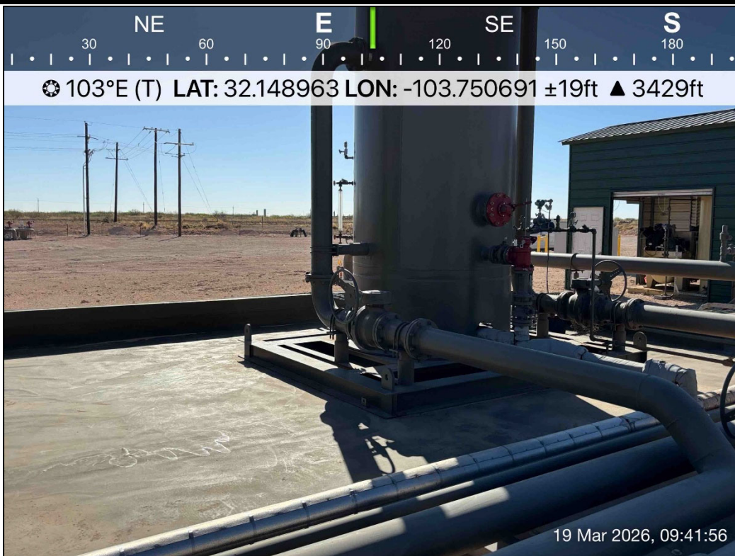
PHOTO 12: Southeastern view during liner inspection activities. 3/19/2026
