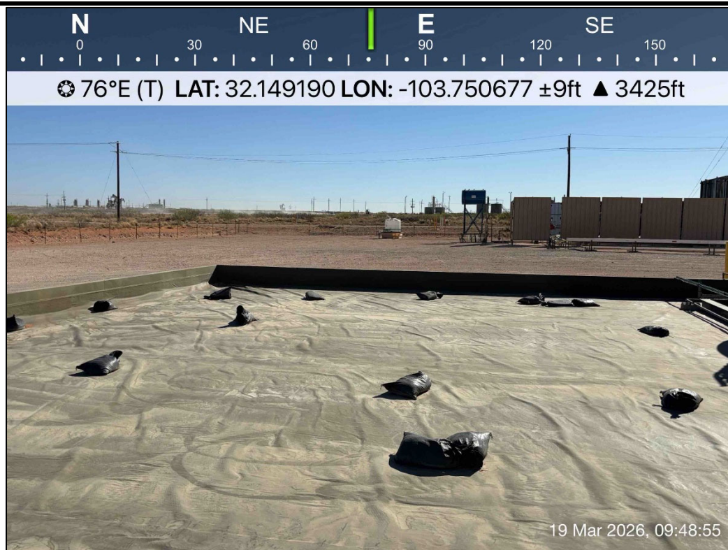
PHOTO 18: Northeastern view during liner inspection activities. 3/19/2026
