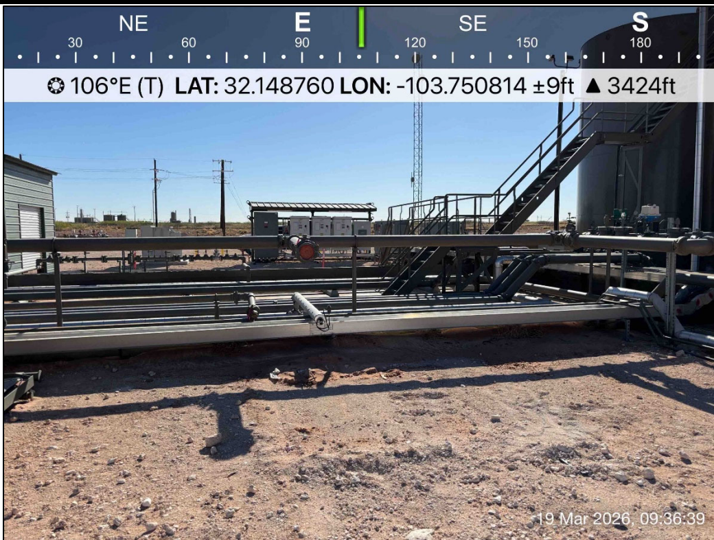
PHOTO 14: Southeastern view outside of containment during liner inspection activities. 3/19/2026
