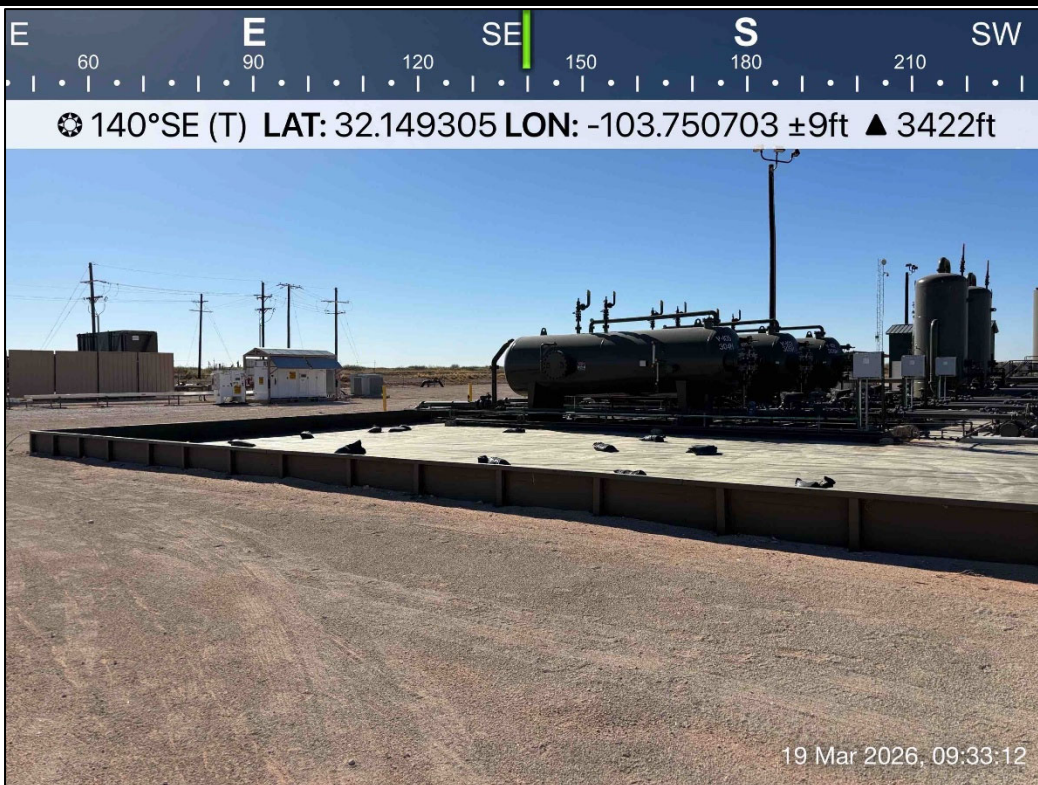
PHOTO 8: Southeastern view outside of containment during liner inspection activities. 3/19/2026
