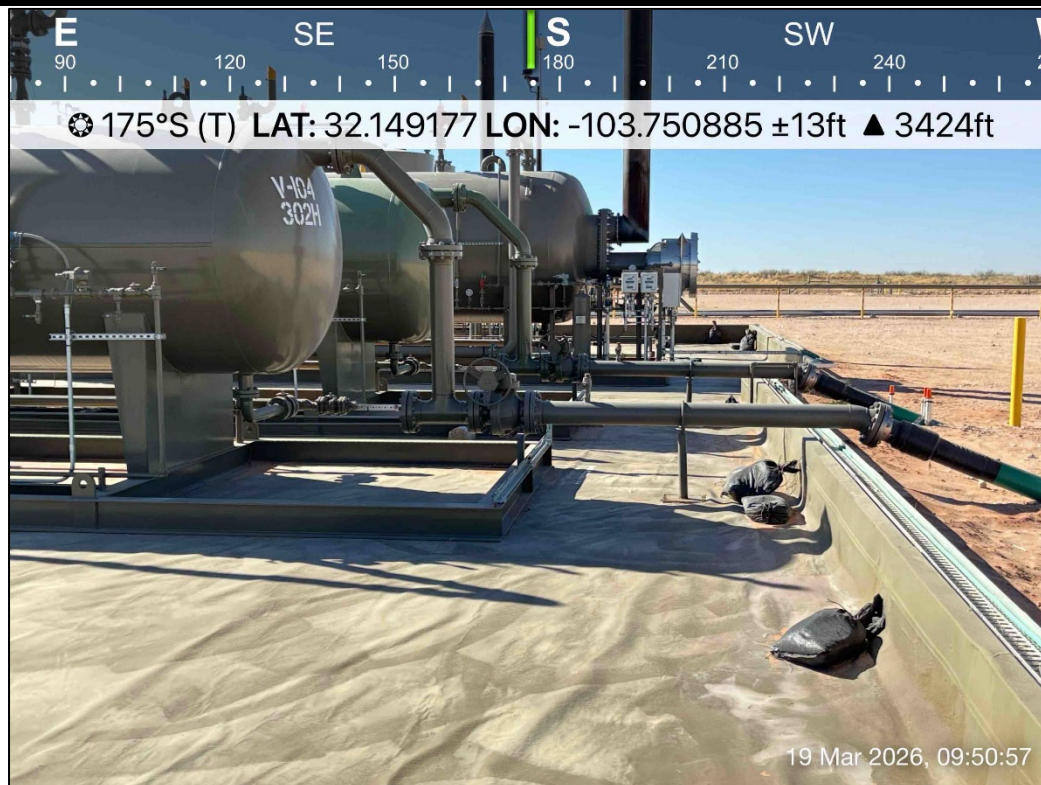
PHOTO 22: Southern view during liner inspection activities. 3/19/2026
