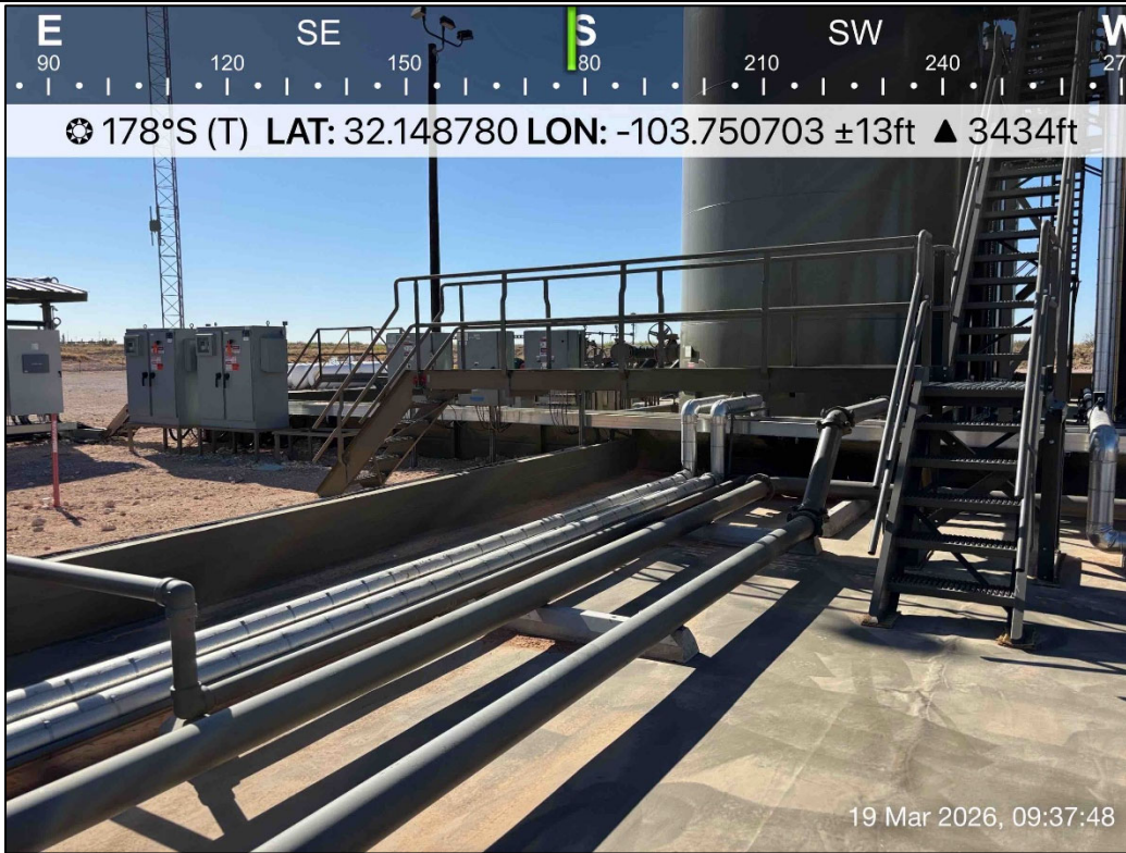
PHOTO 9: Southern view during liner inspection activities. 3/19/2026
