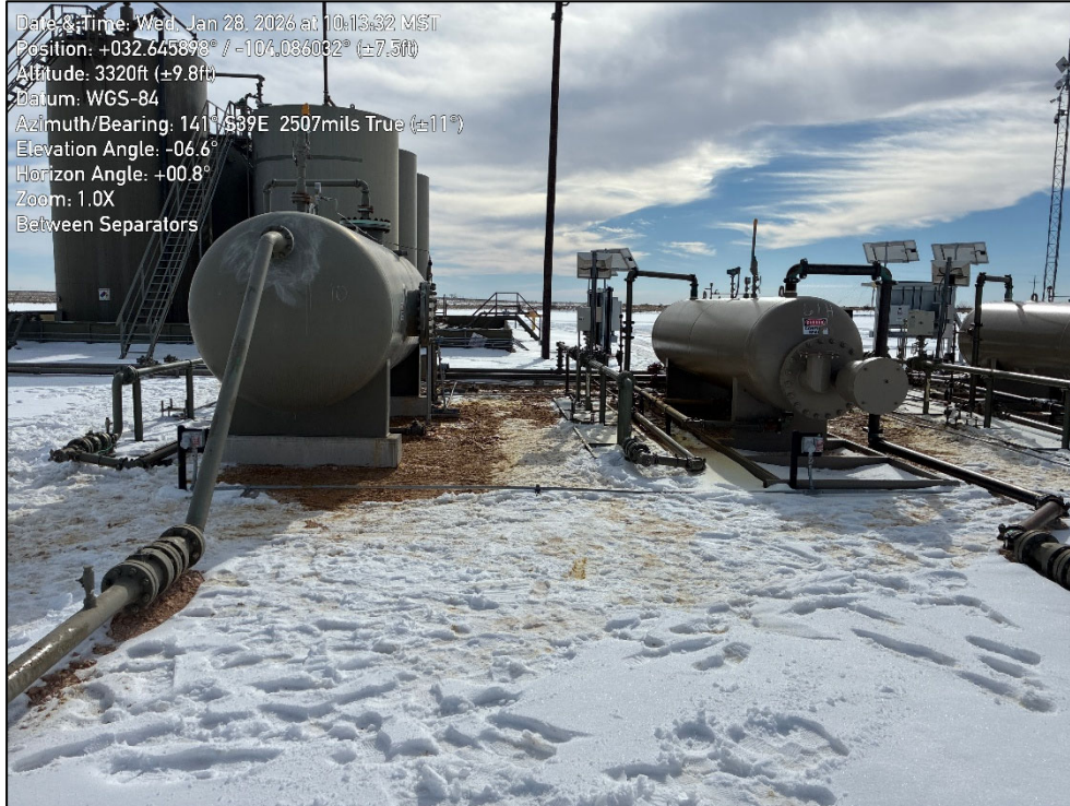
PHOTO 3: Southeastern view during initial site assessment activities. 1/28/2026
