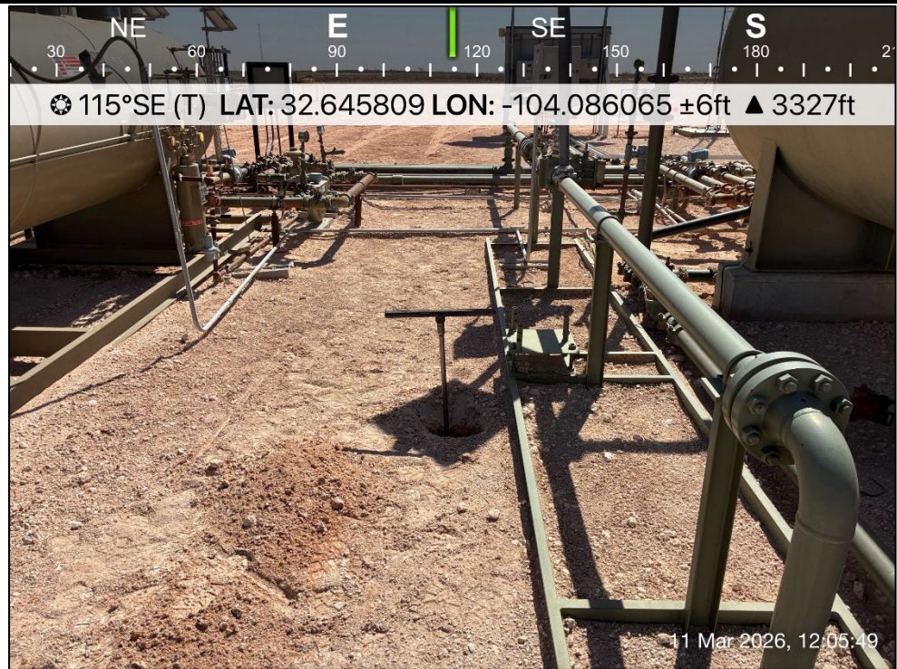
PHOTO 8: Southeastern view during delineation activities. 3/11/2026
