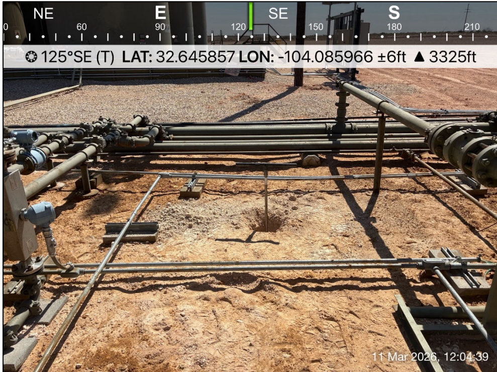
PHOTO 5: Southeastern view during delineation activities. 3/11/2026
