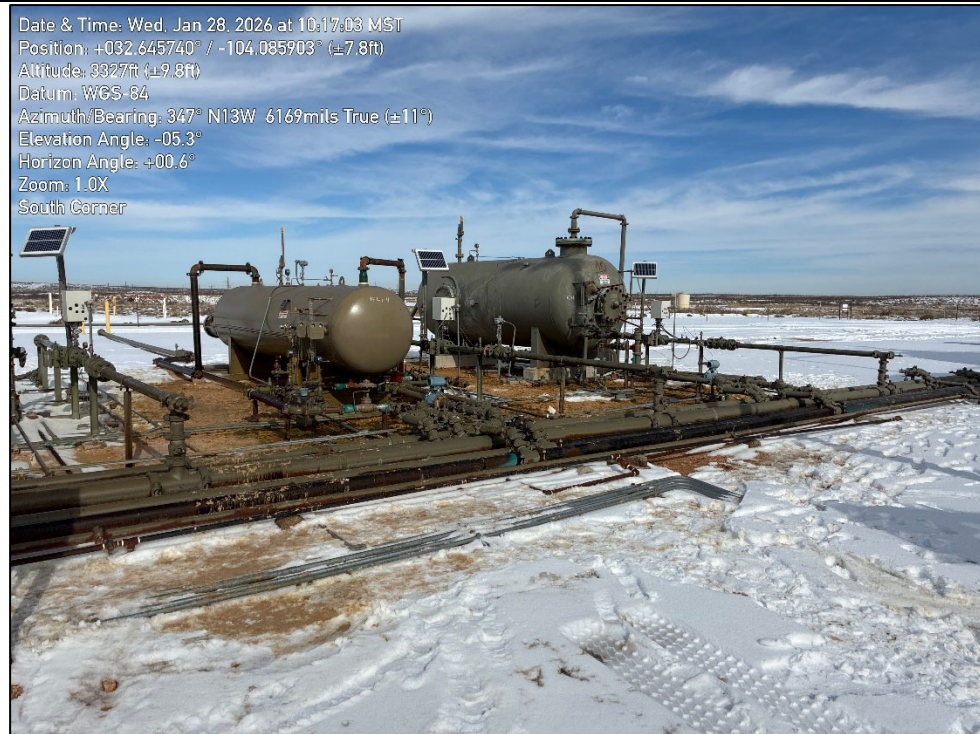
PHOTO 4: Northwestern view during initial site assessment activities. 1/28/2026
