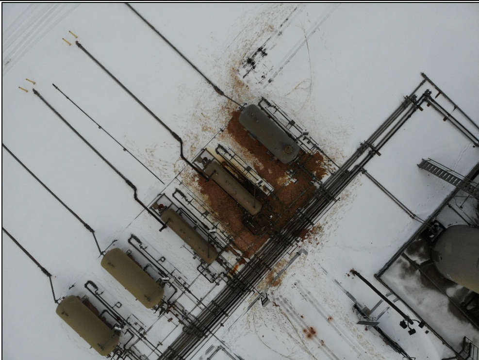
PHOTO 2: Northern aerial view during initial site assessment activities. 1/28/2026
