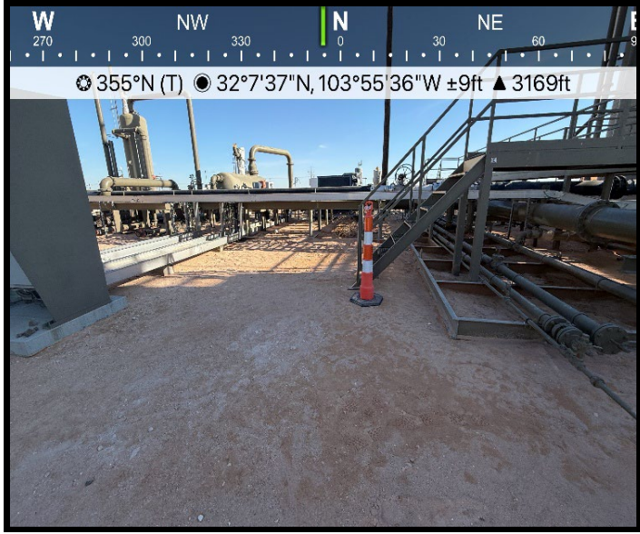
View of Area of Concern
