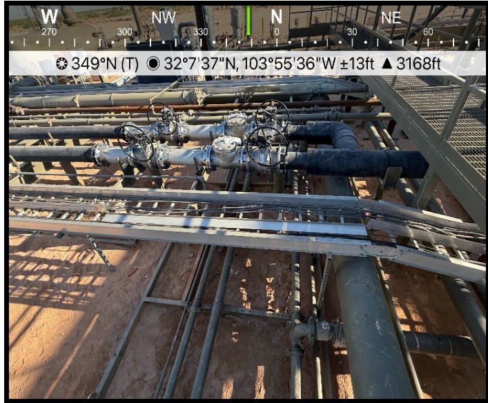
View of Area of Concern
