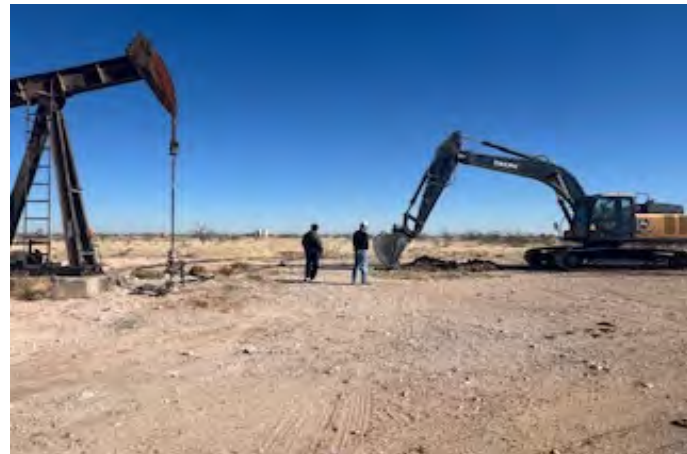
View to N of TH-1 installation.
