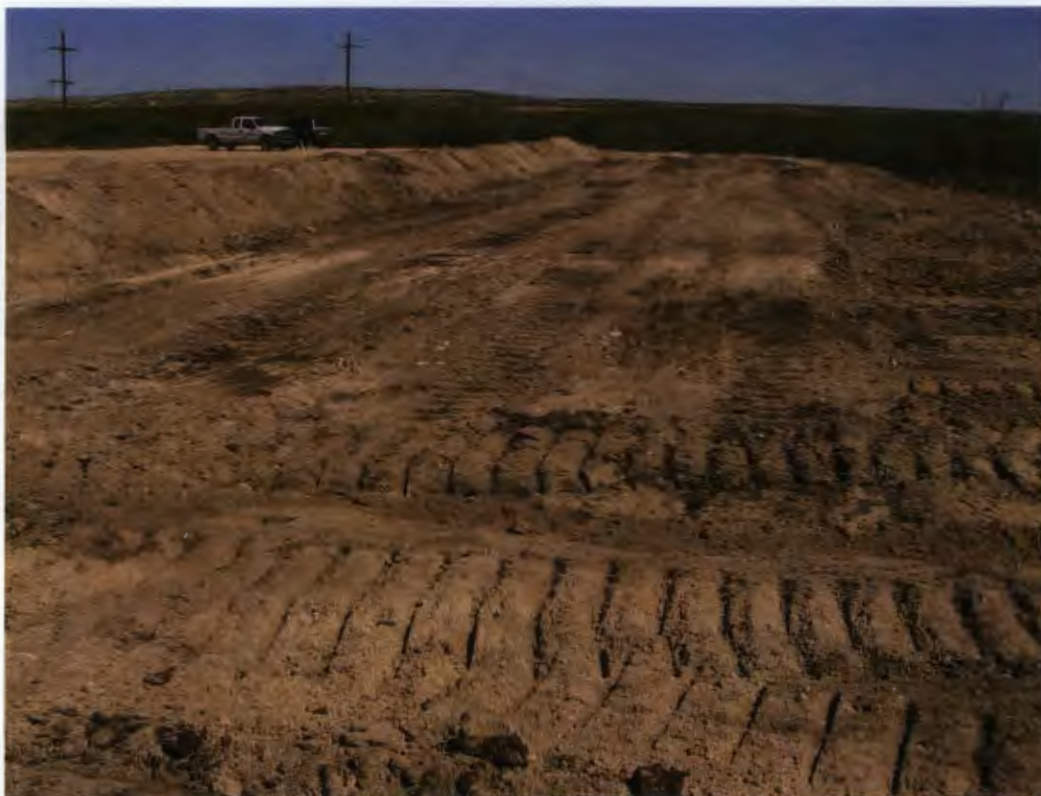
Figure 4: Western 1/3 of caliche pad removed and ready for ripping and seeding. Portions of the caliche pad were included in BLM interim reclamation activities.
