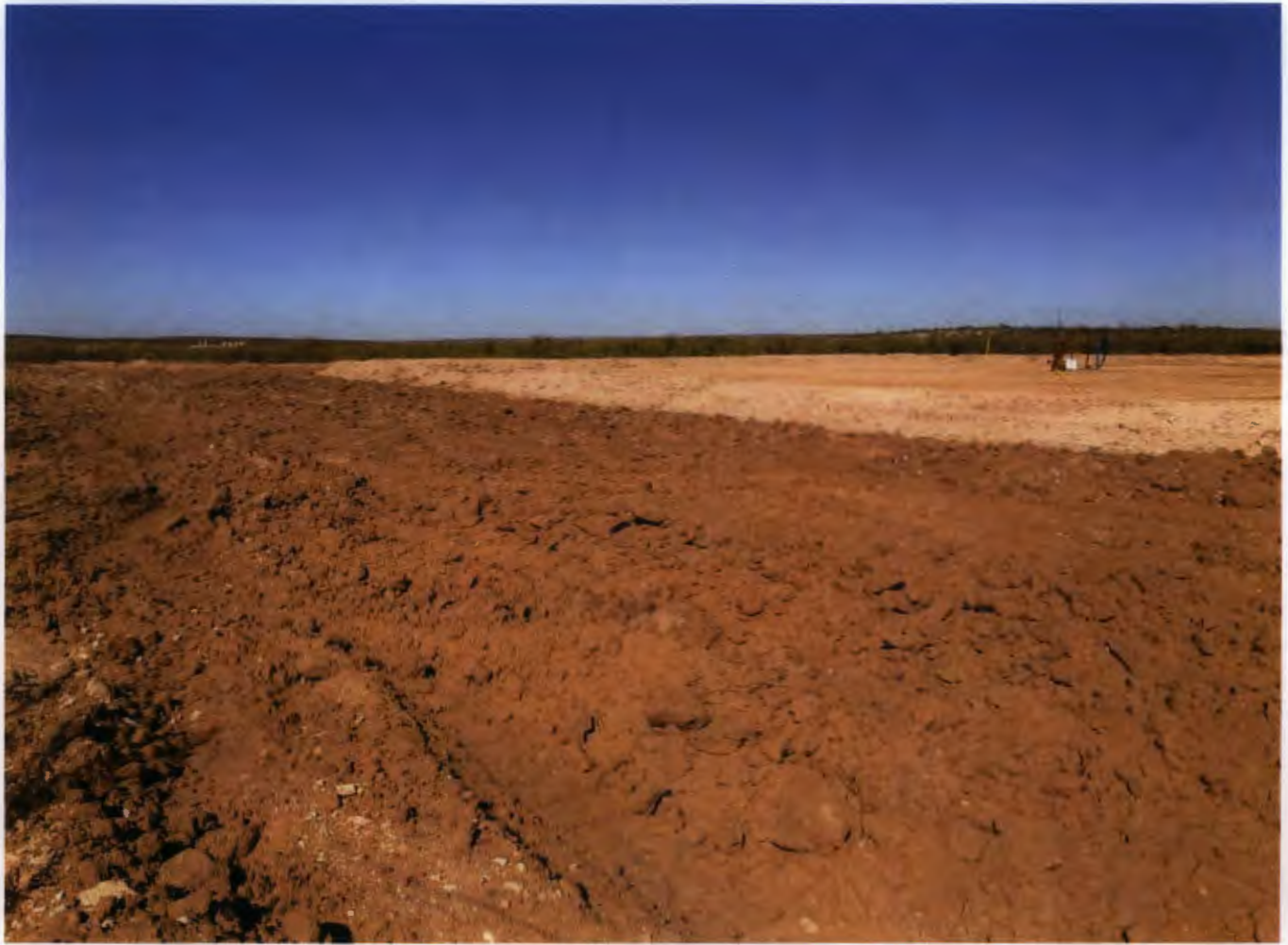
Figure 5: Photo of remediated western 1/3 of caliche pad, viewing north. Area was ripped and seeded with BLM seed mixture #4 and Alkali Sacaton.
