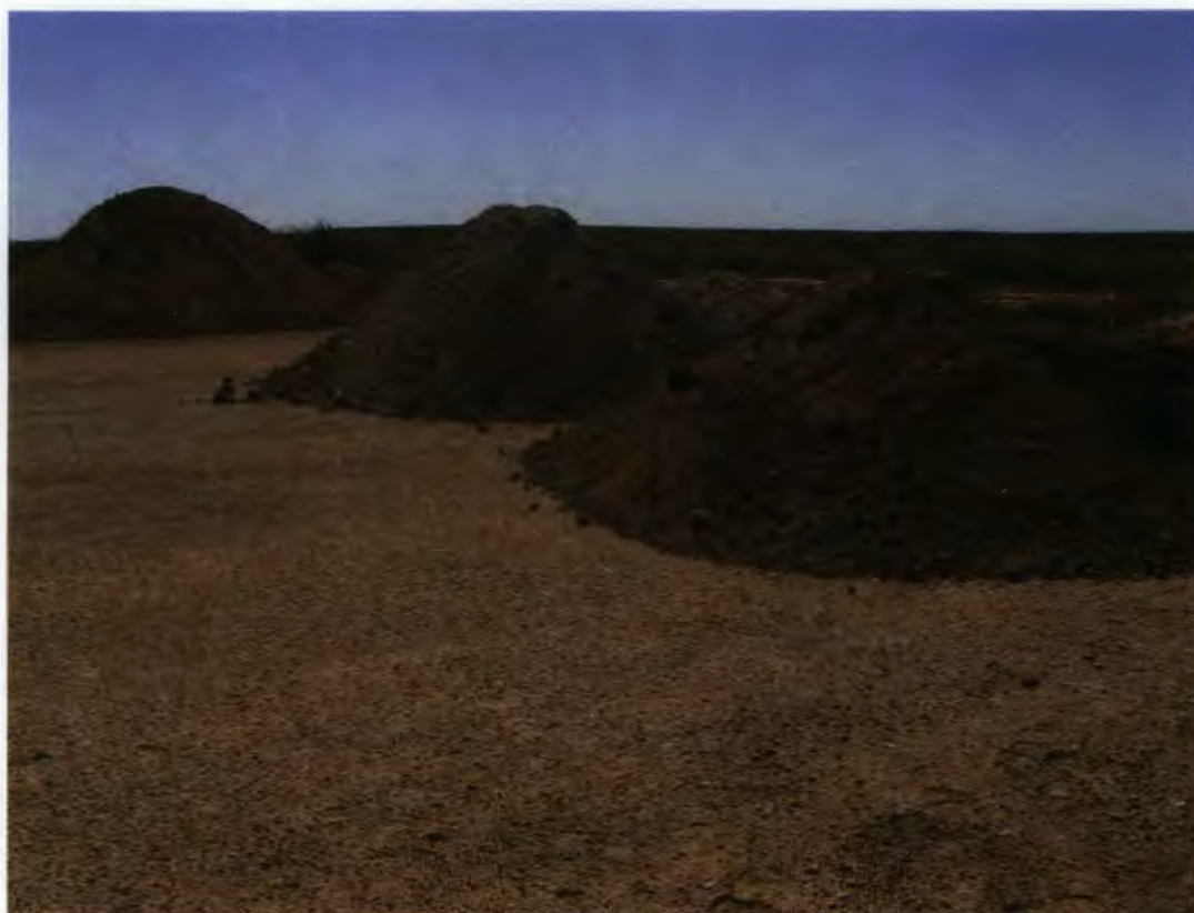
Figure 2: Stockpiled impacted caliche (two right soil piles) waiting transport to R360. The far left soil pile (background) is clean soil to be used for BLM interim reclamation activities.
