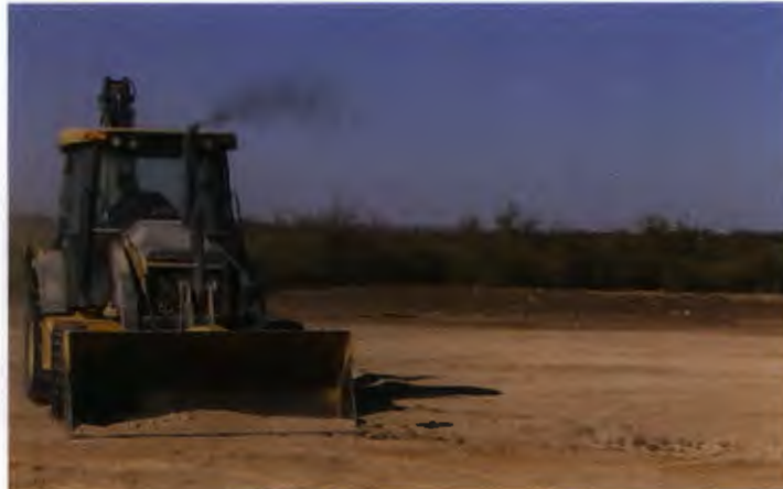
Figure 2: Backfilling a "Y" shaped trench with caliche.
