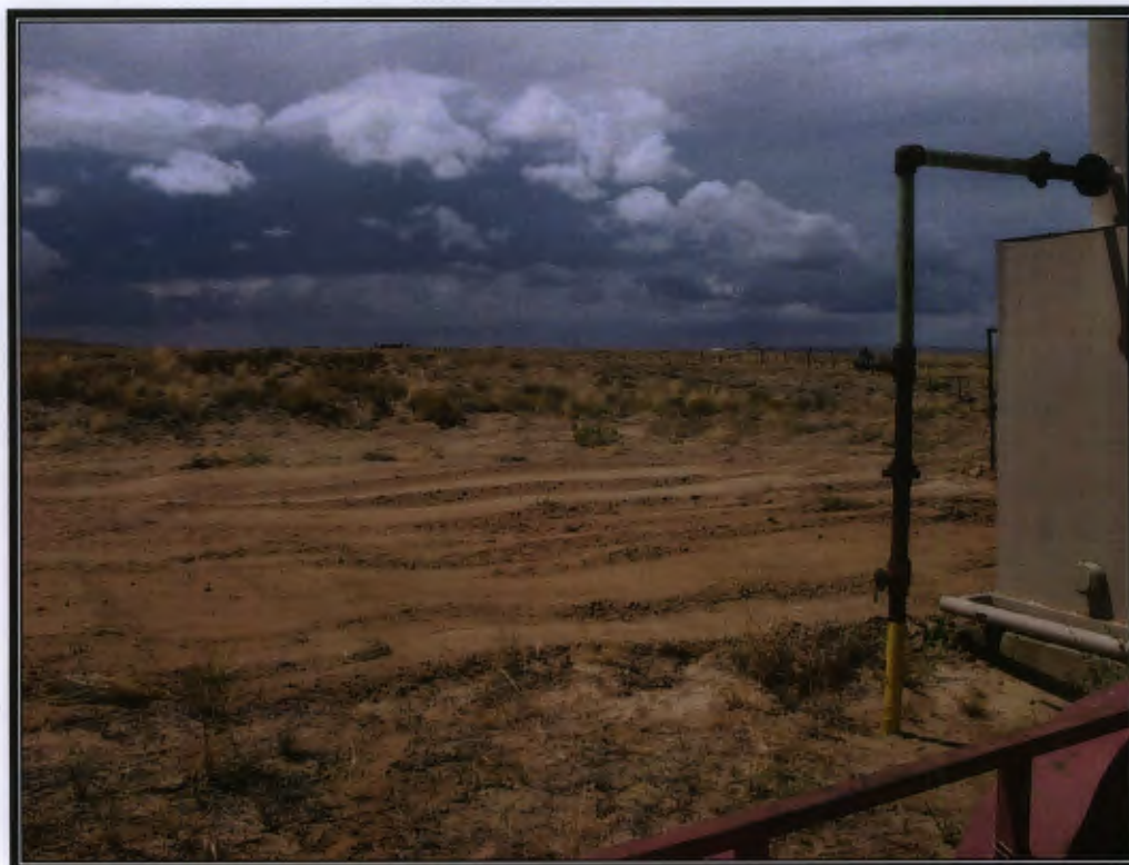
Photo 2: Excavated Area After Backfilling and Recontouring
