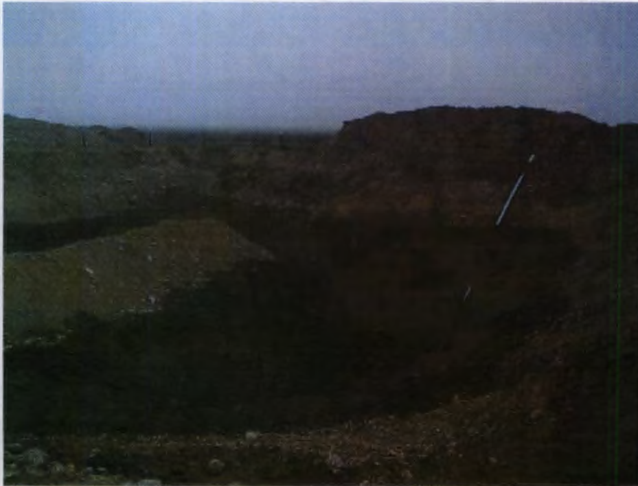
Figure B-3: Condition of pit excavation after installation of permeable layer above secondary liner. Leak detection riser pipe in background.
