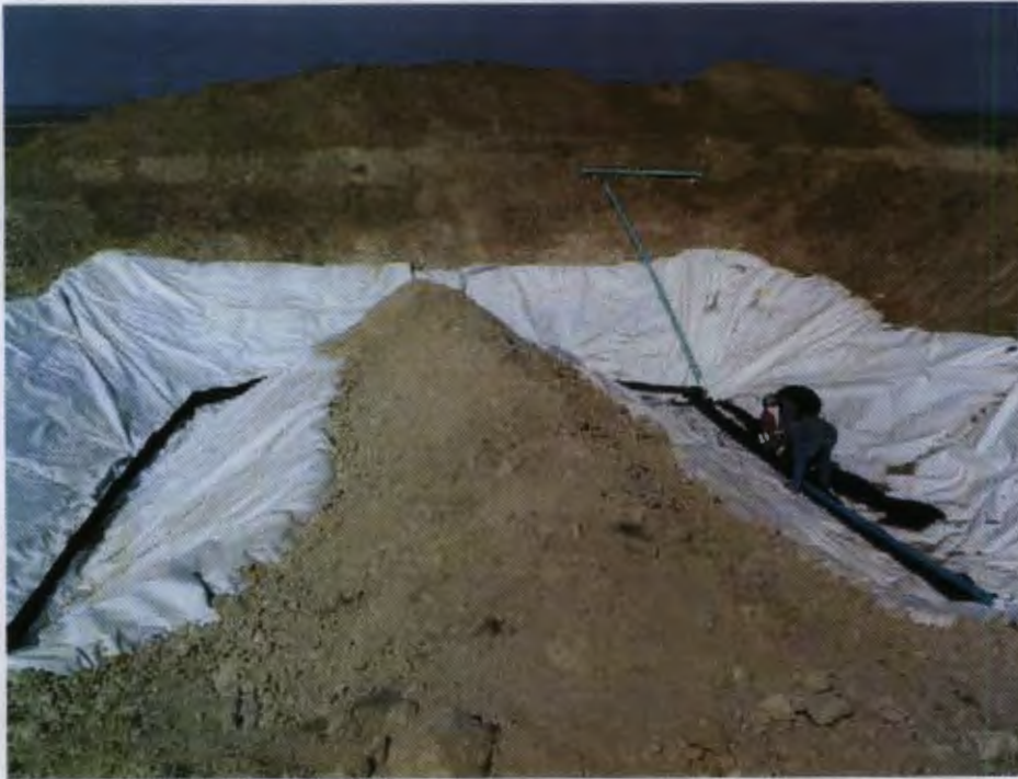
Figure B-1 – Installation of secondary liner and leak detection system
