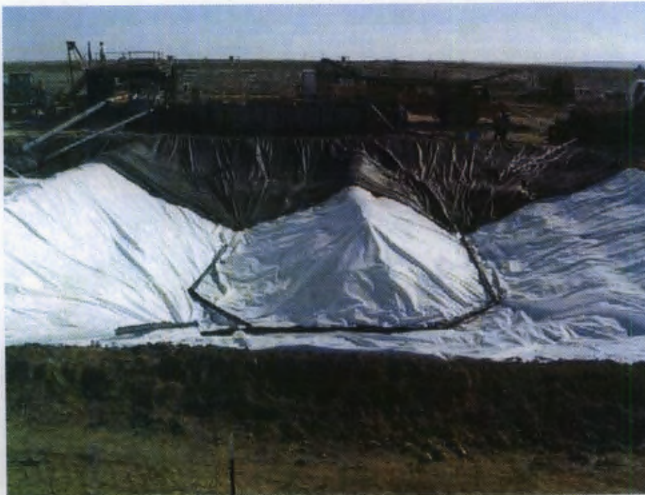
Figure B-5: Cut brine drilling pit chamber with drainage pipes and riser on near side of image. Protective felt (black) on far side of pit.
