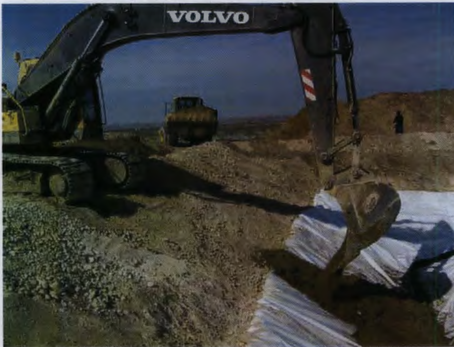
Figure B-2: Placement of permeable layer over secondary liner
