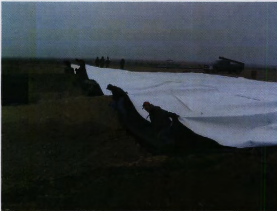
Figure B-4: installation of primary liner over cut brine and fresh water pit chambers.
