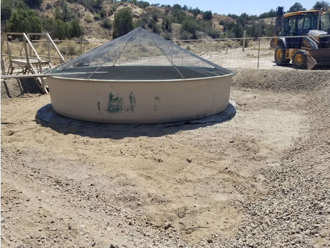
AFTER - TANK WAS RESET ABOVE GRADE
