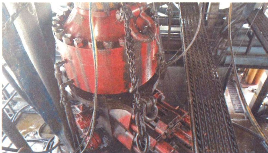
Figure 1: Winch System attached to BOP Stack
