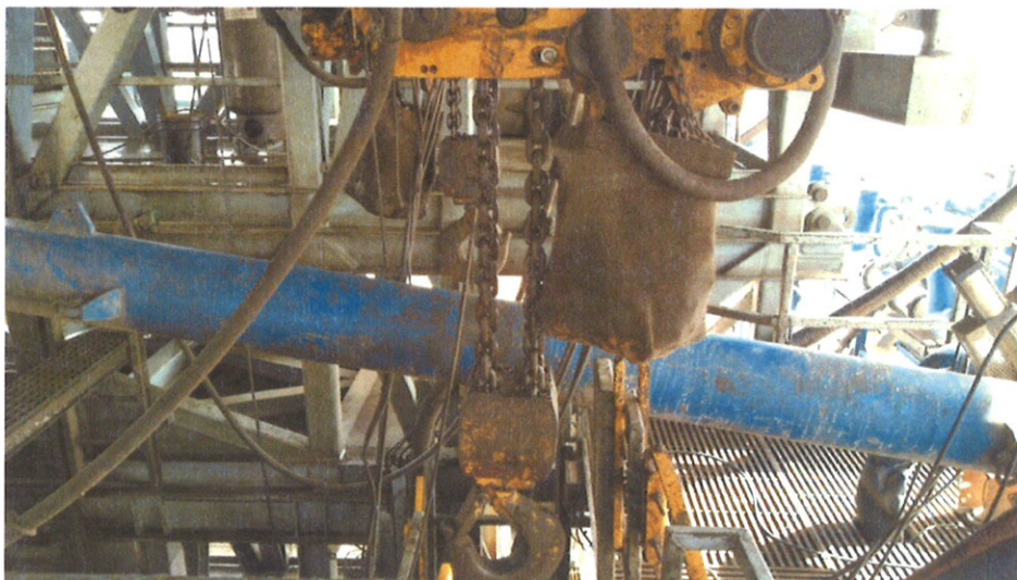
Figure 2: BOP Winch System
