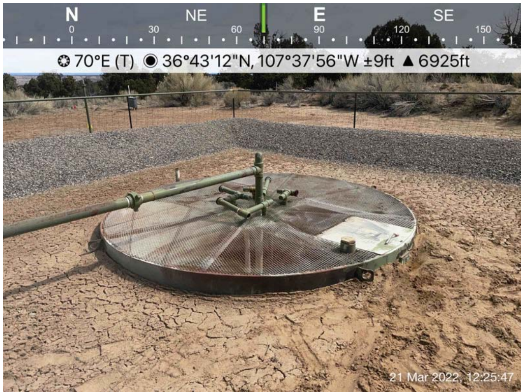
Photo 2: 95 bbls steel tank prior to removal, 3/21/2022.
