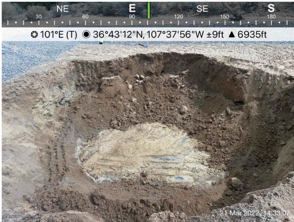
Photo 3: Former location of BGT following removal, 3/21/2022.
