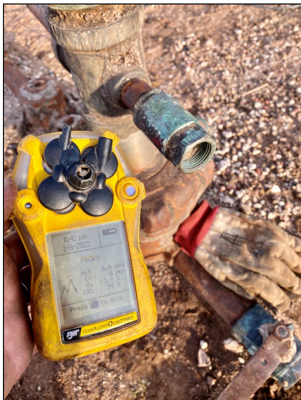
3) DLQ #02Z (30-005-60151) – Wellhead & Field Gas
