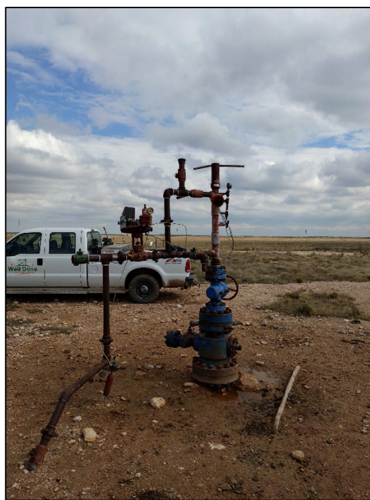
2) Inbe #001 (30-025-37840) – Wellhead - East Facing
