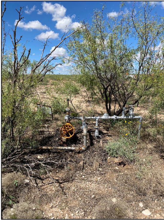
1) Cochise-King Gas Com #002 (30-025-09337) – North Facing
